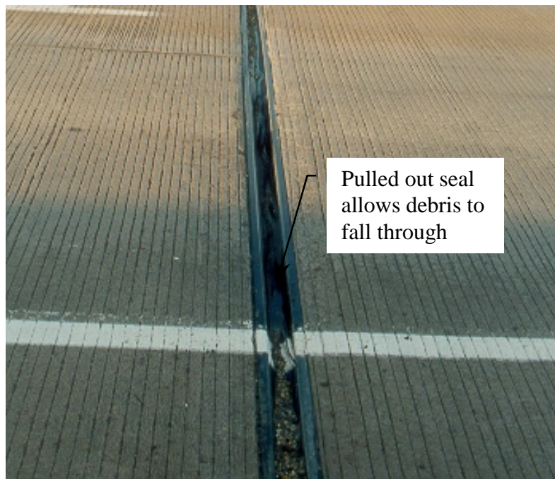
Figure 6.15 Strip seal at G2 for Bridge 4 (0996.0L218)
