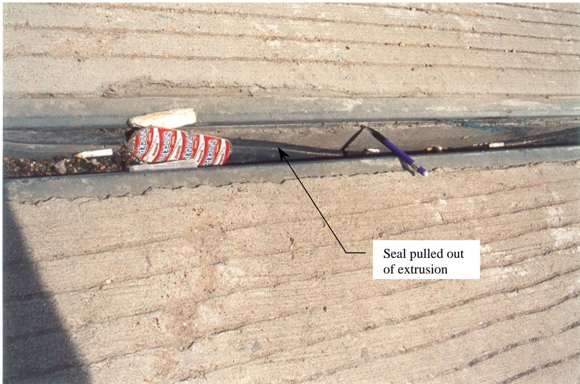
Figure 6.7 Strip seal at G2 for Bridge 2 (0781.1L218)
