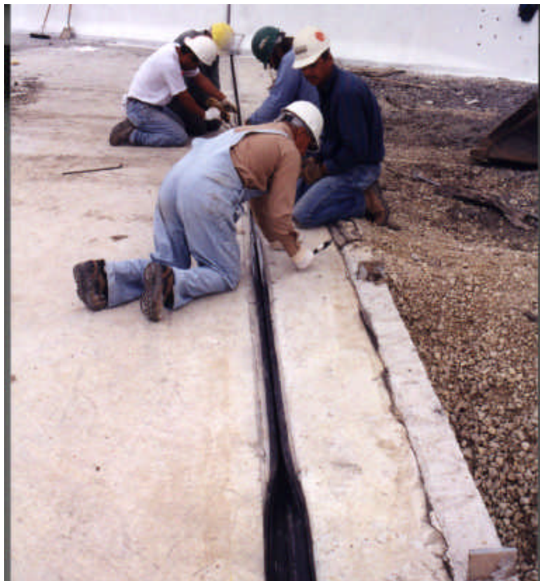
Figure 4.16 Seal is installed in one piece from end to end
