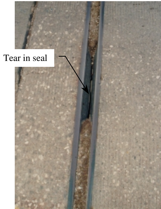
Figure 6.36 Strip seal at G1 for Bridge 10 (6402.0S014)
