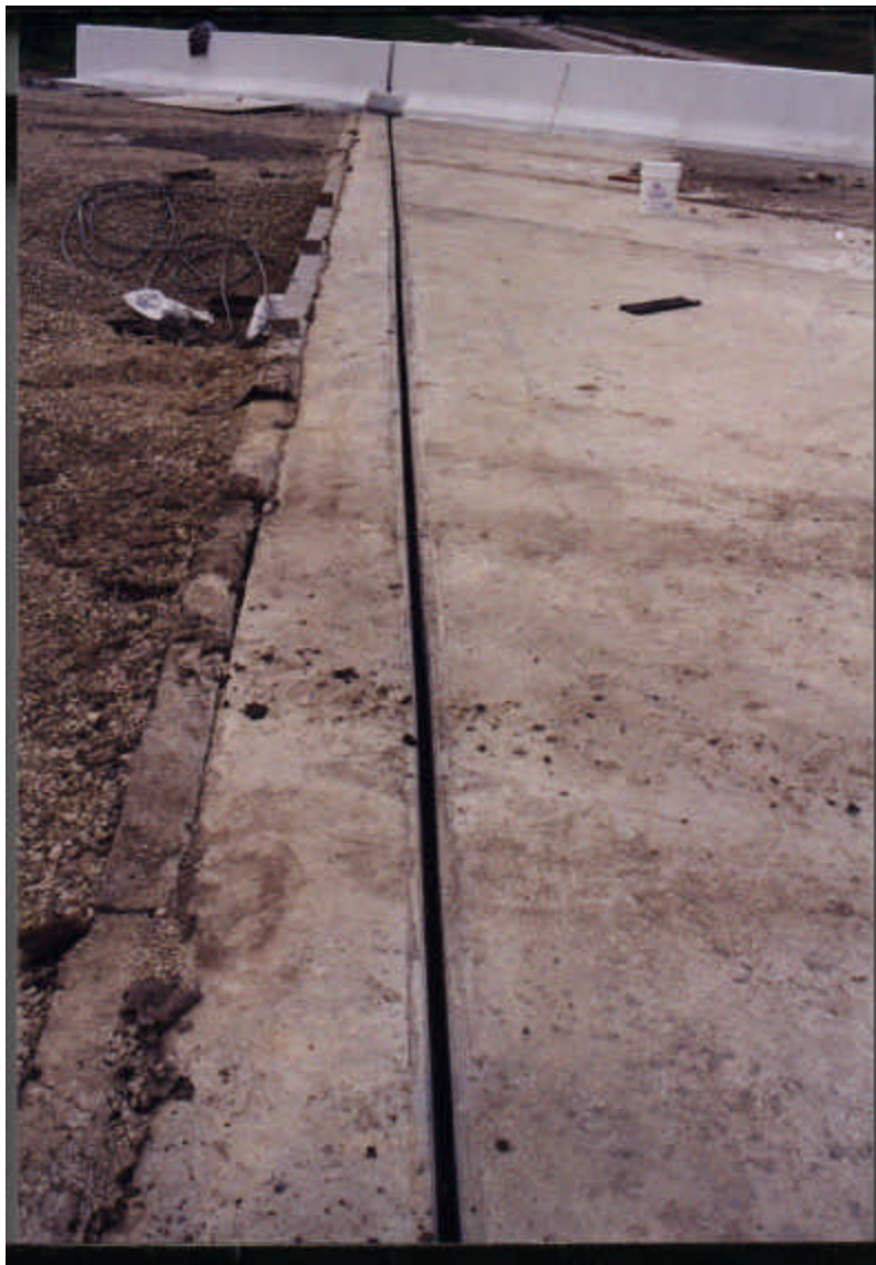
Figure 4.19 Installation of seal complete at east end
