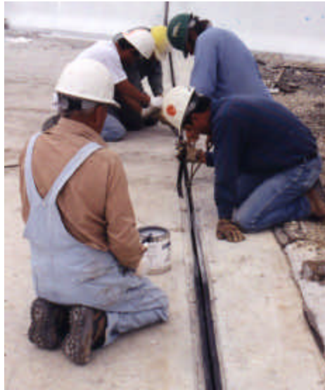
Figure 4.18 Installation requires working in small increments
