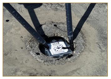
Magnetometer installation: Filling core void with epoxy.
