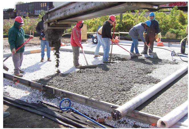
Figure 3.7 Pervious concrete being placed (photo courtesy of John Kevern, University of Missouri-Kansas City)
