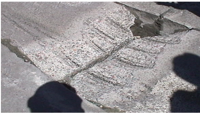
Figure 7.4 Damaged material has been milled out in a partial-depth repair (photo courtesy of Dale Harrington, Snyder and Associates)
