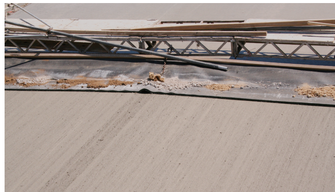
Figure 5.10 Artificial turf drag texture (photo courtesy of Gary Fick, Trinity Construction Management, Inc.)
