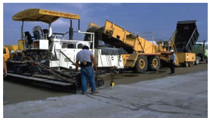
Figure 5.14 RCC placement (Harrington et al. 2010)
