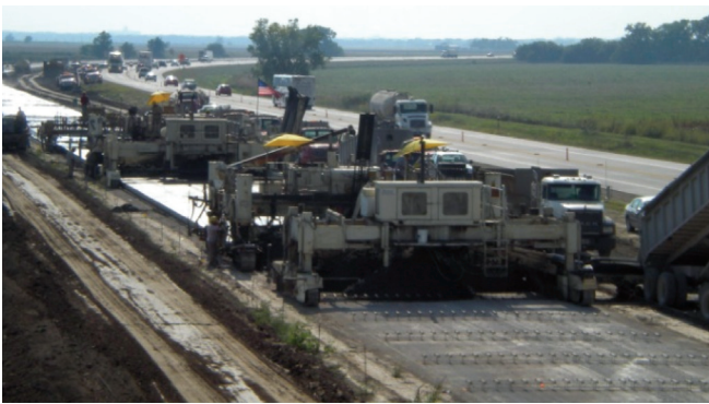
Figure 5.13 Two-lift paving on I-70 in Kansas (photo courtesy of Gary Fick, Trinity Construction Management, Inc.)
