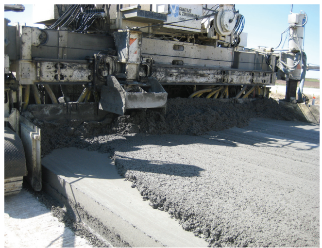
Figure 3.2 Two-lift pavement being constructed in Kansas
