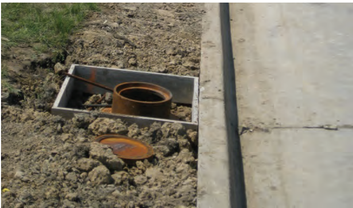
Figure 33. Subdrain retrofit operation including clean out (The Transtec Group)
