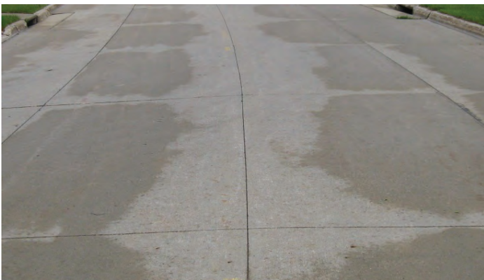
Figure 34. Example of effective drainage of unsealed joints
