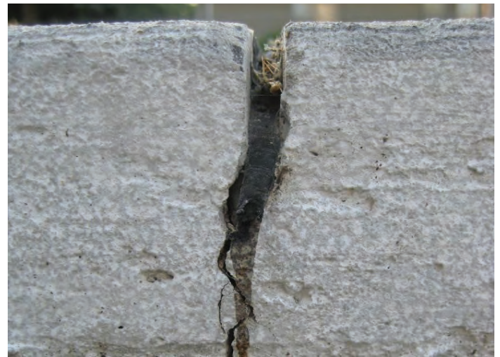
Figure 30. Joint filled with hot pour sealant (Source: The Transtec Group)
