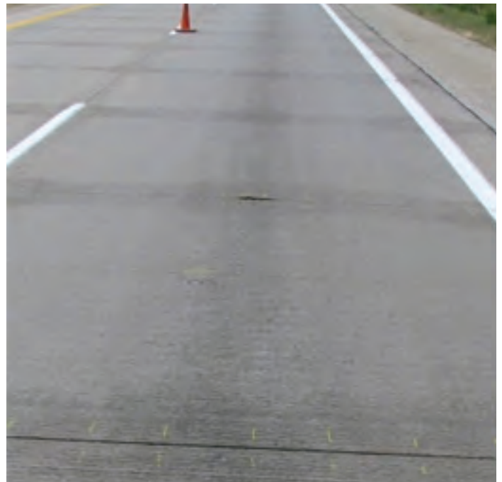
Figure 17. Shadowing at the joints, which is commonly followed by loss of material
