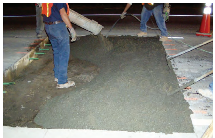
Figure 40. Full-depth patching
