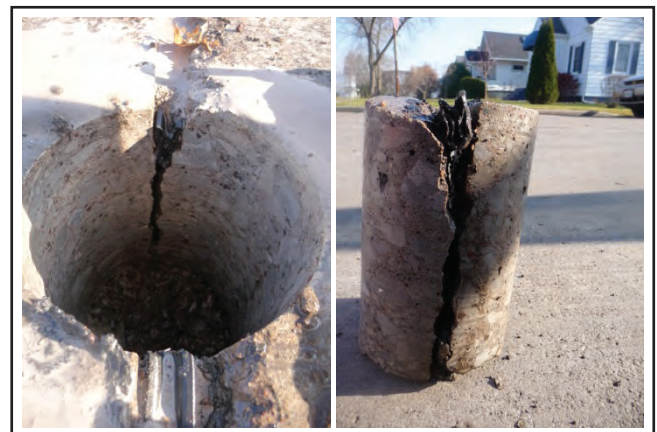
Figure 24. Coring at deteriorated joints to help identify causes of failure
