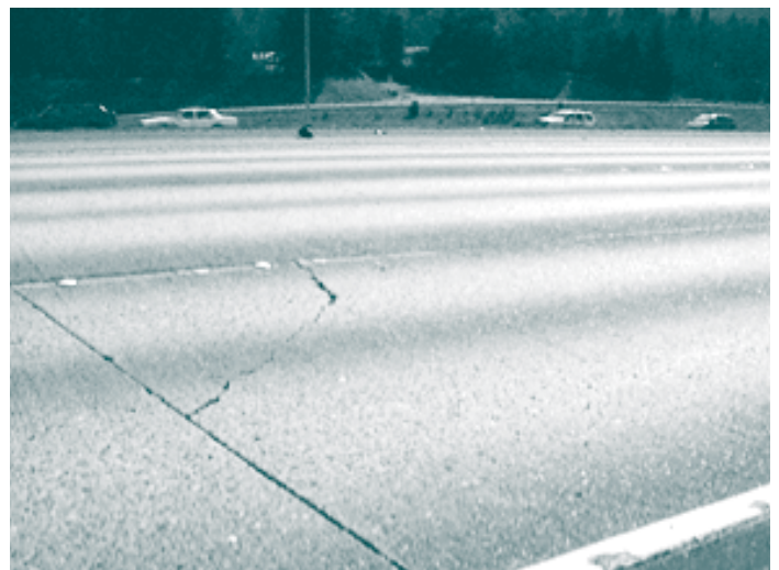
Figure A2. Joint faulting (left, source: Louisiana DOT) and corner breaks (right, source: www.pavementinteractive.com )
