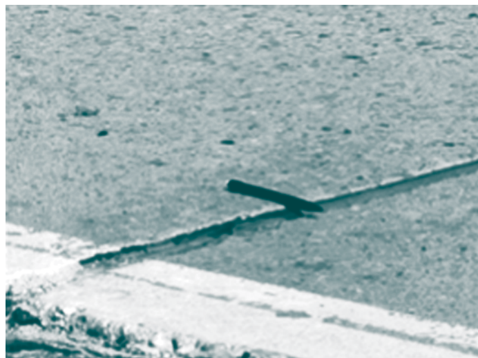
Figure A2. Joint faulting (left, source: Louisiana DOT) and corner breaks (right, source: www.pavementinteractive.com )
