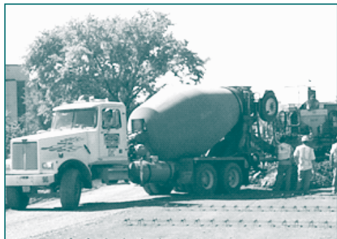
Figure 1b. Dowel baskets positioned ahead of paver
