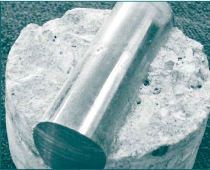
Figure 13. MMFX 2 (microcomposite steel) dowel after five years of service (source: Wisconsin DOT)
