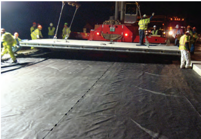
Figure 4-2. Nighttime placement of precast panels in Virginia
