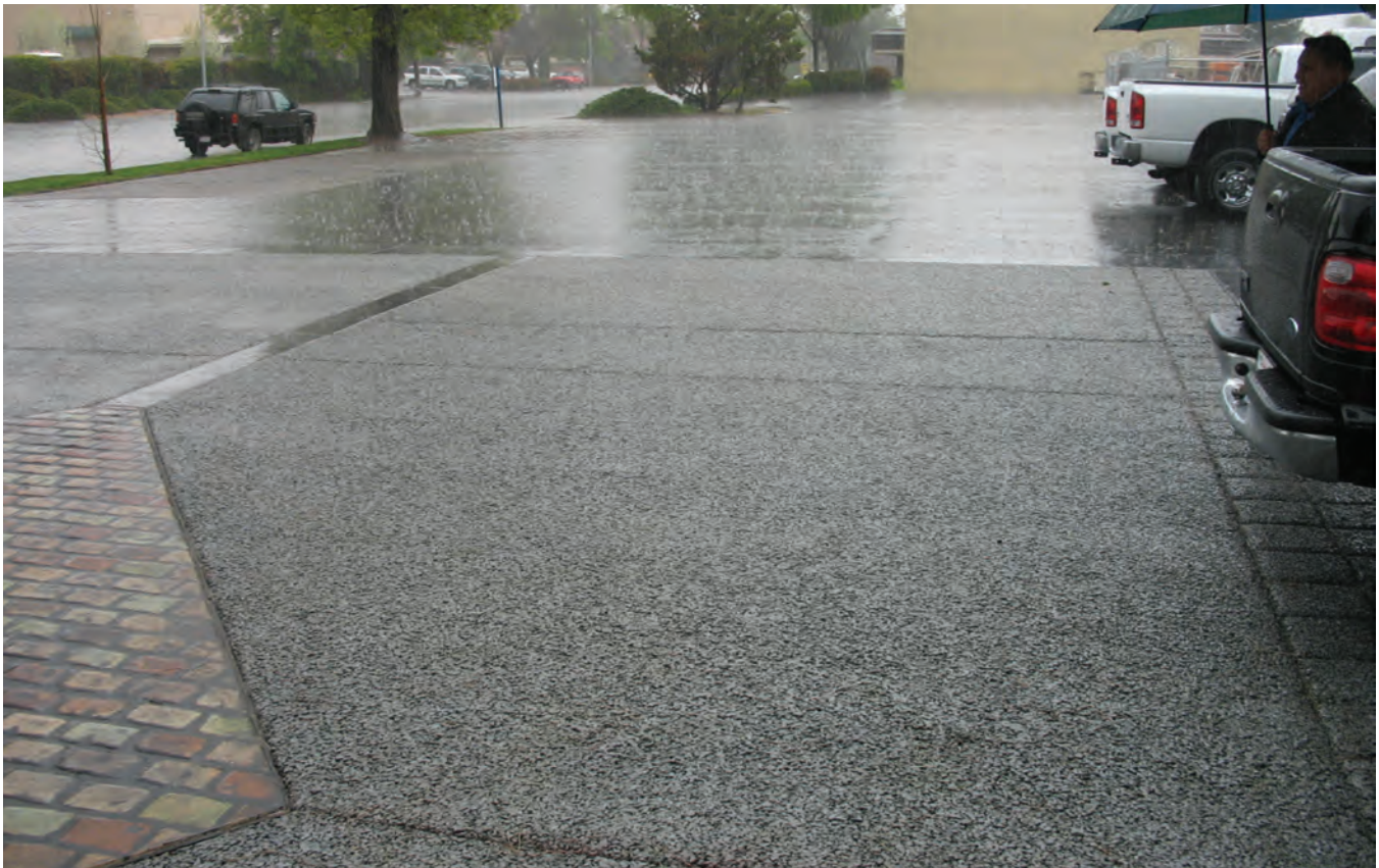
Figure 3-7. Pervious concrete pavement in the rain
