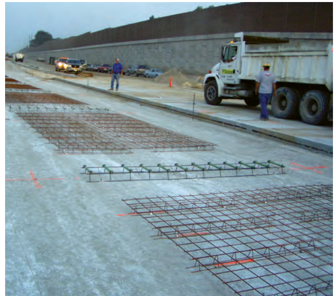
Figure 1-7. JRCP reinforcement in place before paving
