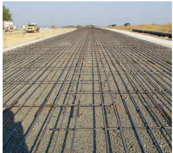
Figure 1-8. CRCP reinforcement placed before paving
