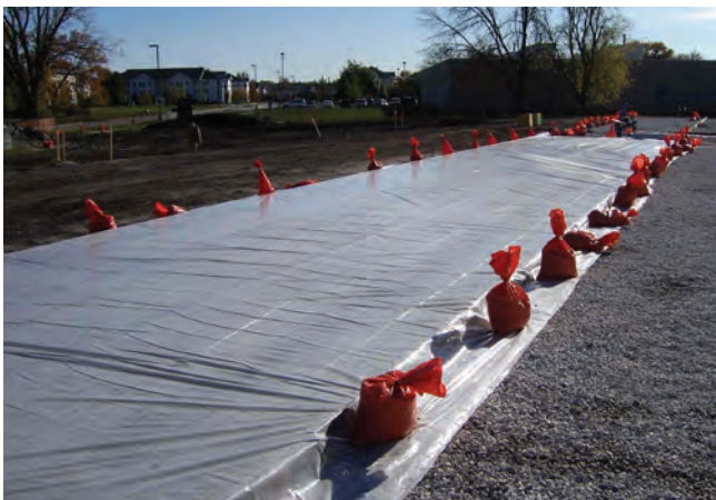
Figure 3-12. Curing pervious concrete with plastic sheeting
