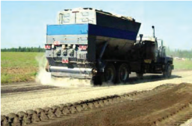
Figure 7-3. Dry cement placed on pulverized material
