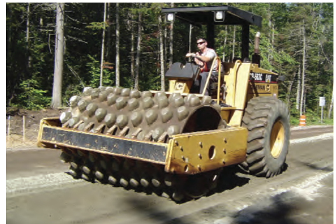
Figure 8-4. Sheepsfoot roller used for compaction
