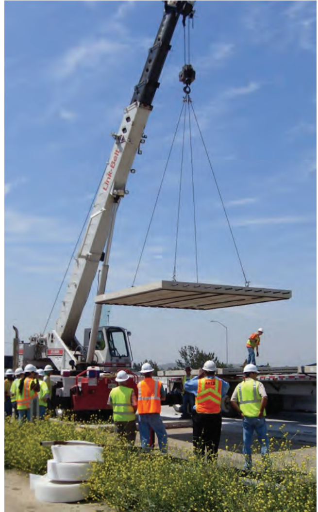
Figure 4-6. Placement of precast panel for precast JCP system
