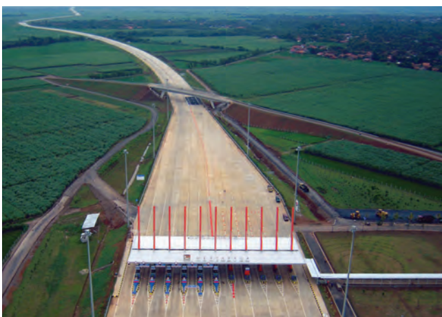
Figure 4-3. Precast pavement system in Indonesia
