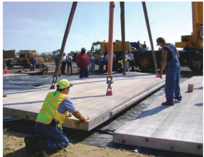
Figure 4-7. Placement of a prestressed precast panel
