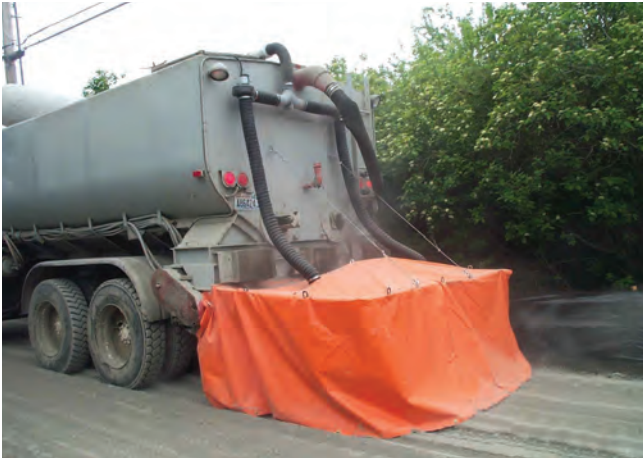
Figure 6-4. Spreading dry cement on grade prior to mixing
