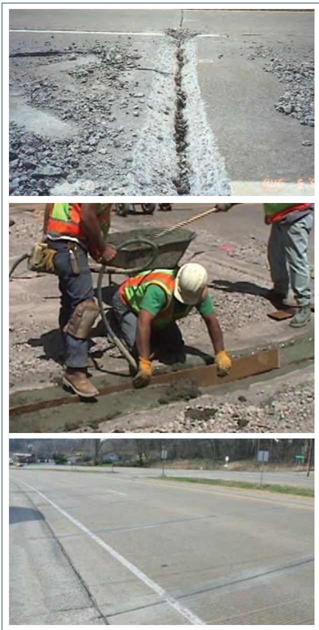
Figure 10-2. Partial-depth repair process at joint
