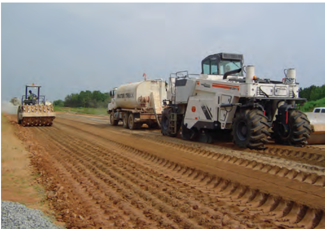
Figure 6-6. Constructing CTB using mixed-in-place method
