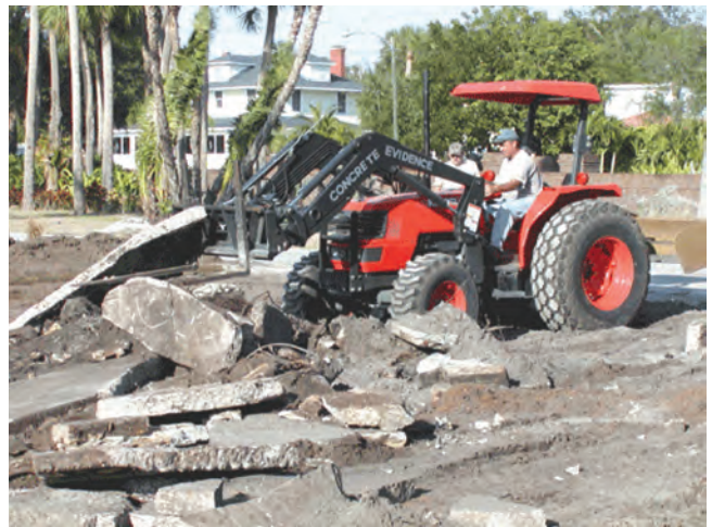
Figure 9-3. Broken concrete pavement is removed for recycling
