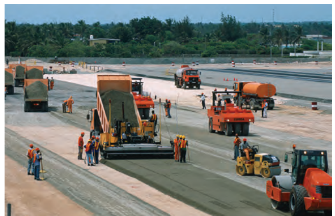
Figure 6-7. Placement of plant-mixed CTB on prepared subgrade
