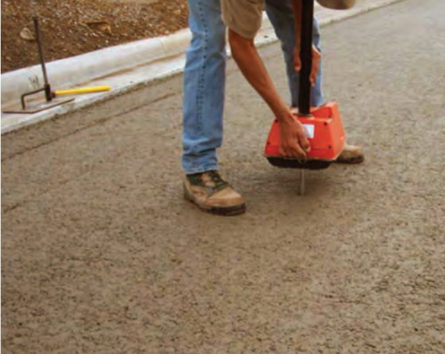
Figure 5-15. RCC in-place density measurement
