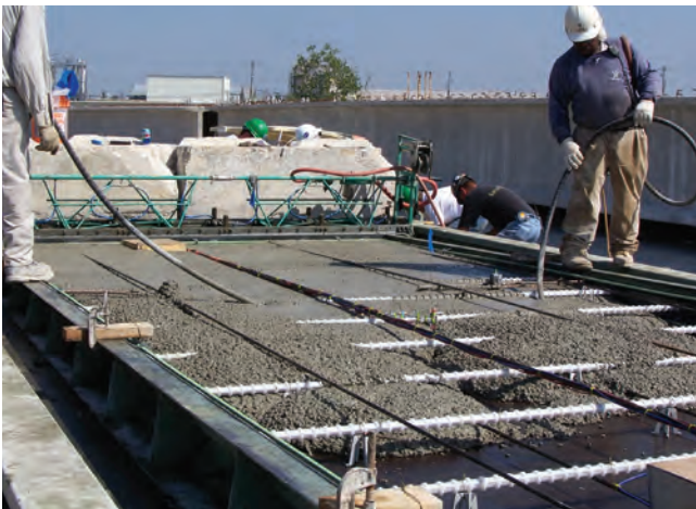
Figure 4-5. Vibrators for consolidation of concrete around reinforcement in precast prestressed panel
