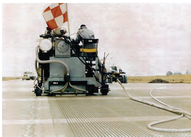
Figure 10-8. Longitudinal grooving of a concrete pavement to restore macrotexture
