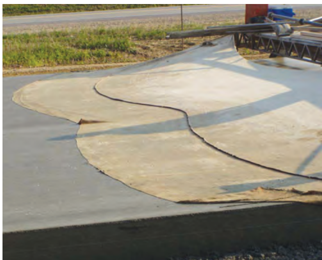
Figure 1-9. Burlap drag on fresh concrete
