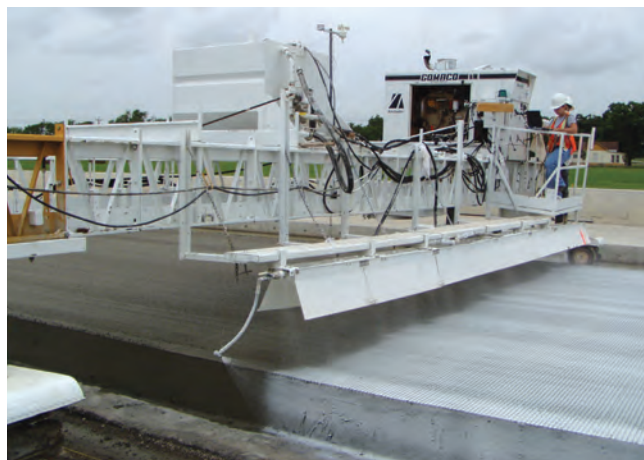
Figure 1-10. Curing compound applied by spray nozzles on a cure cart
