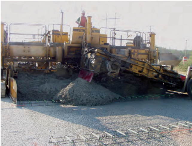
Figure 1-5. Concrete placed over dowel baskets
