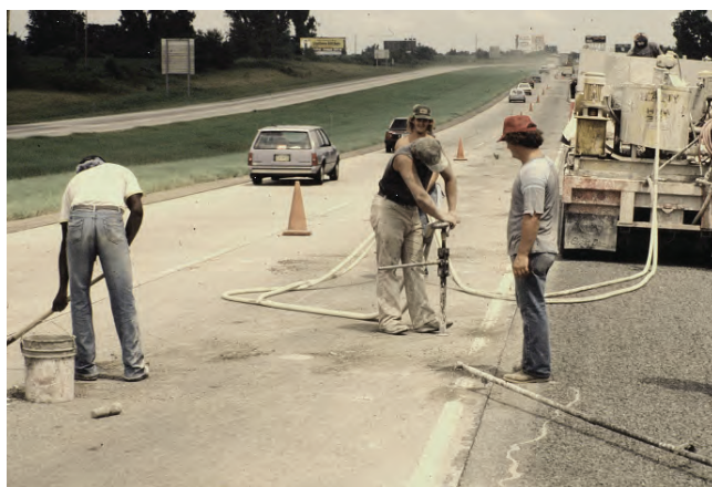
Figure 10-4. Drilling operation as part of slab stabilization
