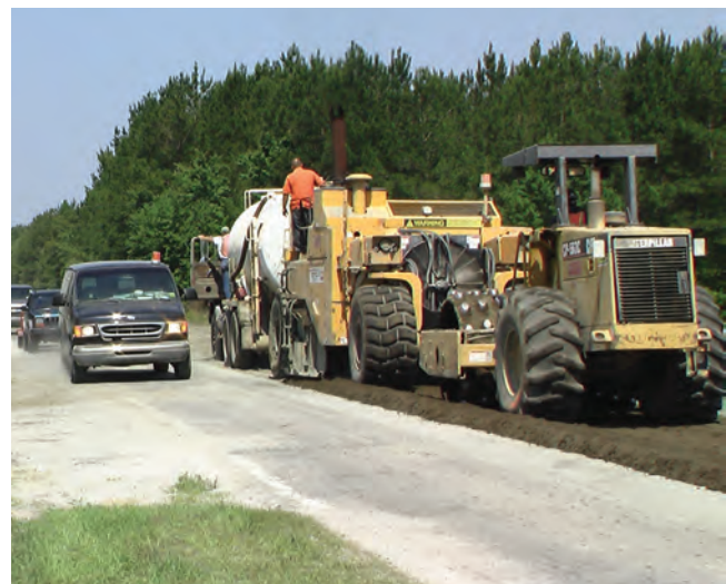
Figure 7-2 Reclaimer pulverizing existing asphalt pavement and base material
