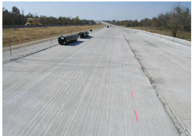
Figure 6-3. Completed CTB for new pavement construction in Oklahoma
