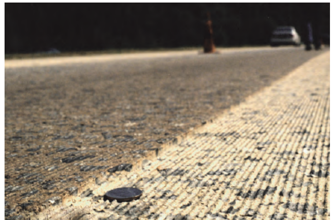
Figure 10-7 Diamond grinding concrete pavement for surface restoration
