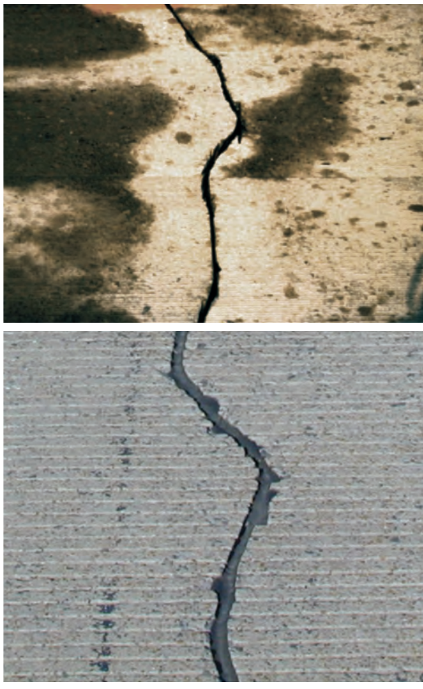
Figure 10-5. Application of joint sealant
