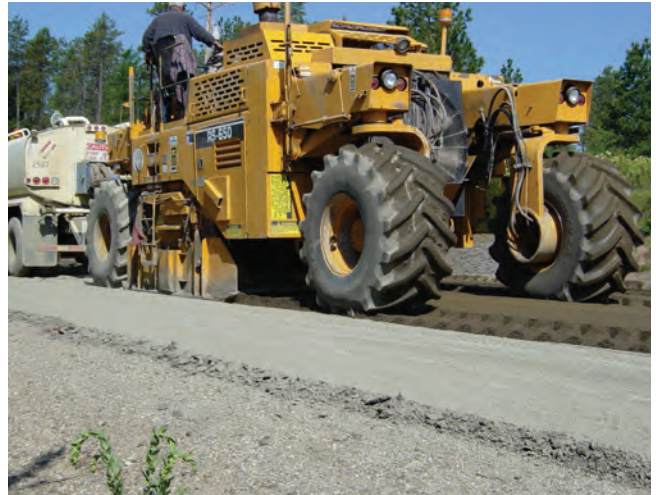
Figure 7-5. Mixing the cement into the pulverized material
