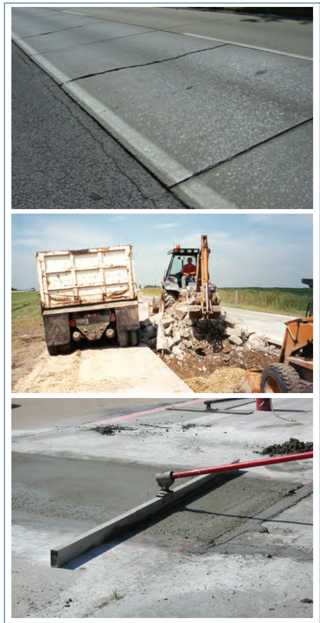
Figure 10-1. Full-depth repair of a concrete pavement slab
