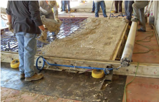
Figure 4-4. Concrete poured into form for precast panel
