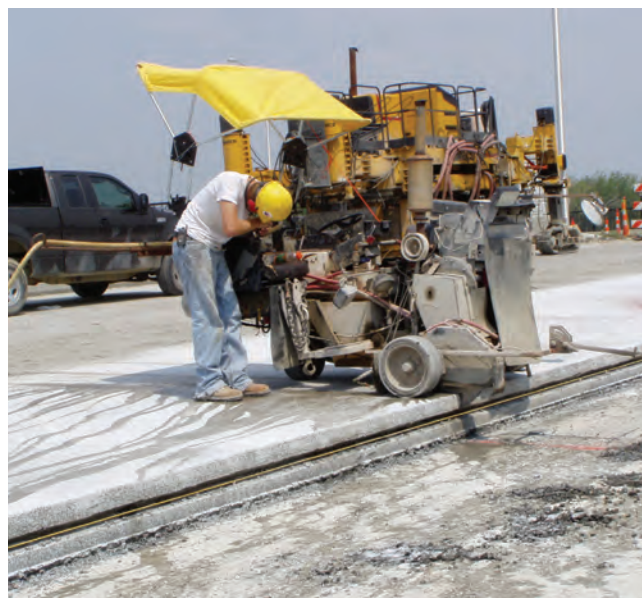
Figure 1-4. Sawcutting JPCP
