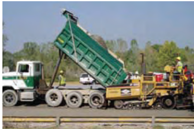
Figure 5-9. RCC delivered to jobsite
