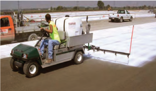
Figure 5-16. Curing RCC
