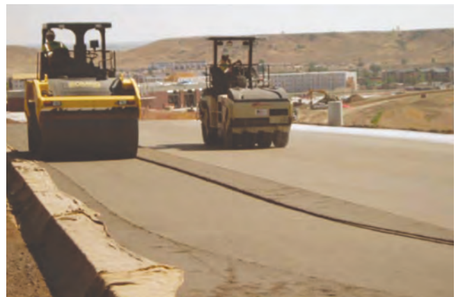
Figure 5-14. Compacting RCC using both vibratory and pneumatic-tired rollers
