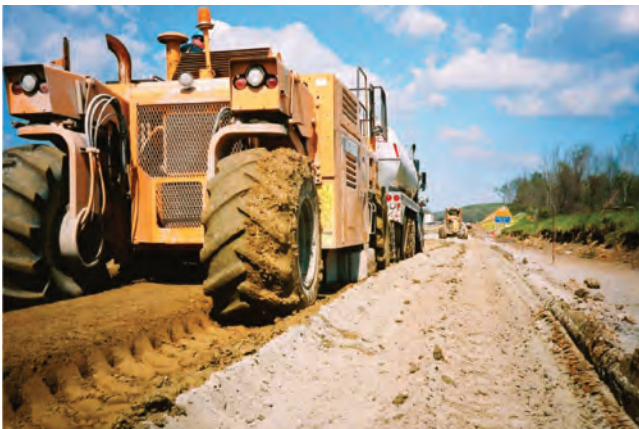
Figure 8-3. Pulverizer used for in-place mixing of CMS
