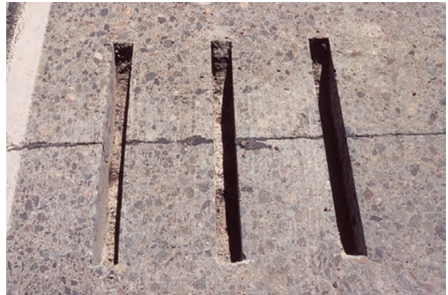
Figure 10-6. Contiguous concrete slabs prepared for dowel bar retrofitting
