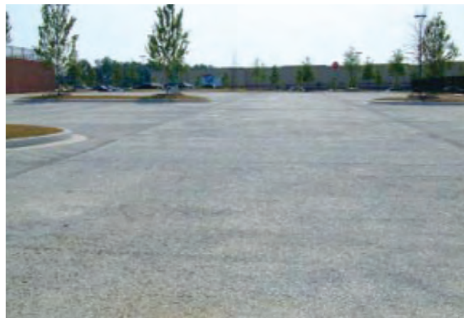
Figure 3-5. Pervious concrete pavement parking lot
