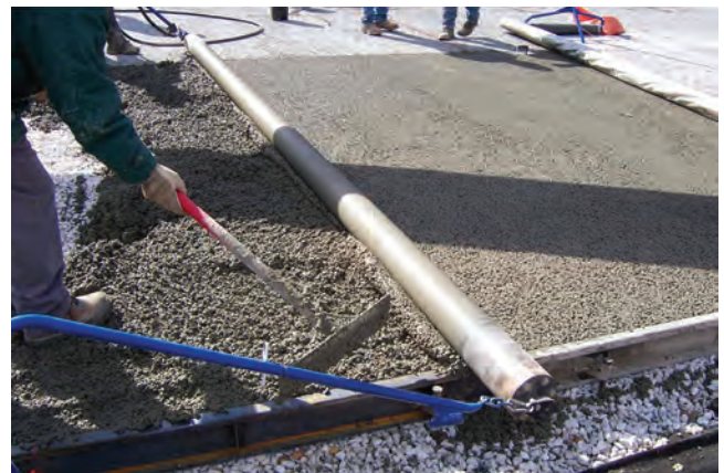
Figure 3-11. Compacting the placed pervious concrete
