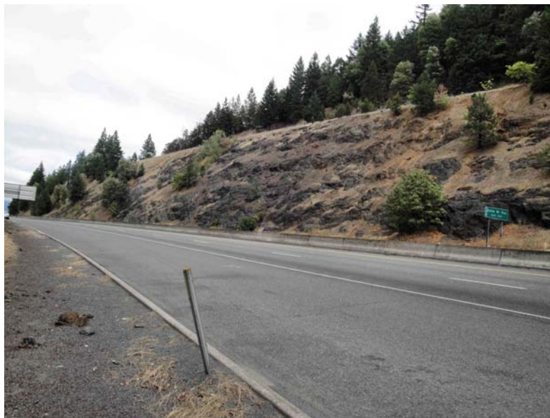
Figure 4.22: View of the Sexton Summit from I-5's northbound lane. In the highwall of the roadcut, the rocks are metavolcanic and metasedimentary rock.
