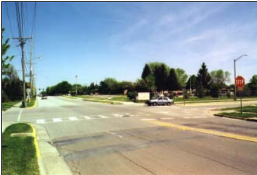
Figure 6.5. Marked Crosswalk
