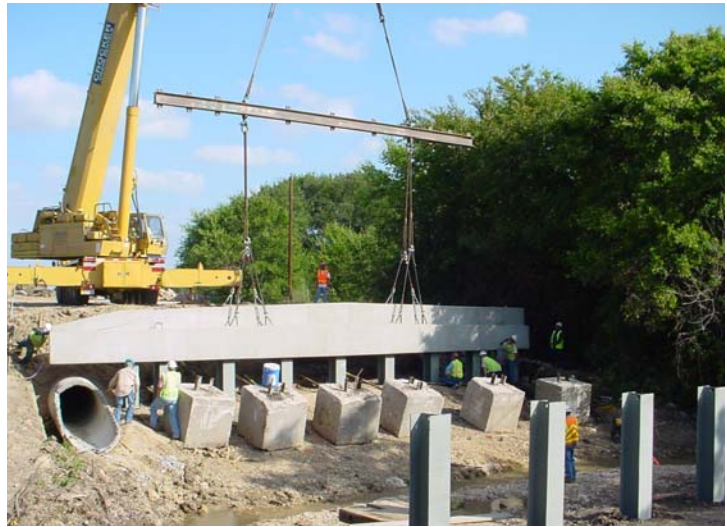
Figure CS3-4 Abutment Bent Installation
