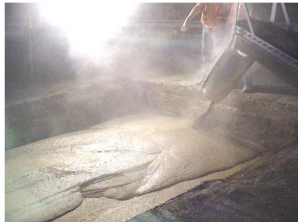
Figure CS3-10 Placement of Flowable Fill
