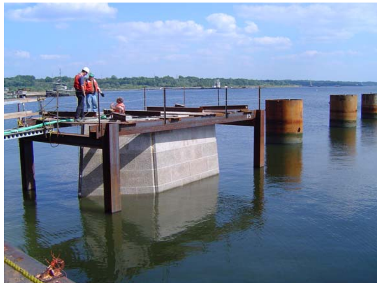
Figure 4.1.7-1 Providence River Bridge Pier Box
