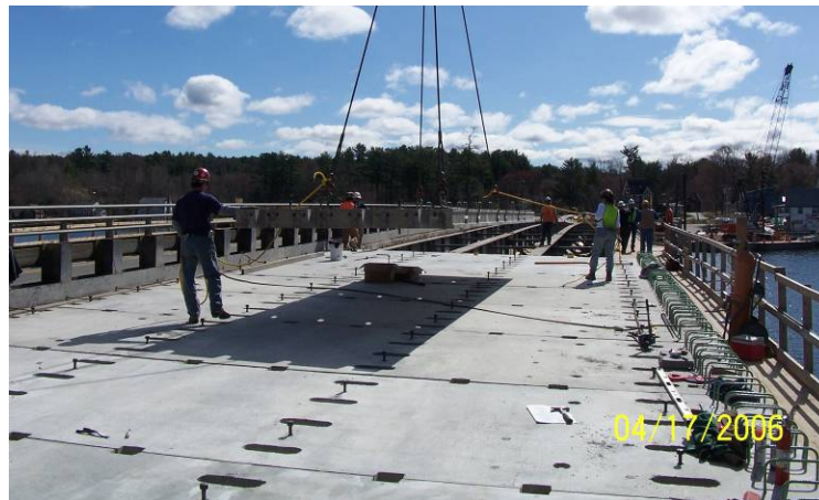
Figure 1.2.4-1 Full Depth Precast Deck Panels
