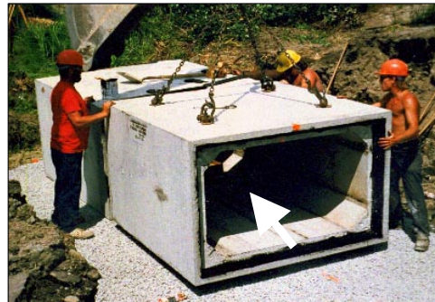
Image Courtesy American Concrete Industries, 2007
