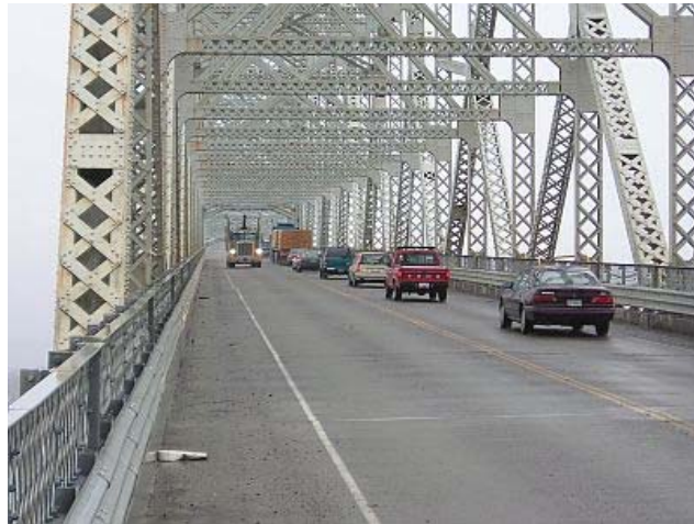
Figure 2.4.2-2 Lewis and Clark Bridge (Courtesy of Washington DOT)
