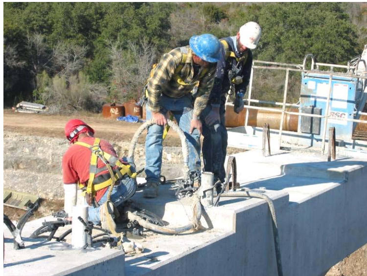
Figure CS2-6 Grouted Placement
