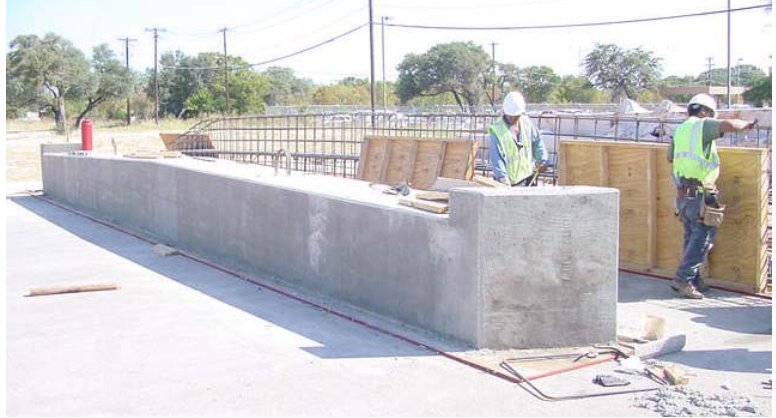
Figure CS3-2 Pile Bent Cap Fabrication
