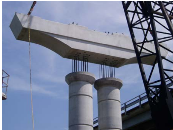
Figure EX2-1 Lake Belton Bridge Pier
