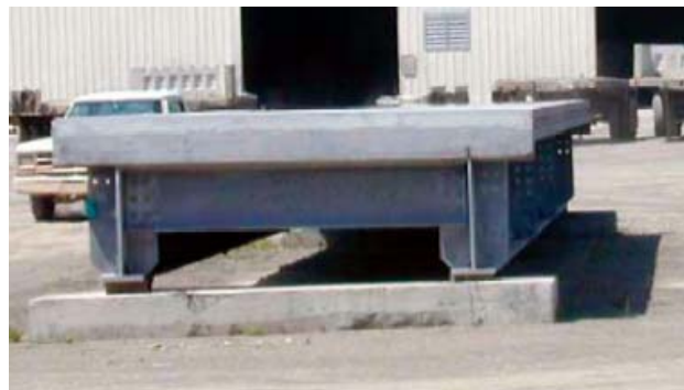
Figure 2.4.1-1 Inverset Deck System Details
