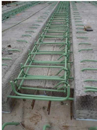
Figure 2.2.3.1-1 Minnesota Adjacent Beam System
