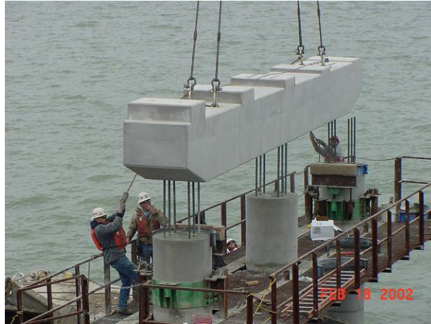
Figure 1.2.4.-2 Precast Pier Cap
