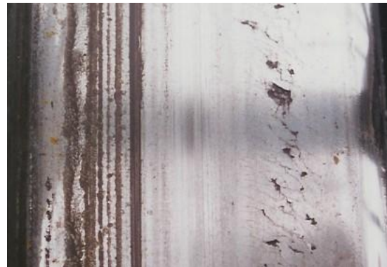
D) Deeper cracks on the field/rim side of the wheel tread with material starting to shell out.
