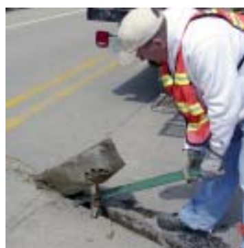
1. Removing the old foam
