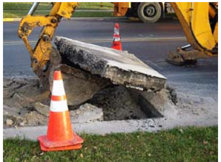
Pavement removal
