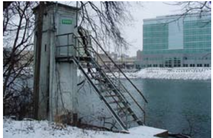
A typical USGS streamflow-gauge with satellite telemetry
