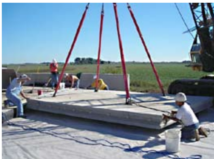
Figure 9 - Precast approach slab unit prior to placement in O'Brien County
