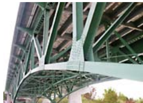
Figure 8 - A truss bridge on Hwy 926 in Fort Dodge that was load tested to validate load-rating results.
