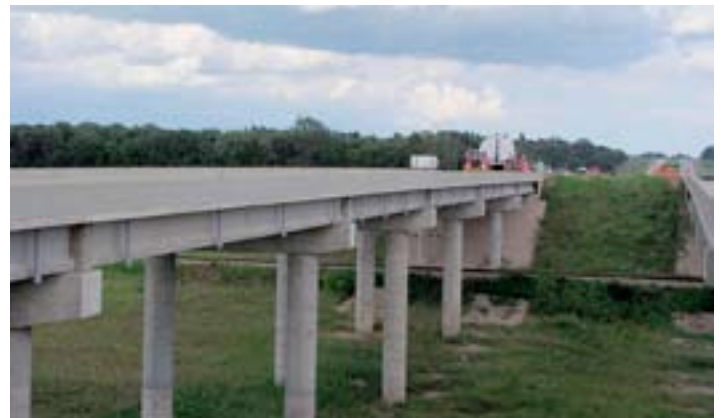
Figure 35 - Partial elevated view of the five-span, prestressed girder bridge
