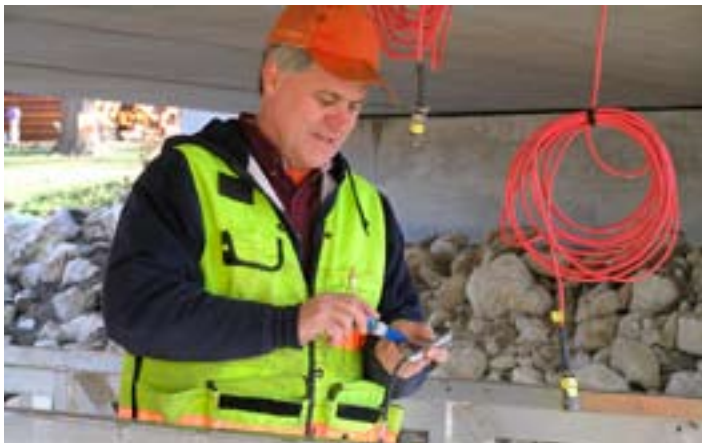
Figure 3 - Quick-setting adhesive applied to "footprints" on sensors allows bonding to a concrete beam in a region previously cleaned by surface grinding.
