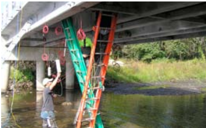
Figure 32 - Strain instrumentation placed on the pi-girder bridge prior to load testing.
