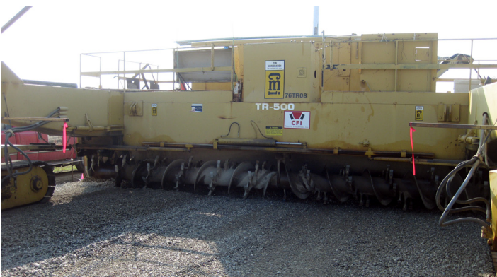
Figure 10 – On-site conditions and construction operations
