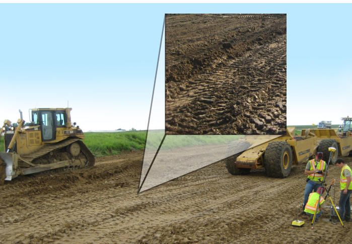
Figure 7 – Soil conditions on site
