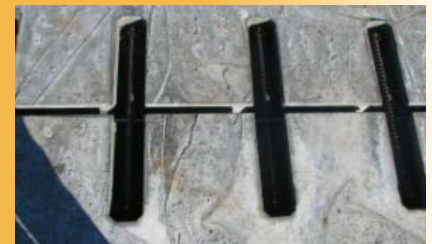
Figure 6 - Jakway Park Bridge
