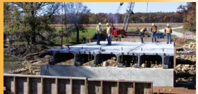
The first of three 51-foot-long pi-shaped girders being placed on Jakway Park Bridge piers
