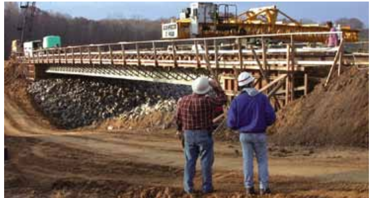
Figure 1 – The first UHPC bridge built in the United States is located in Wapello County, Iowa.
