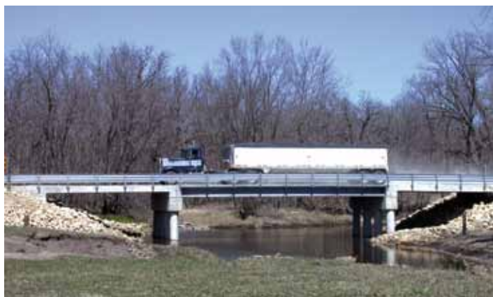
Figure 8 – The completed bridge was open to traffic on November 26, 2008.
