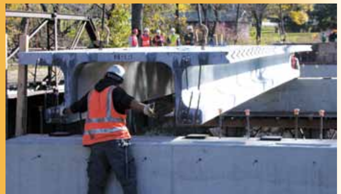
The first of three 51-foot-long pi-shaped girders being placed on Jakway Park Bridge piers
