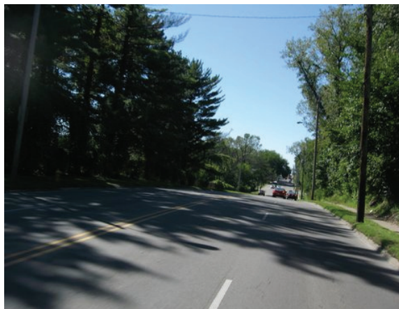
Utility poles along a Des Moines, IA street are within a few feet of the roadway.
