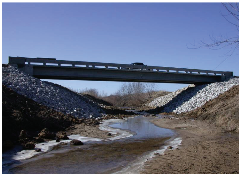
A UHPC prestressed Bridge constructed on Little Soap Road in Wapello County, Iowa
