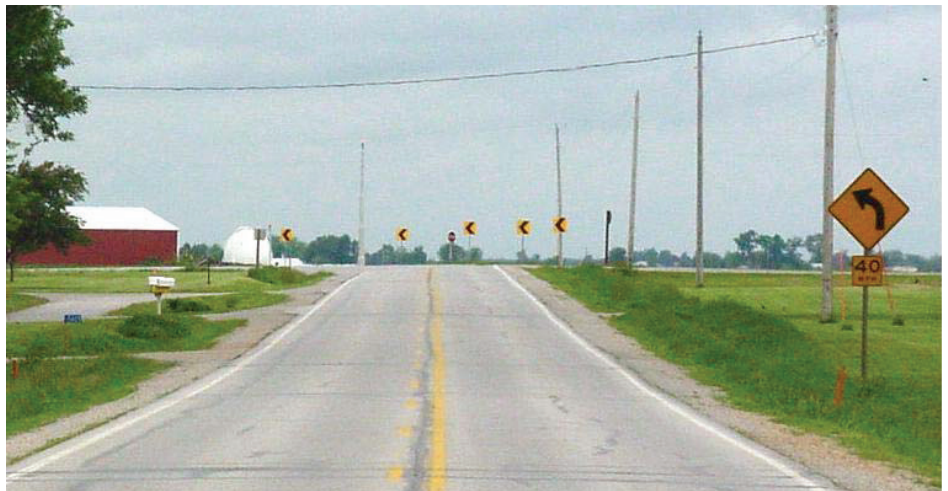
Larger chevrons and curve signs on US 6, Johnson County - Photo: Tom Welch, Iowa DOT Office of Traffic and Safety
