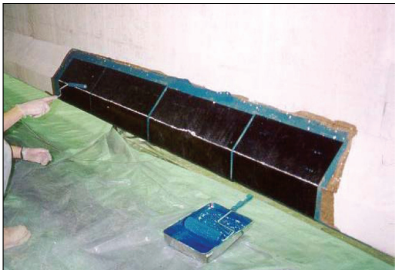
Installation of transverse CFRP jacket on Beam
