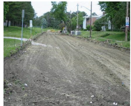
Re-compacted uniform subgrade prior to placement of new pavement
