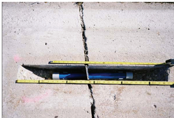
Proper Slot Length
