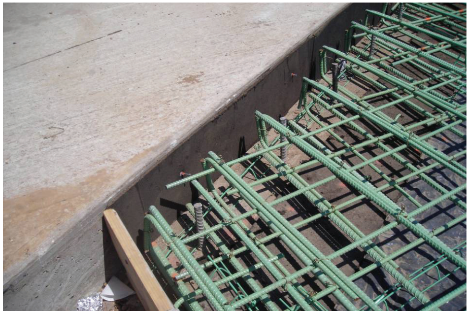
Installation of an improved bridge-to-pavement connection detail
