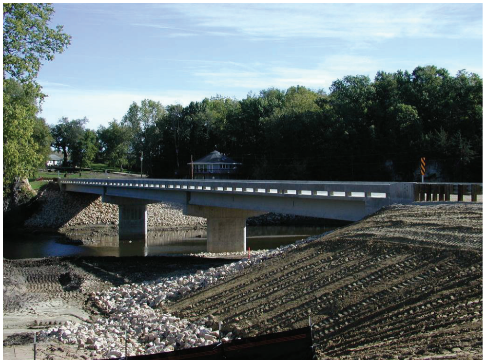
A three-span prestressed concrete bridge constructed in Jones County
