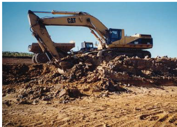
Soil mixing operation through layered soils, Des Moines, Iowa
