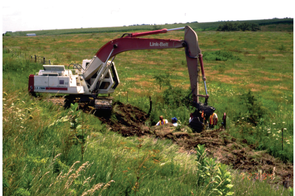
Crew excavating Mahaska County site for placement of culvert
