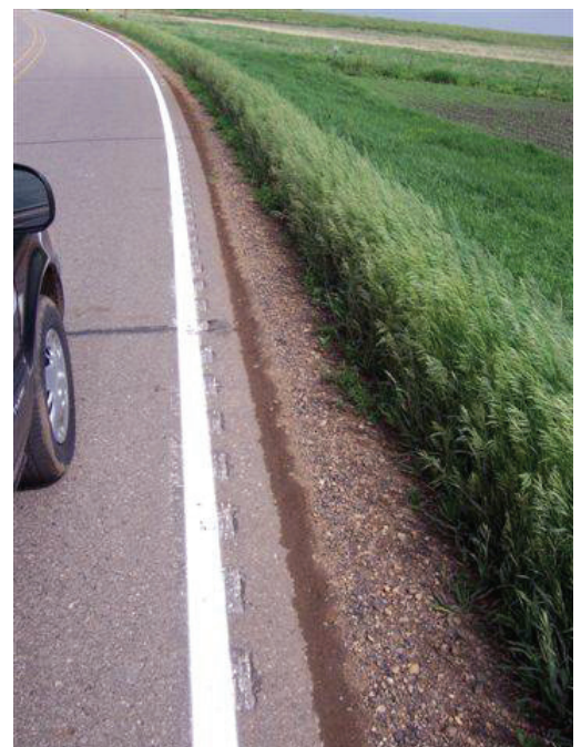
A test section of rumble stripes and reflective paint completed in June 2008
