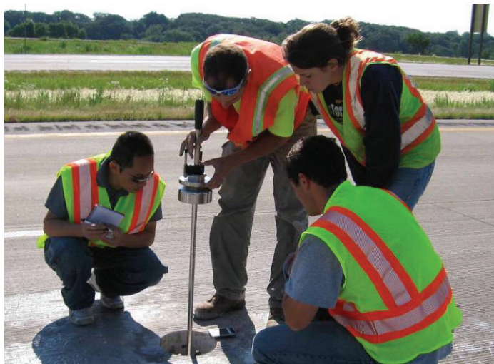
Lightweight deflectometer (LWD) test
