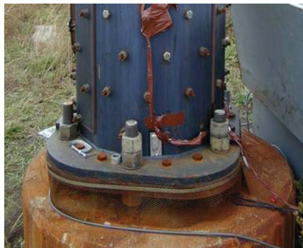
Bolted Reinforcing Jacket
