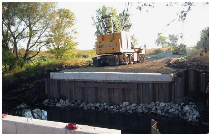
Modified sheet pile abutments
