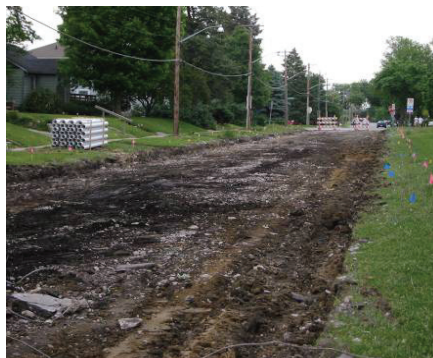
Existing non-uniform subgrade after pavement removal
