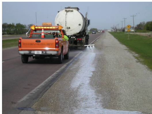
S.S. polymer topically applied to the granular shoulder
