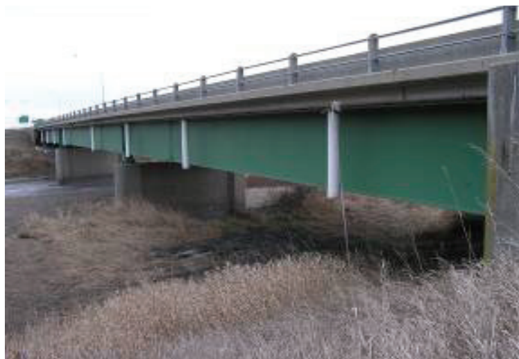
Side view of the US 30 steel bridge
