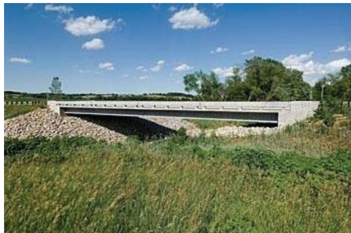
A view of completed Mars Hill Bridge – Photo: ISU Bridge Engineering Center 2007
