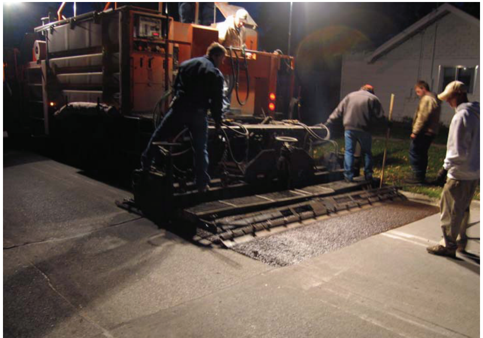
Application of the night test section in West Des Moines, Iowa
