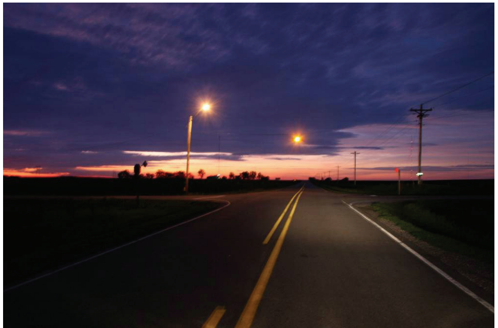
Nighttime lighting at N.W. 142 nd at R38 (Polk County) at dawn – Photo: Neal Hawkins, Iowa State University/CTRE
