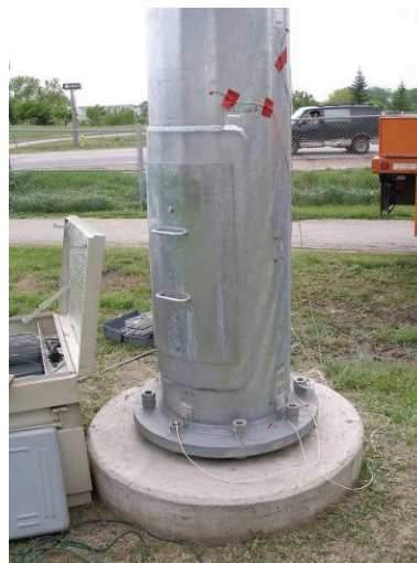
Replacement tower base
