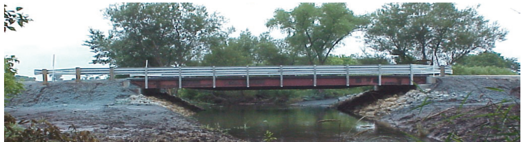
The finished Buchanan County RRFC Bridge
