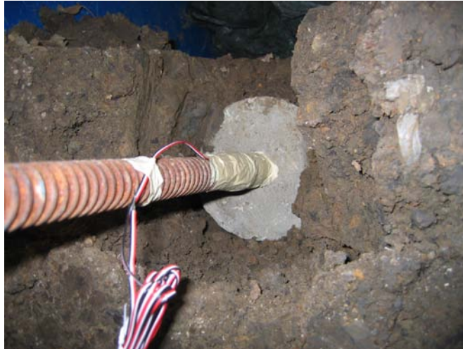
FIGURE 4.13 Strain gage connected to the soil nail
