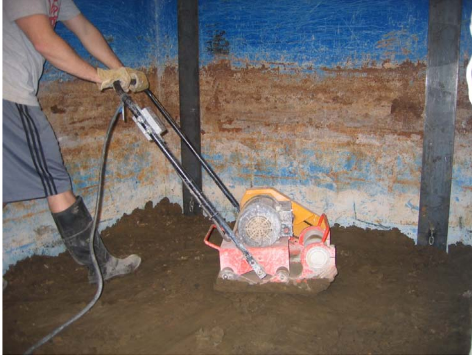
FIGURE 5.1a Compaction
