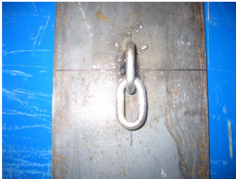
FIGURE 4.7a Chain link on the anchor plates
