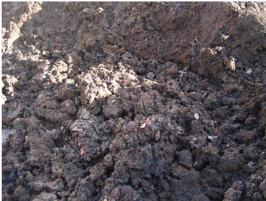
FIGURE 4.2 Soil used as fill material for the soil nailed wall
