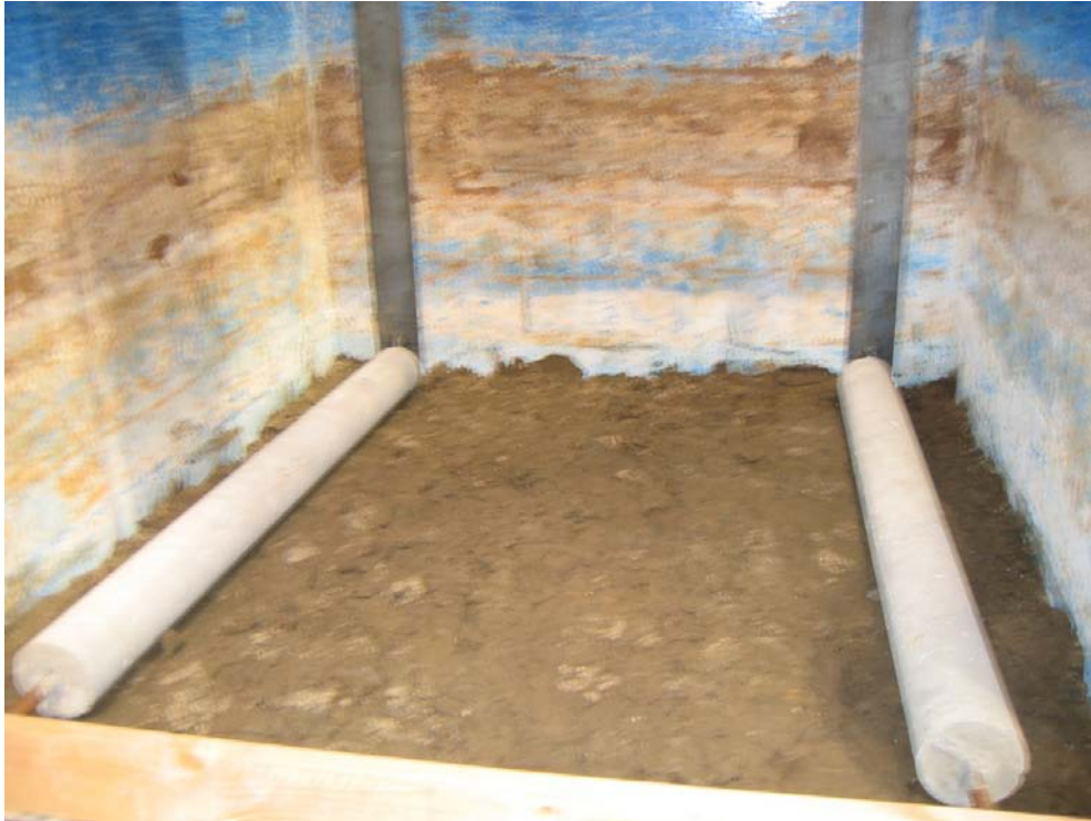
FIGURE 5.2 Soil nails installed
