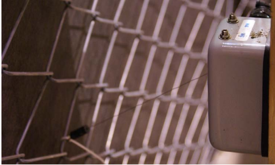
FIGURE 5.14 Downward movement of string pot connection due to settlement
