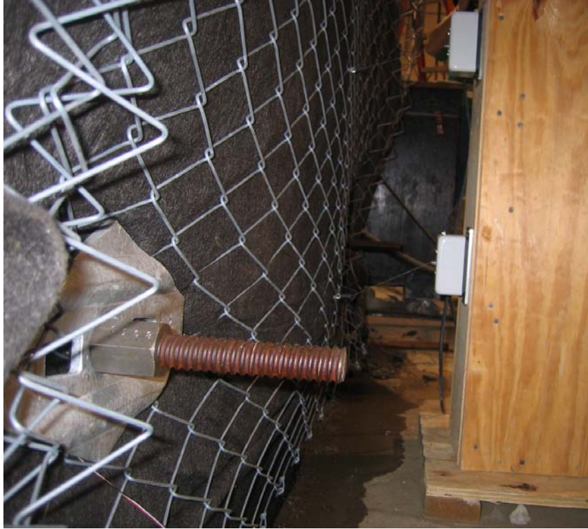
FIGURE 5.9 Soil face after application of 5 psi surcharge
