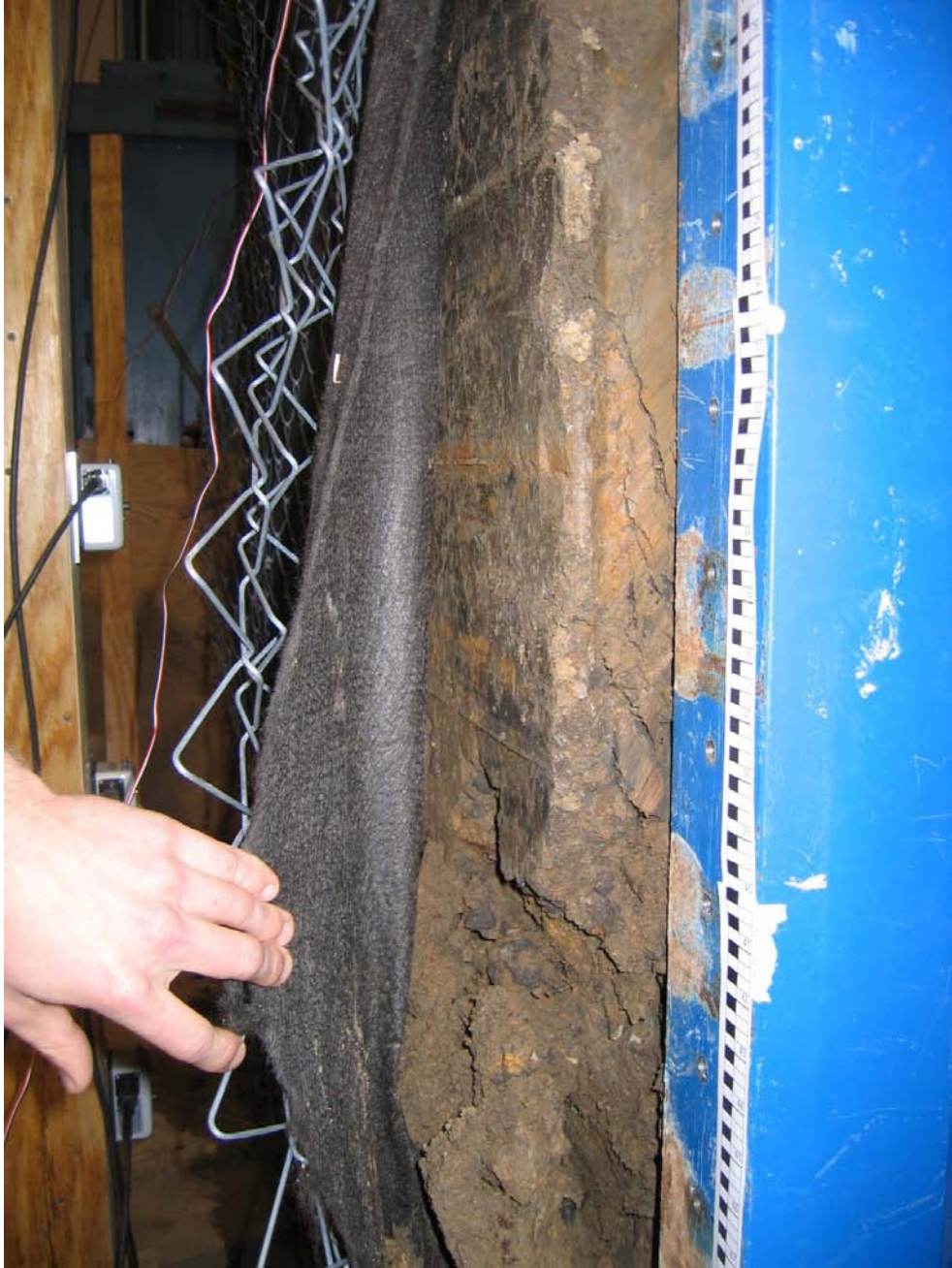
FIGURE 5.8 Right side of soil face after application of 5 psi surcharge
