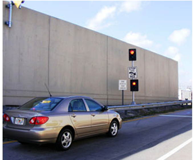
A car waits at a ramp signal before entering I-95 in South Florida. Regulating the rate at which cars enter the interstate can improve overall traffic flow on the highway.
