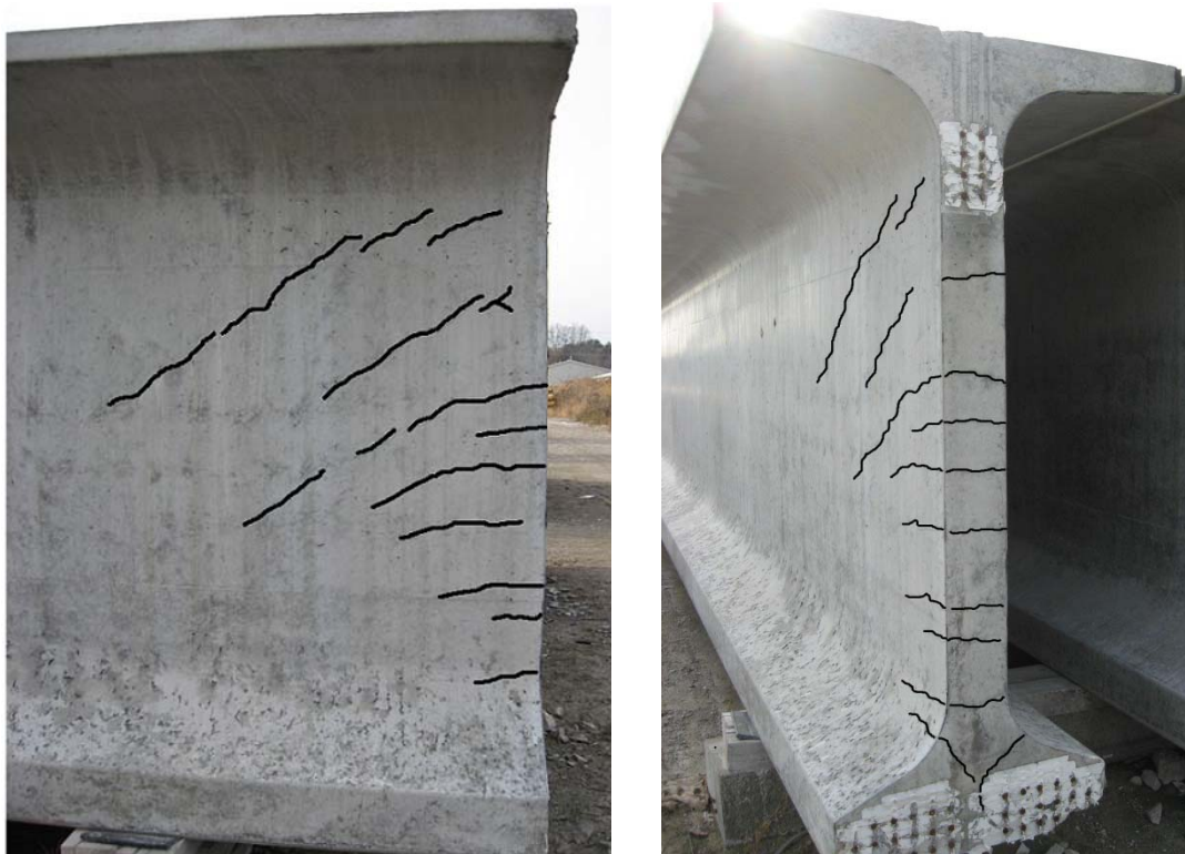
Figure 1 – Typical cracking pattern of the deep wide flanged girders.
