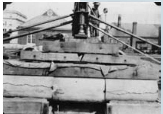
Concrete pipes subjected to stress testing in the early 1920s
