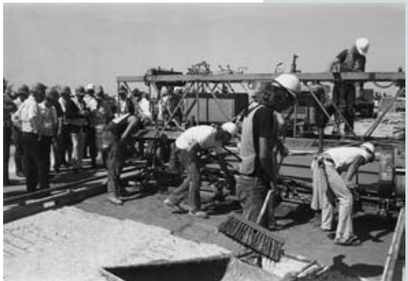
1970s Iowa method of bridge deck repair
