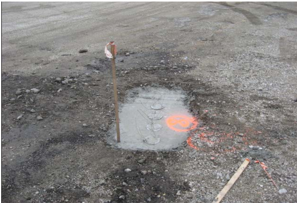
Figure 6.10 View of Block 8 at Test Pile #2 Location
