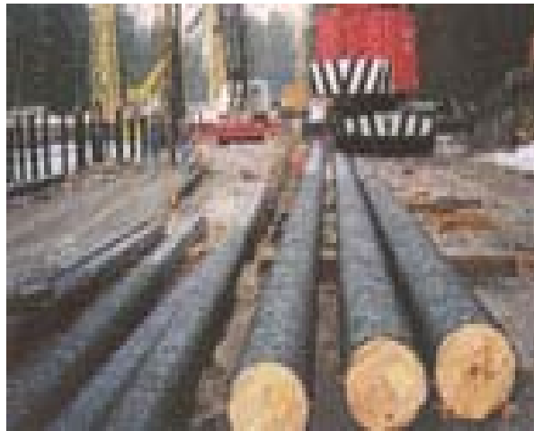
Figure 2.24 Timber piles
