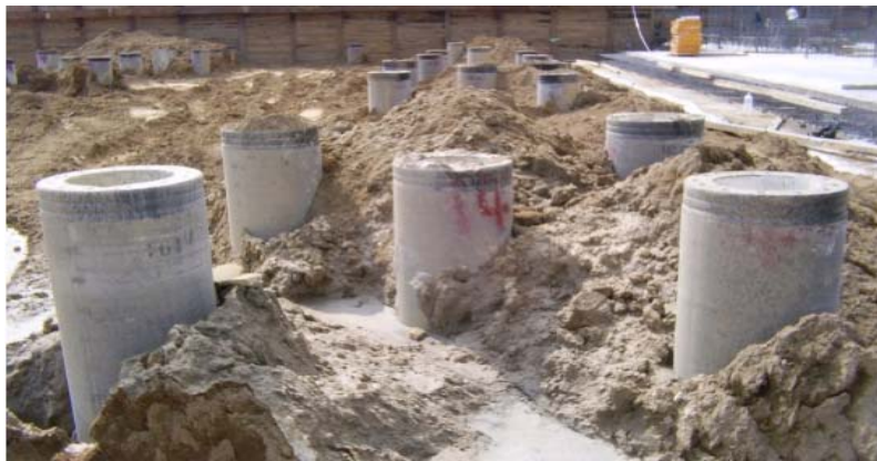
Figure 2.21 Precast concrete piles
