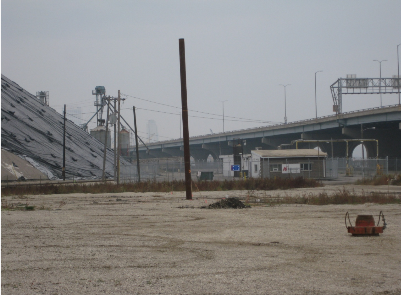
Figure 6.8 – View of Test Pile # 1 after completion of driving
