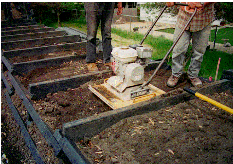
Figure 4.6: Soil Compaction in the Recywall (14)
