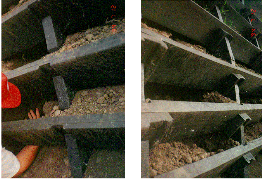
Figure 4.7: Soil Loss in Plating Cells (14)
