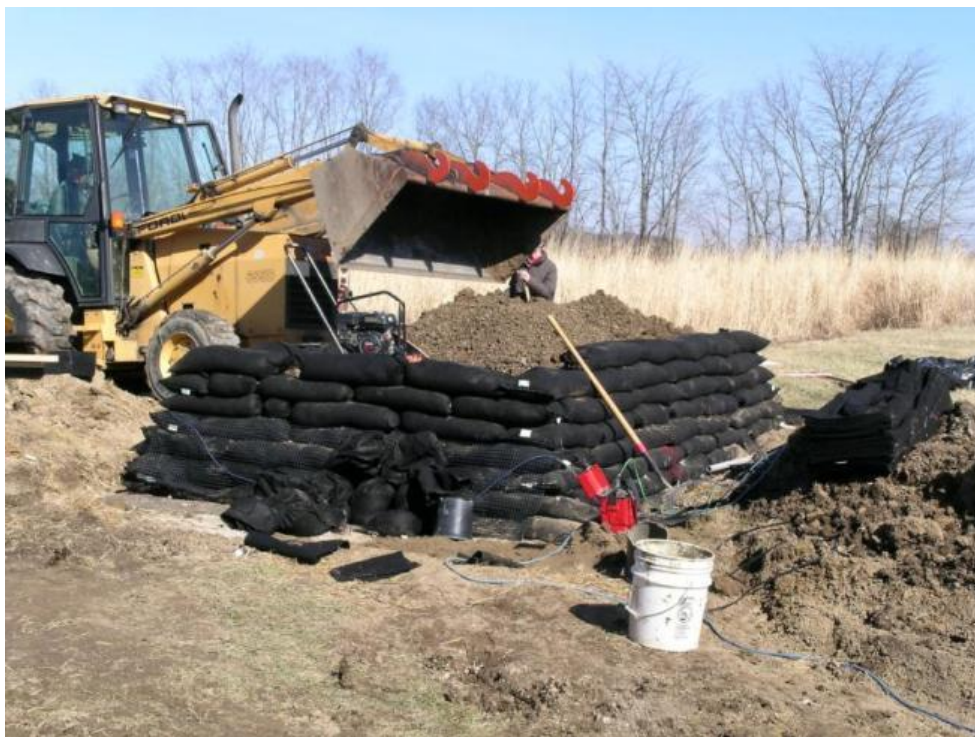
Figure 5.11: Wall Backfill
