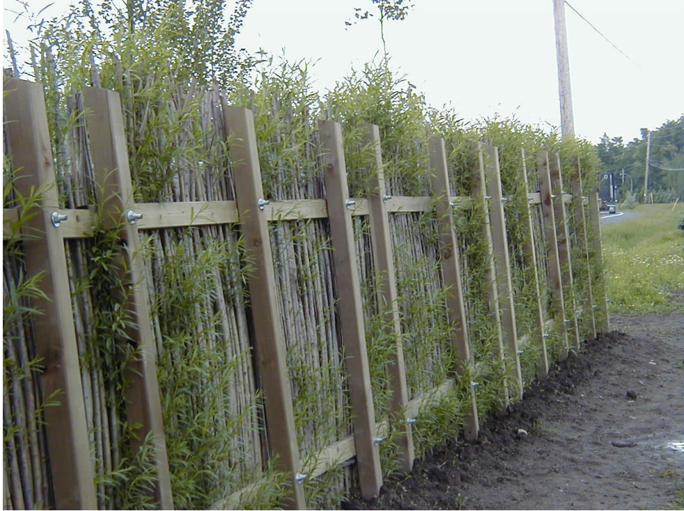
Figure 3.3: Living Willow Wall Shortly after Construction (9)
