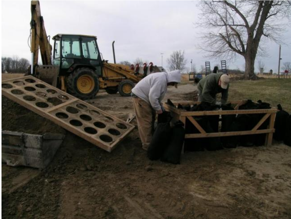
Figure 5.6: Closing the Bags using Zip Ties
