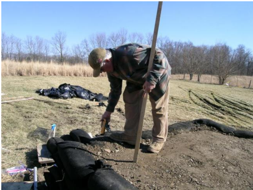
Figure 5.15: Checking the Wall Height
