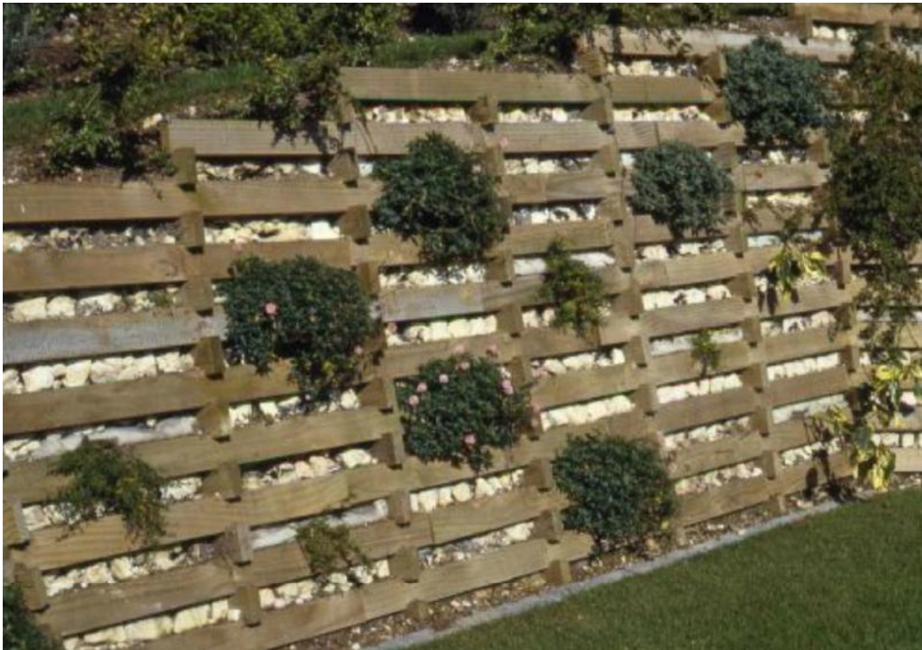
Figure 3.19: Timbergrid Wall with Planting Bags (12)
