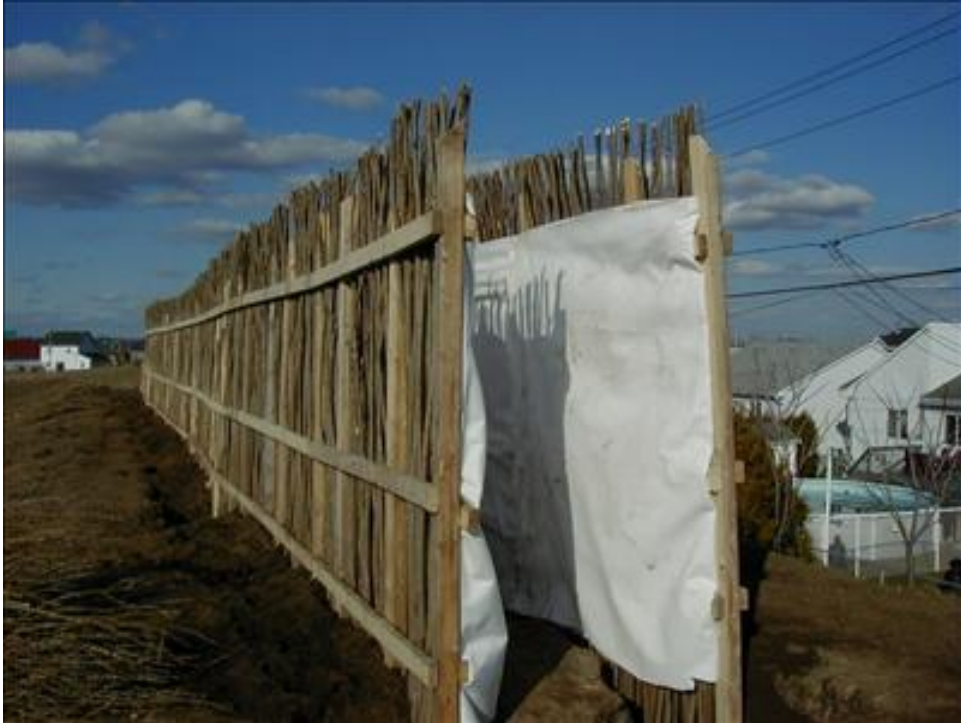
Figure 3.2: Construction of the Living Willow Wall (9)
