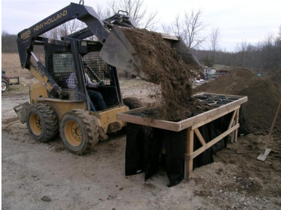
Figure 5.4: Filling the Deltalok Bags
