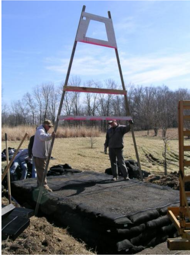
Figure 5.16: Checking Angle with A-Frame
