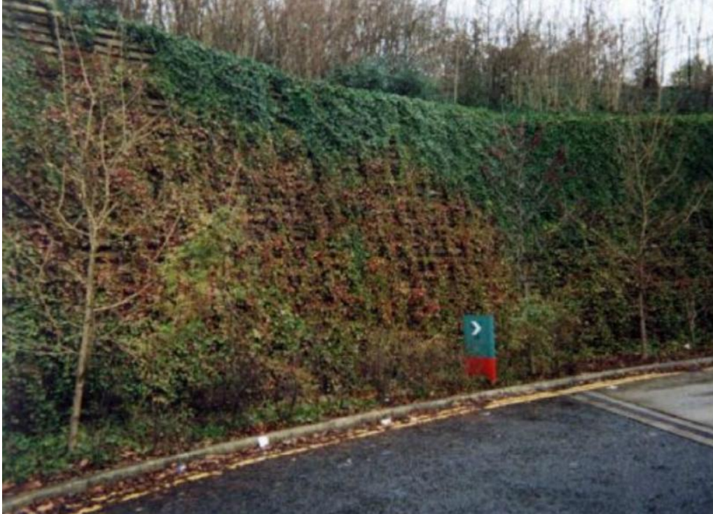
Figure 3.20: Timbergrid Wall Planted with a Mixture of Ivy and Virginia Creeper (12)
