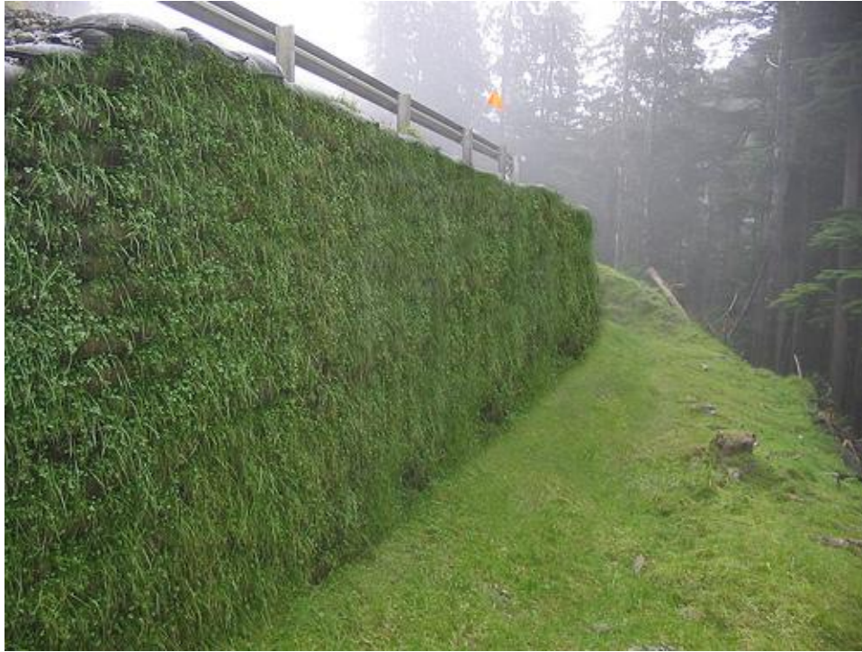
Figure 3.30: Deltalok Retaining Wall Fully Covered with Vegetation (16)
