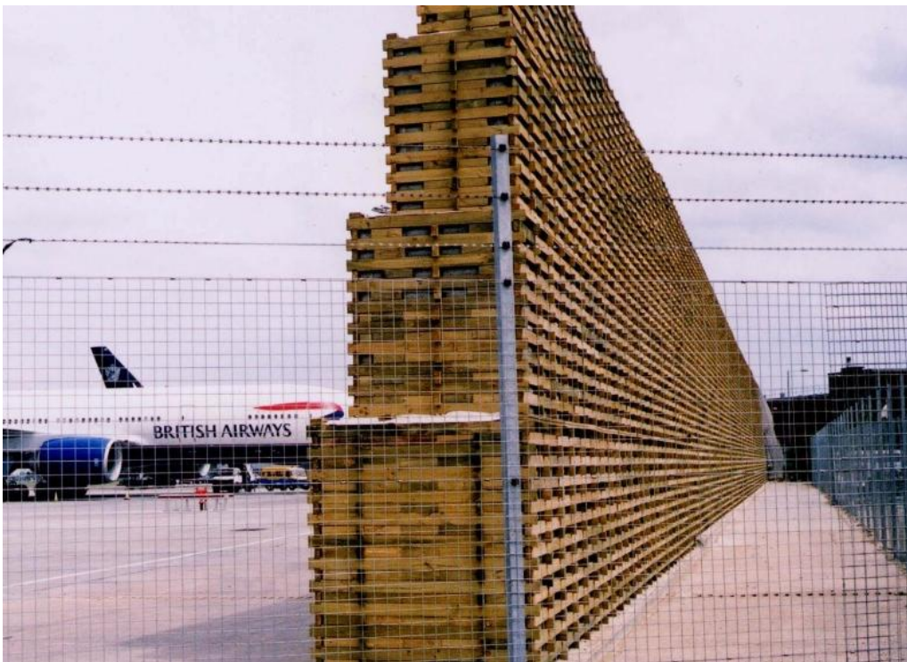
Figure 3.21: Timbergrid as a Noise Barrier (12)
