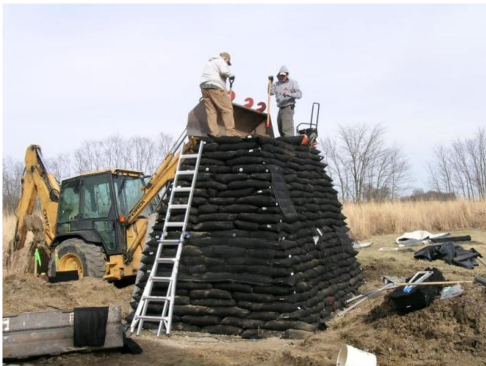
Figure 5.13: Construction at Higher Height Levels
