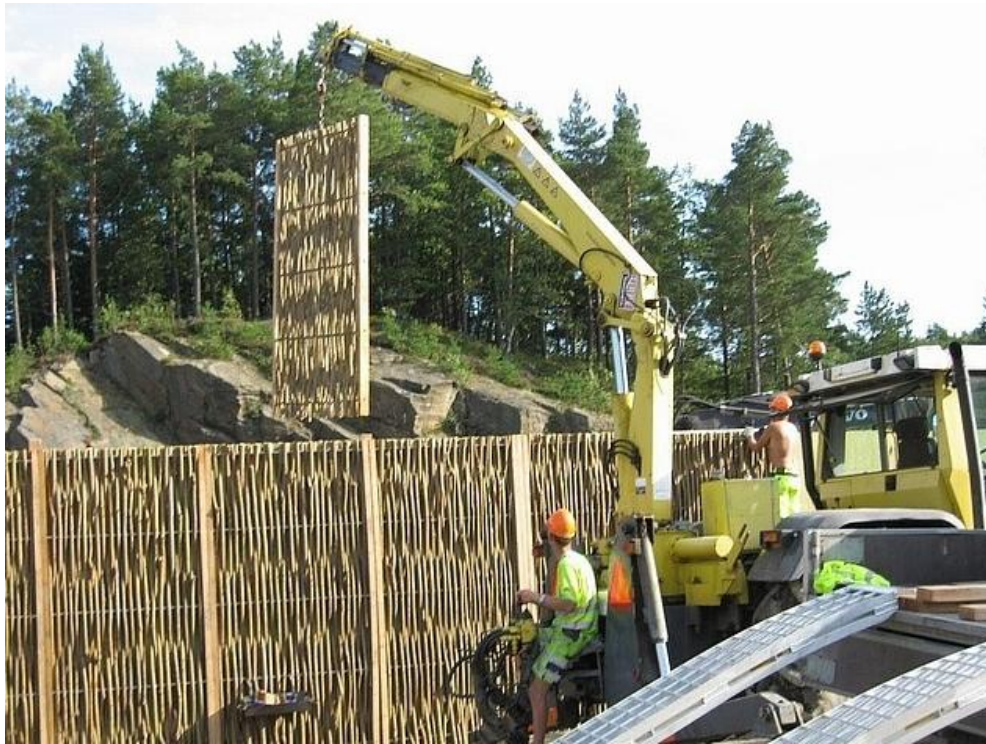
Figure 3.6: Construction of the Dry PileByg Structure (10)
