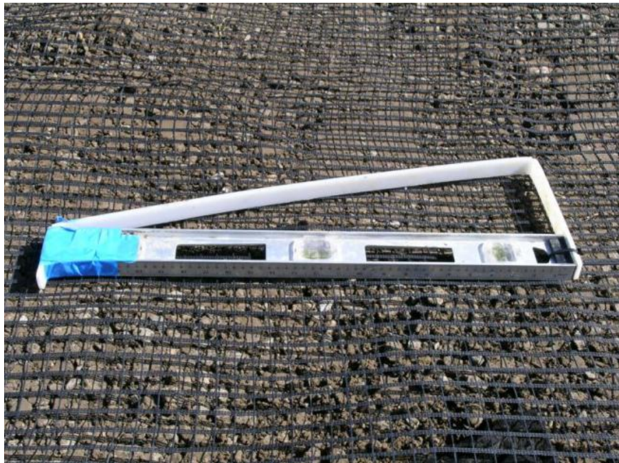
Figure 5.17: Checking Angle with Triangle Jig
