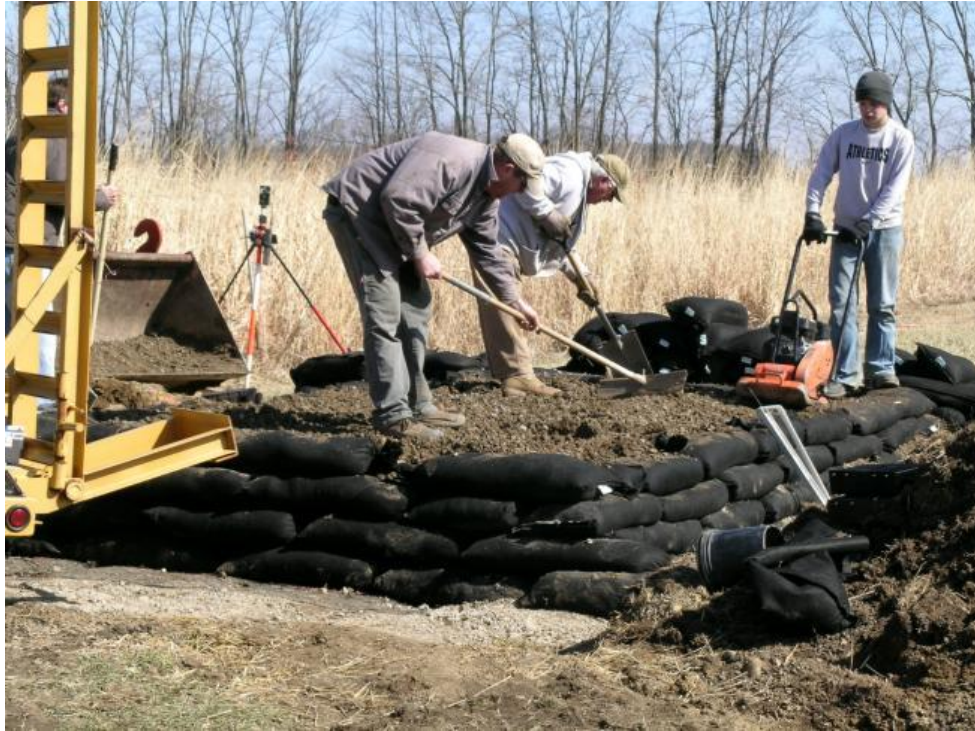
Figure 5.12: Backfill Compaction
