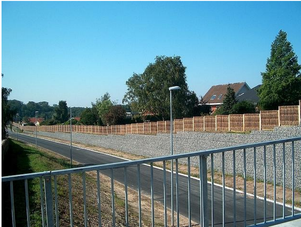
Figure 3.8: Picture of the Dry PileByg Structure (10)
