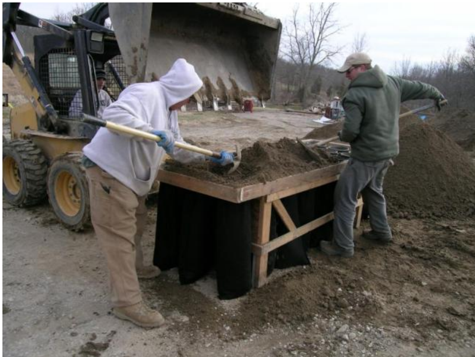
Figure 5.5: Pushing the Soil into the Bags
