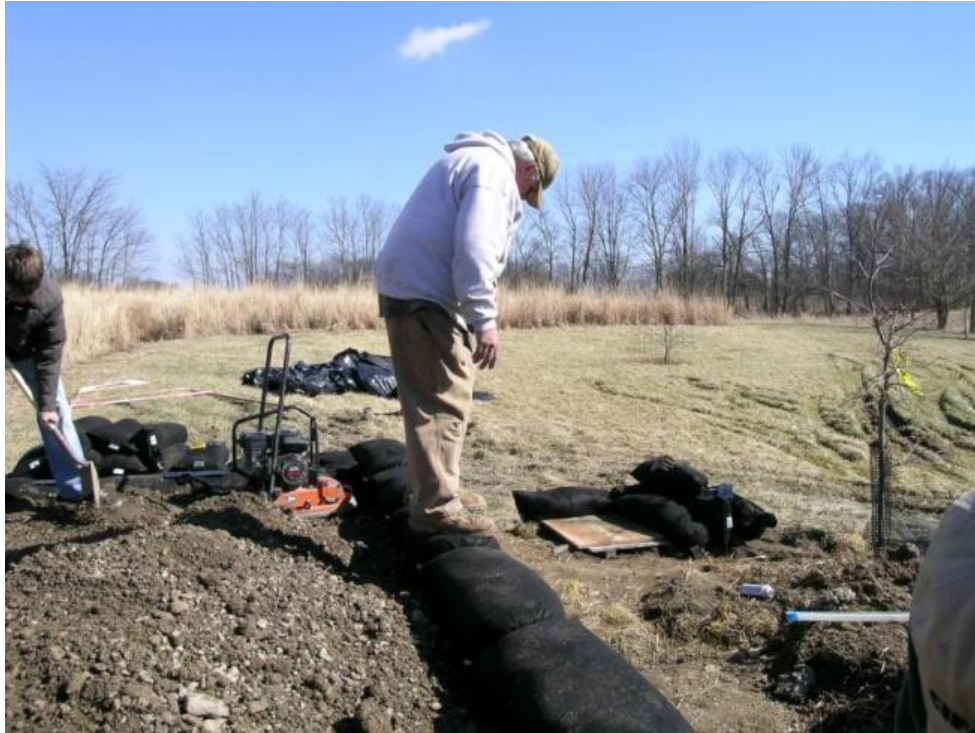
Figure 5.10: Stepping on the Bags to Engage the Deltalok Units
