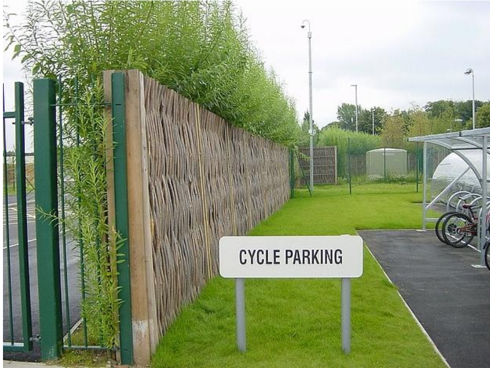
Figure 3.11: Picture of the Living PileByg Structure, Dry Façade (10)
