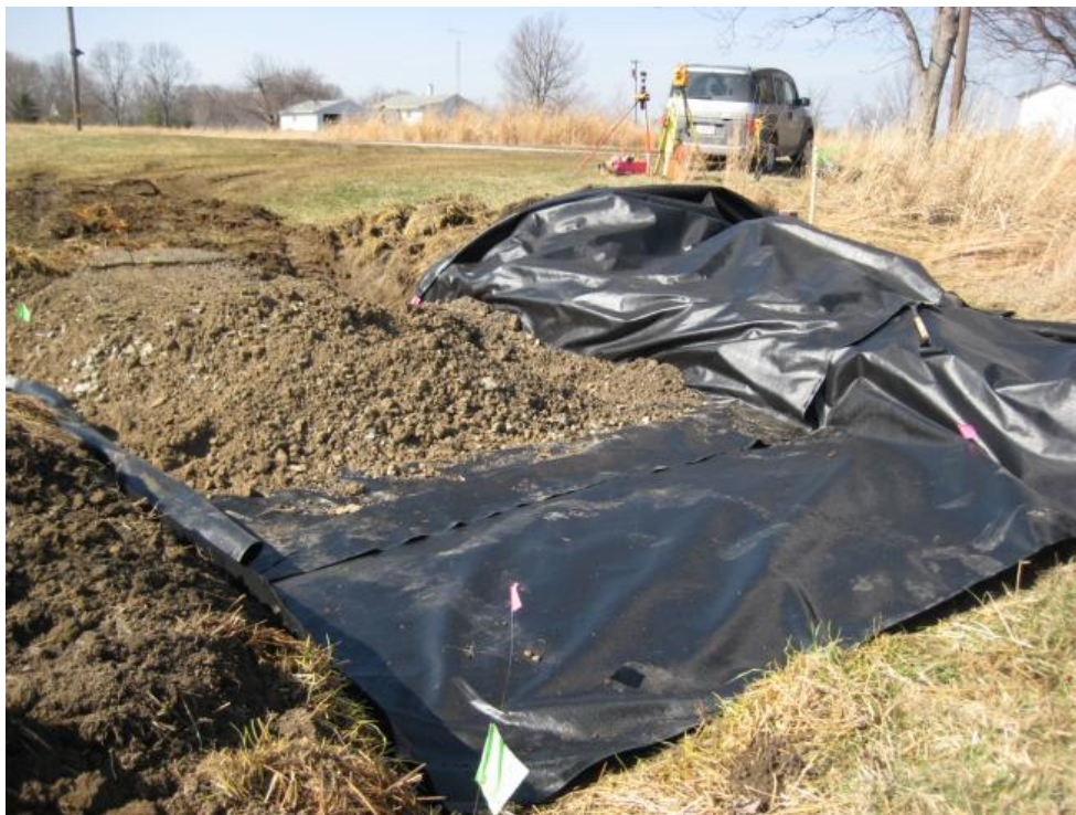
Figure 5.8: Geotextile Fabric and Base Course
