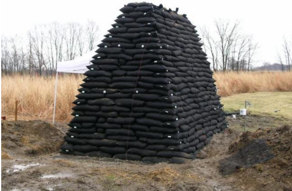
Figure 5.18: Completed Prototype Wall
