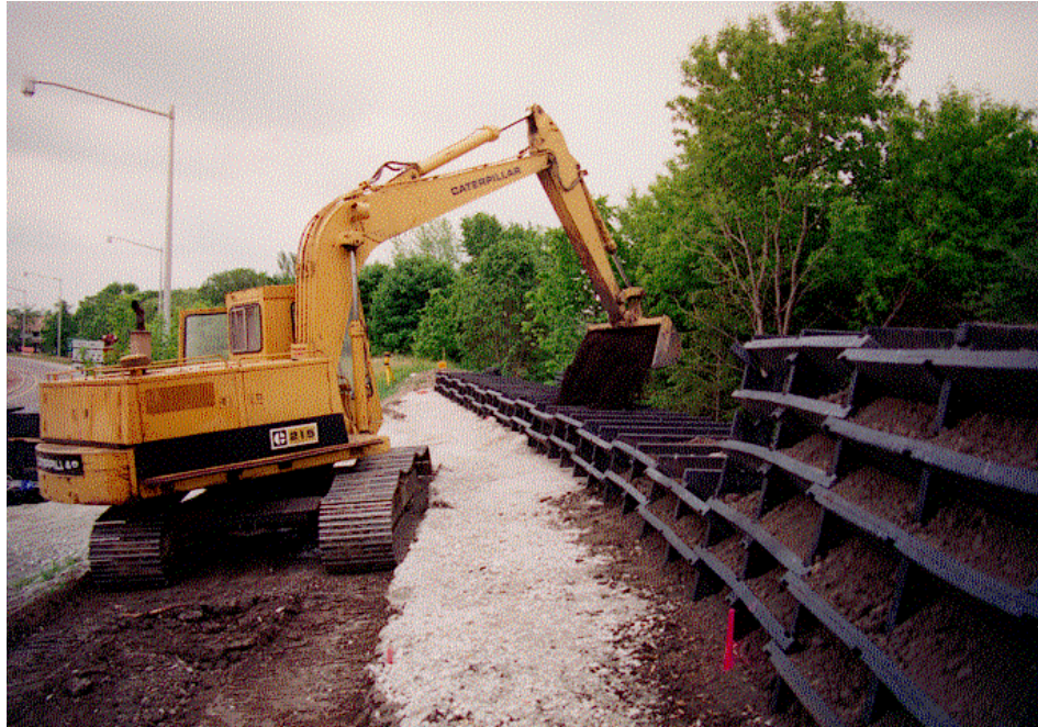
Figure 4.5: Filling the Recywall with Soil (14)
