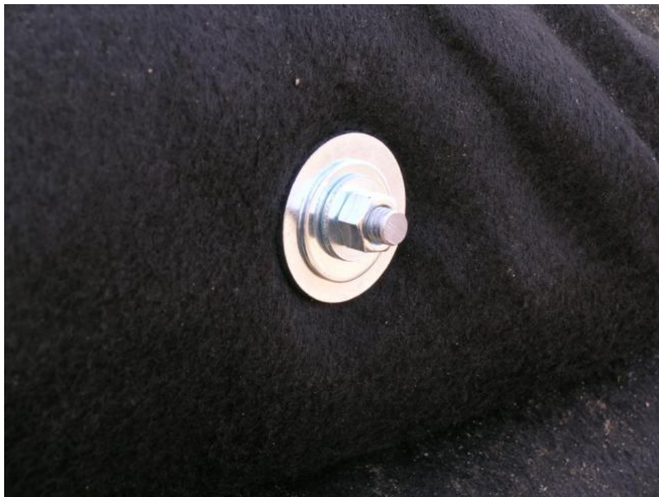
Figure 6.6: Survey Point (After Installation)
