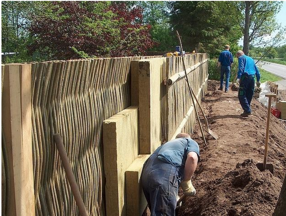
Figure 3.10: Construction of the Living PileByg Structure (10)
