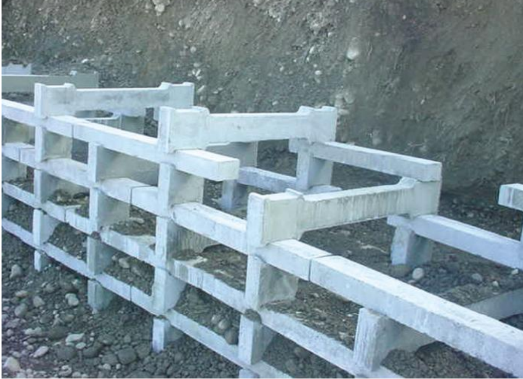
Figure 3.14: Soil Backfilling in the Cribblock Wall (11)
