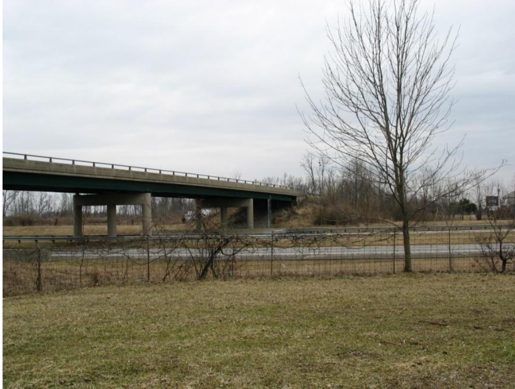
Figure 9.2: Picture at Phase II Barrier Site Showing Interstate 70 and the Tollgate Road Overpass
