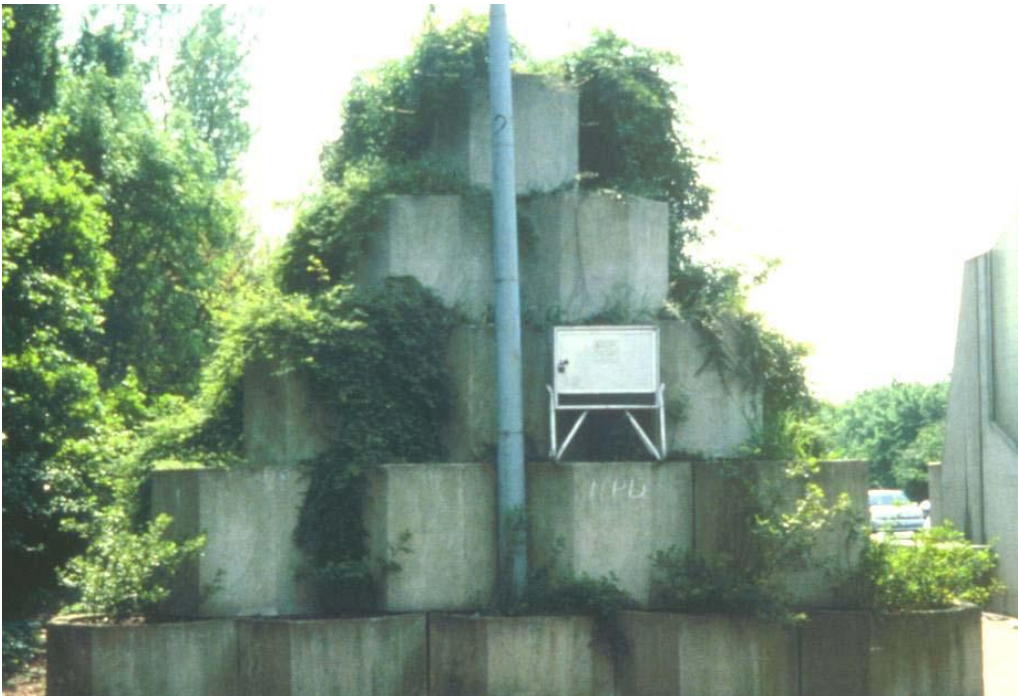
Figure 3.27: Supported Earth Embankment with Concrete (15)
