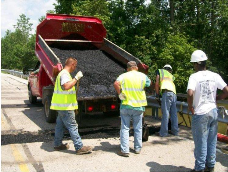
**Figure 20: Cold Patch Placement**
