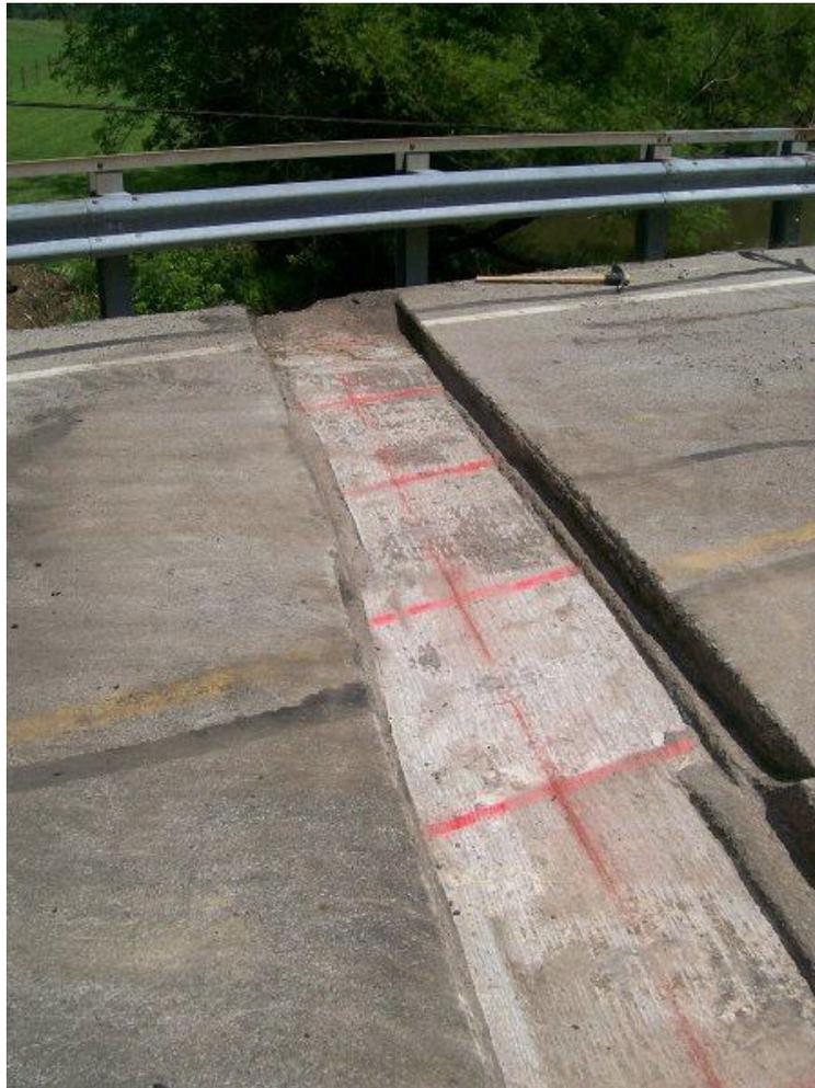
**Figure 17: Asphalt Removed**
