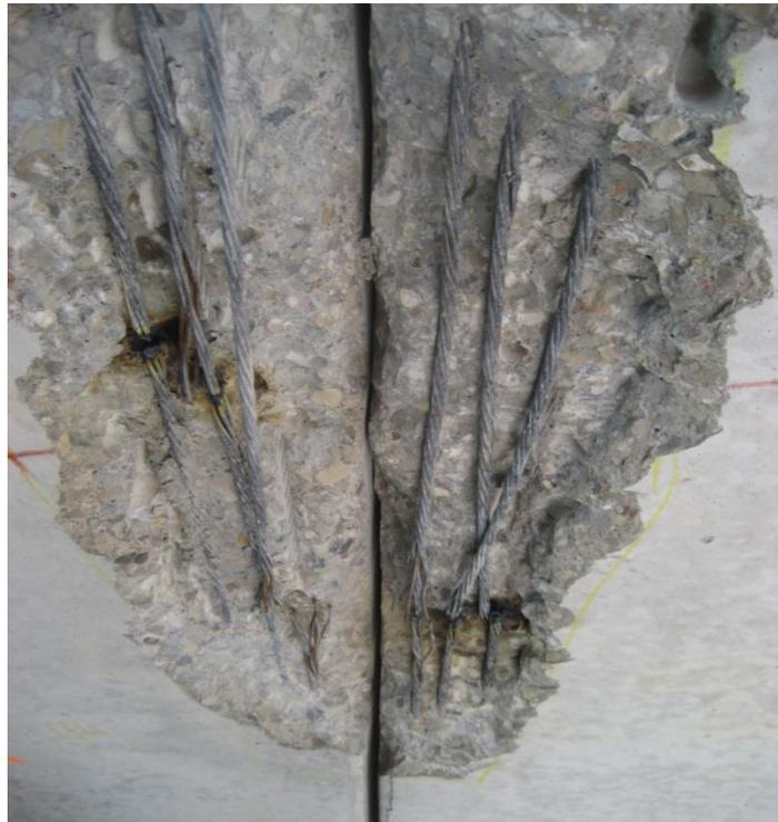
**Figure 35: Exposed and Cut Strands – East Span**
