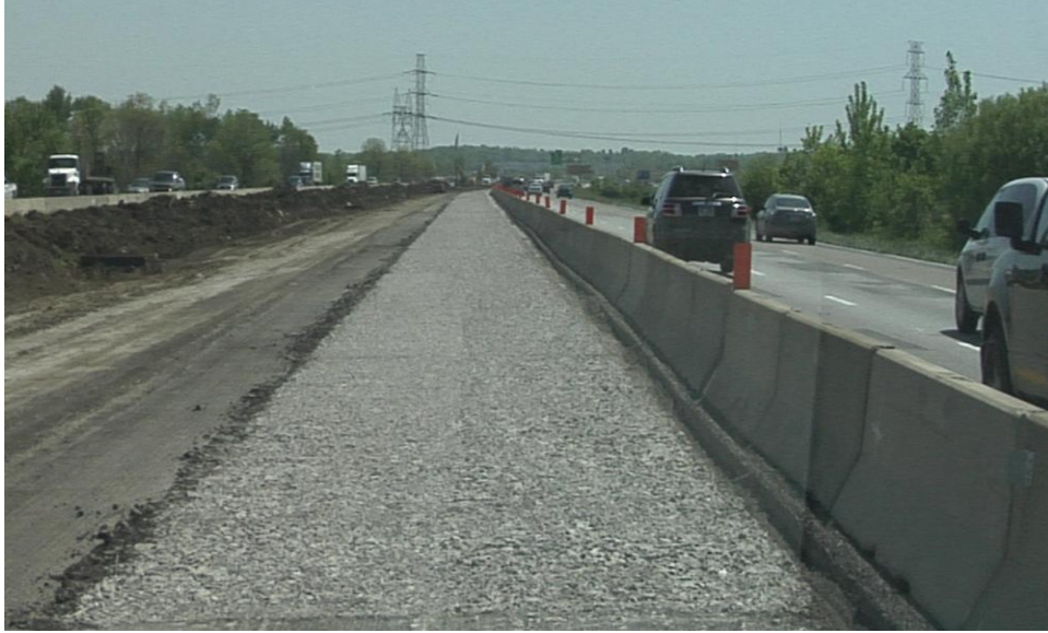
Figure 5. Particle Size Observed on the Surface of Rubblized Layer
