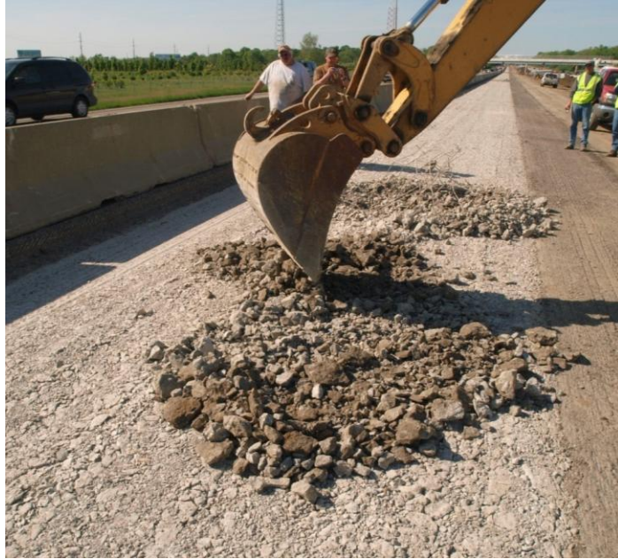
Figure 25. Making a Test Pit to Expose the Material through the Depth
