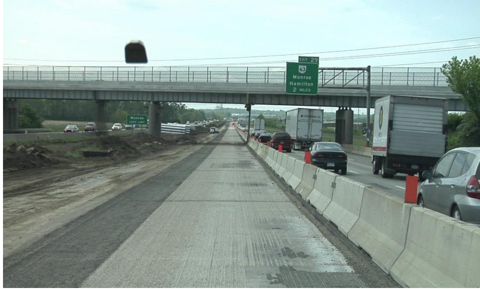
Figure 1. Asphalt Concrete Layer Milled to Expose Concrete Pavement Prior to Rubblization
