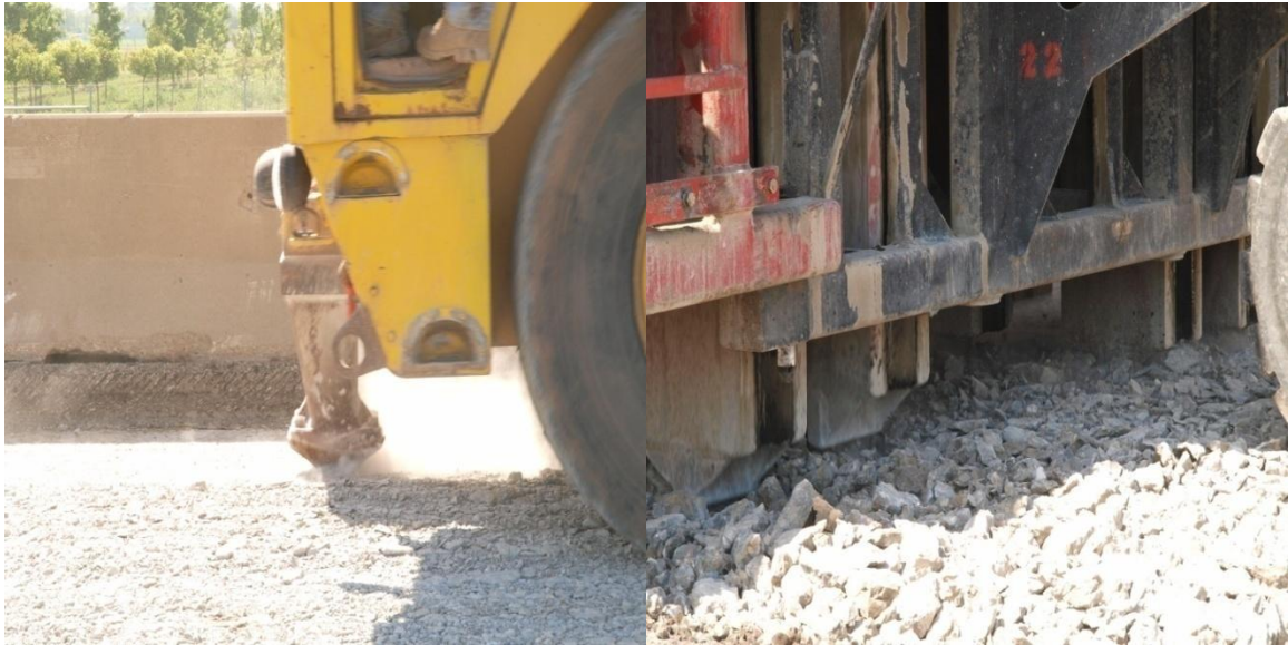
Figure 2. Rubblization using Resonant Machine and Multi Head Breaker
