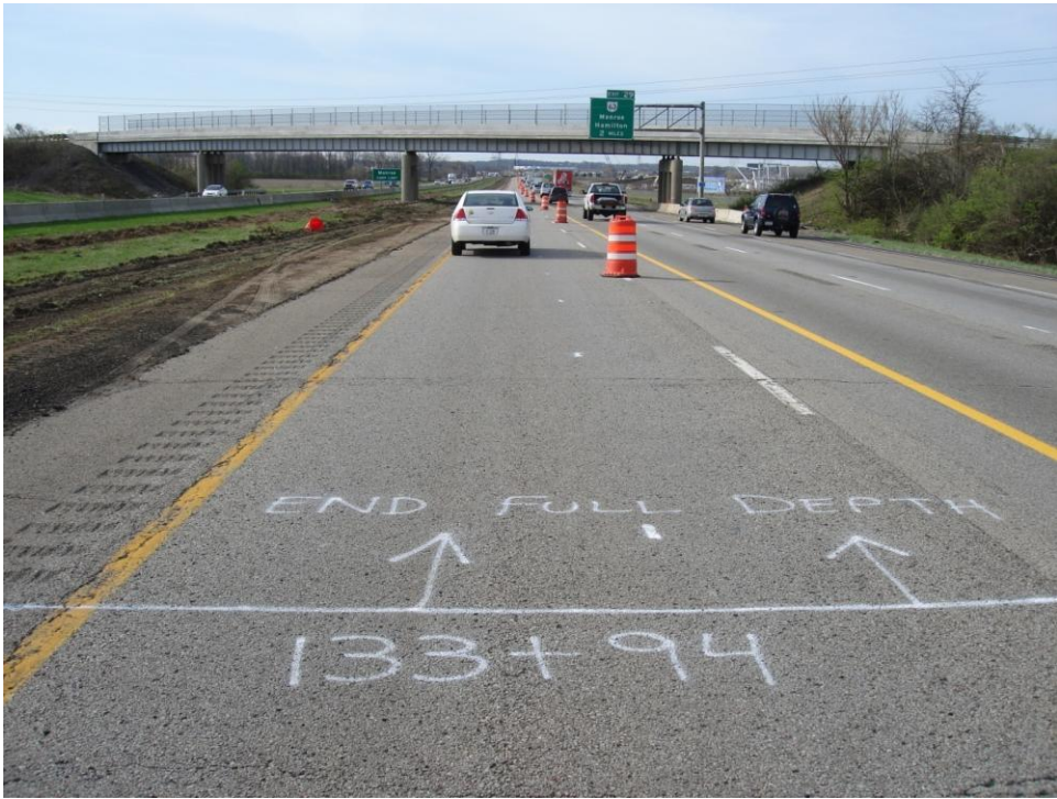
Figure 11. General Condition of Project – In-service Composite Pavement, Prior to Milling
