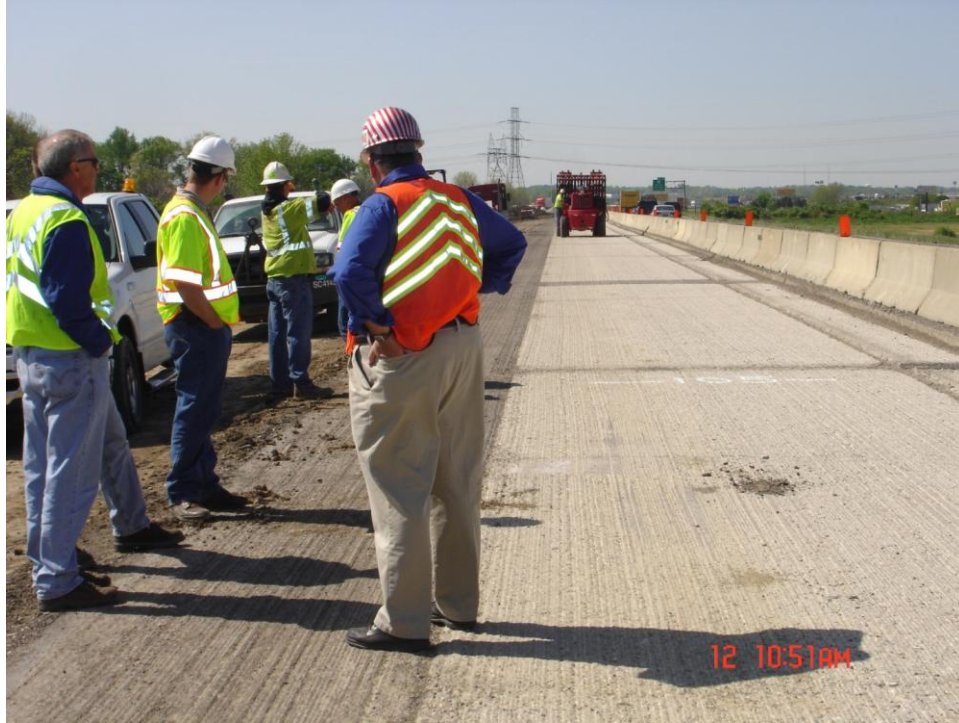
Figure 12. Exposed Concrete Pavement After Milling the AC Layer
