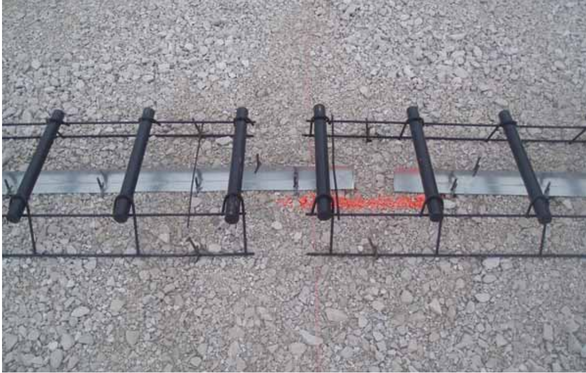
Figure 8. Typical cross-section of metal angles placed on the base materials
