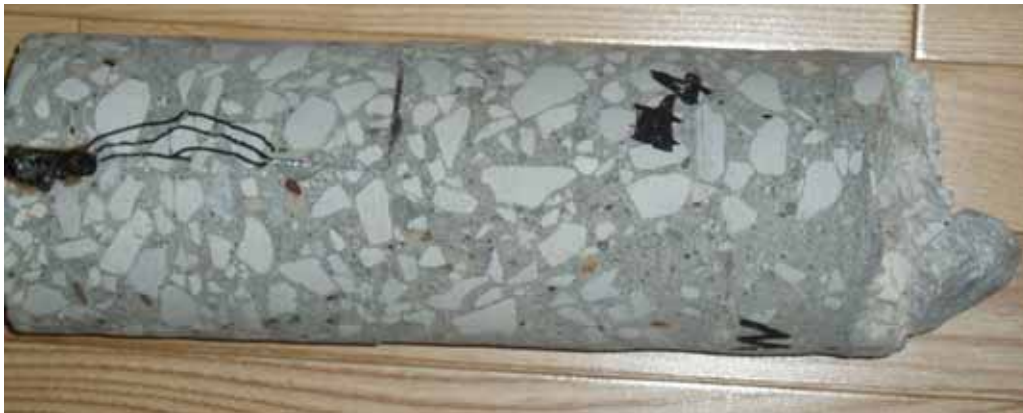
Figure G5. Crack in test section 4 core
