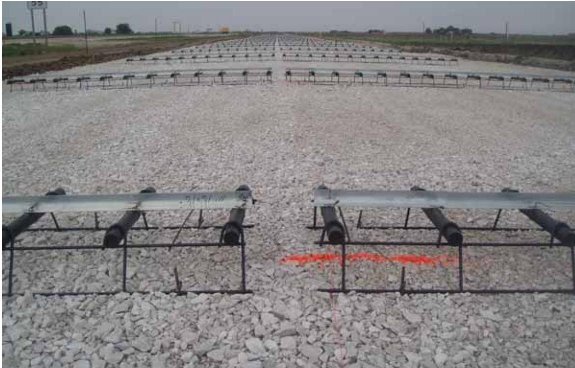
Figure 7. Typical cross-section of metal angles placed over dowels
