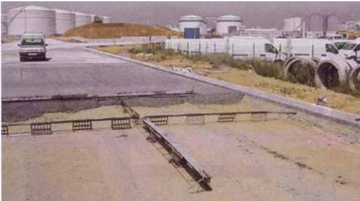
Figure 1. JRI+ joint before concrete placement
