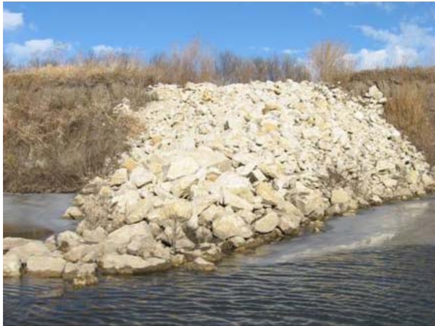
Figure 2. Typical bendway weir design as constructed at the Raccoon River study site. Picture taken from the channel center looking perpendicular at bank with flow going from left to right. The bridge (not pictured) is located downstream of this structure.
