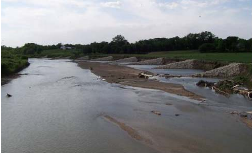
Figure 3. Constructed bendway weirs looking upstream from the U.S. Highway 169 Bridge.
