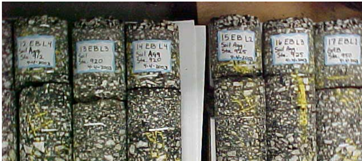
Figure 3-22. I-20 cores showing stripping from 4 to 6 inches from the surface
