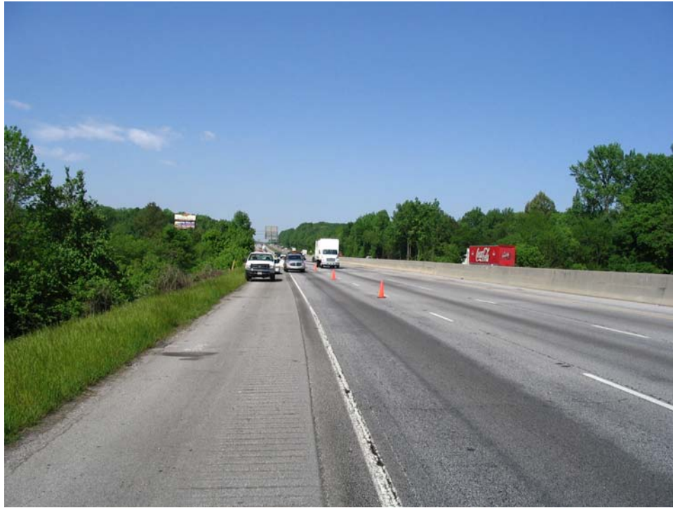
Figure 3-2. Photograph of I-20 eastbound lanes looking west
