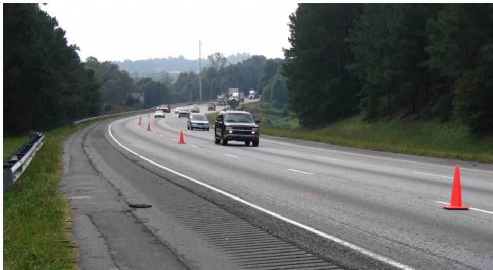
Figure 4-2. Photo of I-75 northbound lanes near MP 270.5
