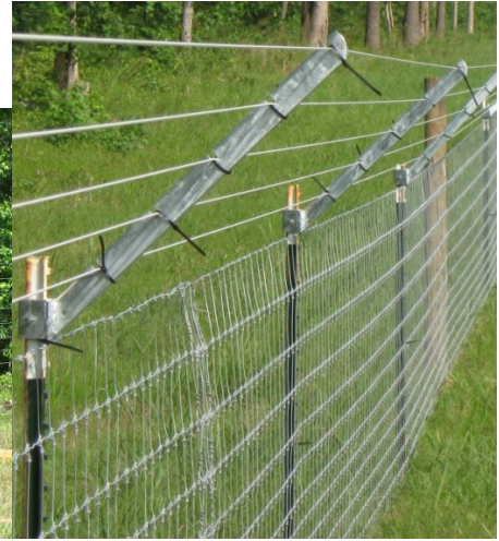
Figure 1.1. The 2.4-m woven-wire fence treatment (left) and outrigger fence treatment (right) constructed on Berry College, Floyd County, Georgia.
