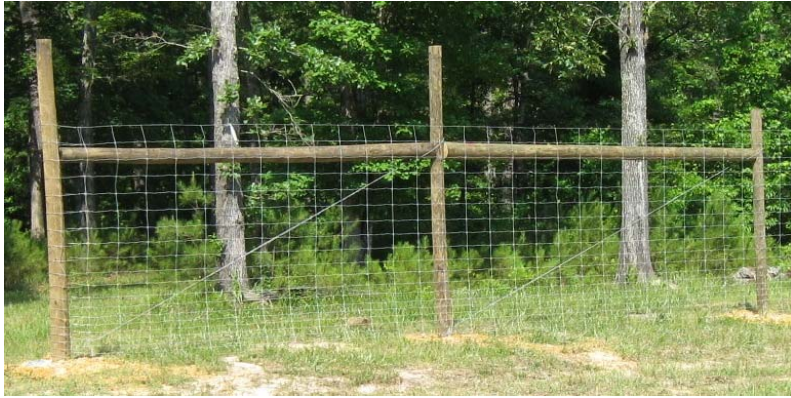
Figure 1.1. The 2.4-m woven-wire fence treatment (left) and outrigger fence treatment (right) constructed on Berry College, Floyd County, Georgia.
