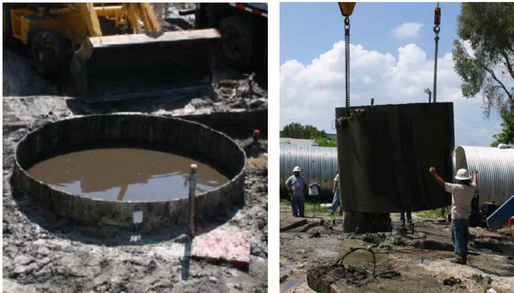
Figure 2.9 Temporary surface casing (left) after extraction (right).
