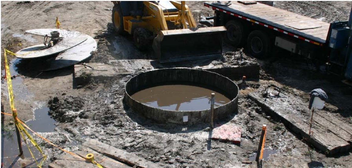
Figure 1.1 Slurry-stabilized drilled shaft excavation with temporary surface casing.
