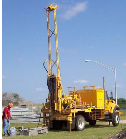
Figure 2.7 Truck-mounted drill rig
