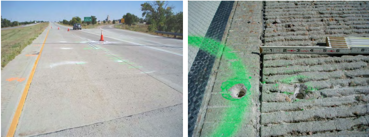
Figure 25. Control Joints A, B, and C (left) and close-up of Control Joint B (right).
