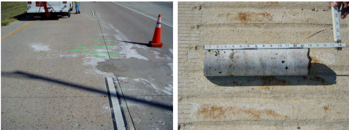
Figure 25. Control Joints A, B, and C (left) and close-up of Control Joint B (right).
