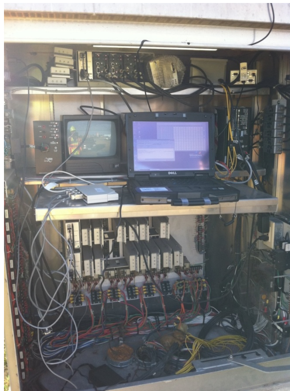
Figure 18. Toolbox Implementation at SH 6 and FM 60 Site.
