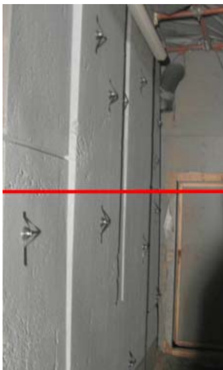
Figure 4.41: South face of the east pier divided into two sections, high and low sand content. Low sand content section is below the red line in the picture.
