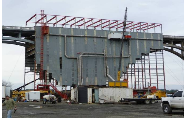
Figure 4.7: Containment enclosure at the McCullough Bay Bridge.
