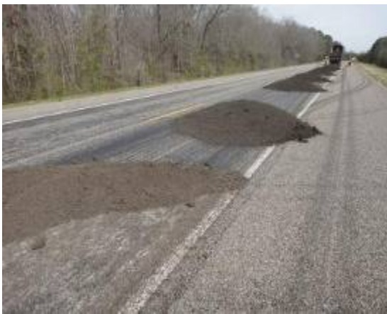
b) Placing Material
