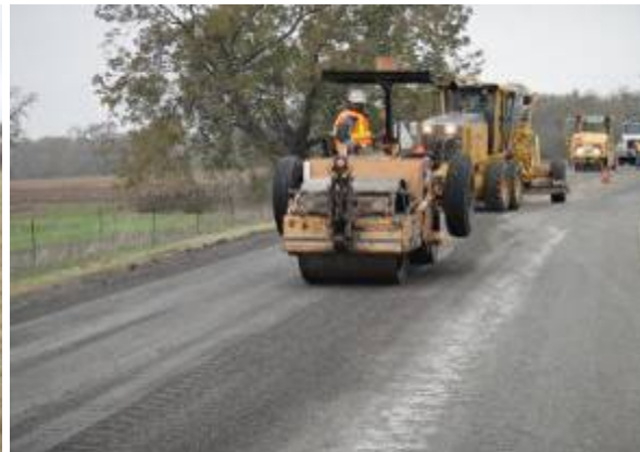
f) Small Steel Wheel Roller
