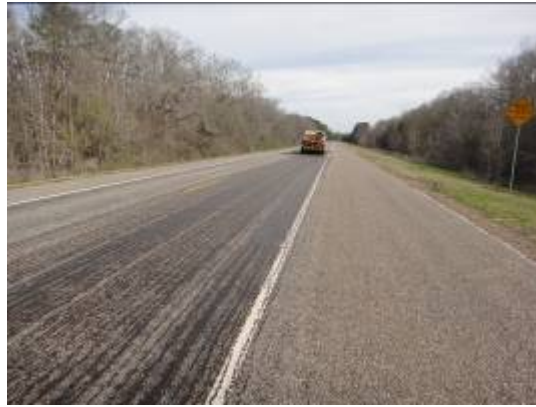
a) Application of Tack
