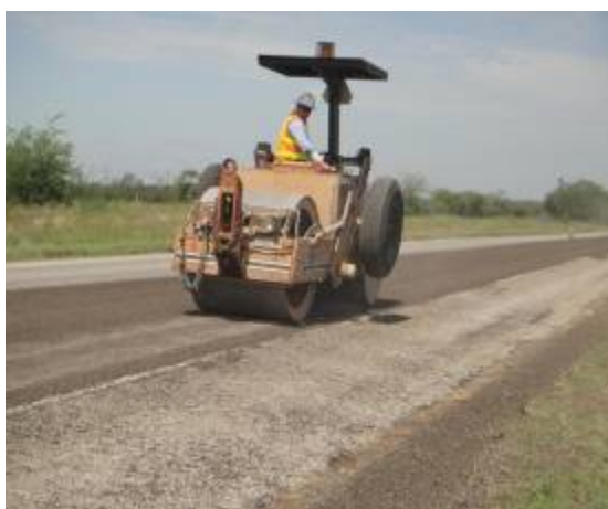
e) Small Steel Wheel Roller
