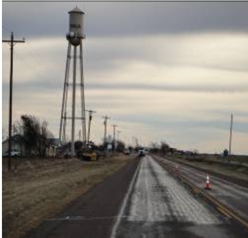
a) Application of Tack
