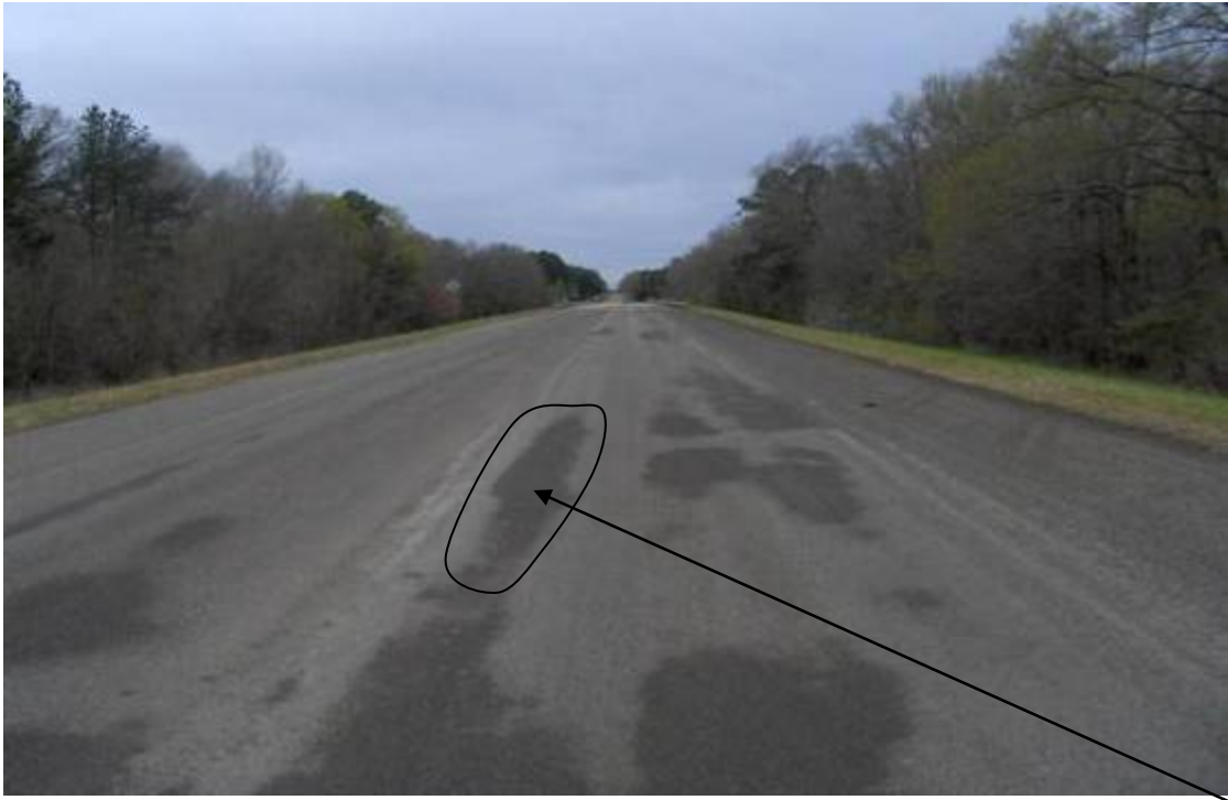
(a) Areas of Low Density Holding Water (Small Potholes Developed in Wheelpath (Martin Marietta DS).
