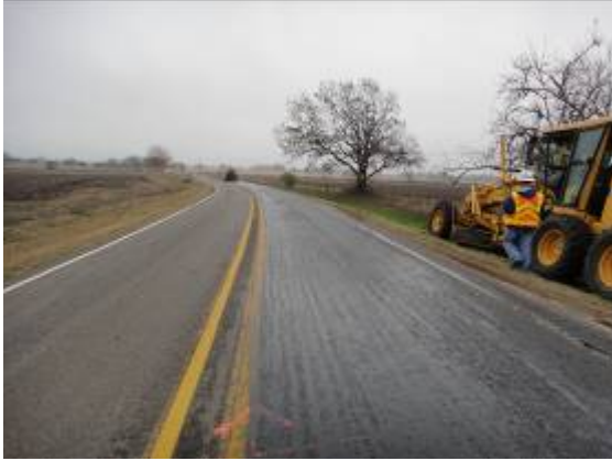
a) Application of Tack
