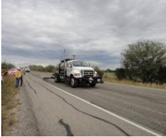
a) Application of Tack
