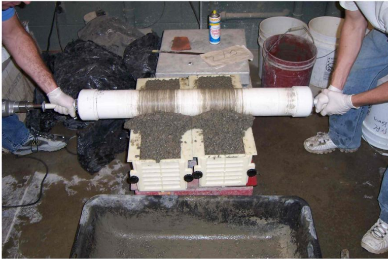
Figure 35. Finishing using a roller screed
