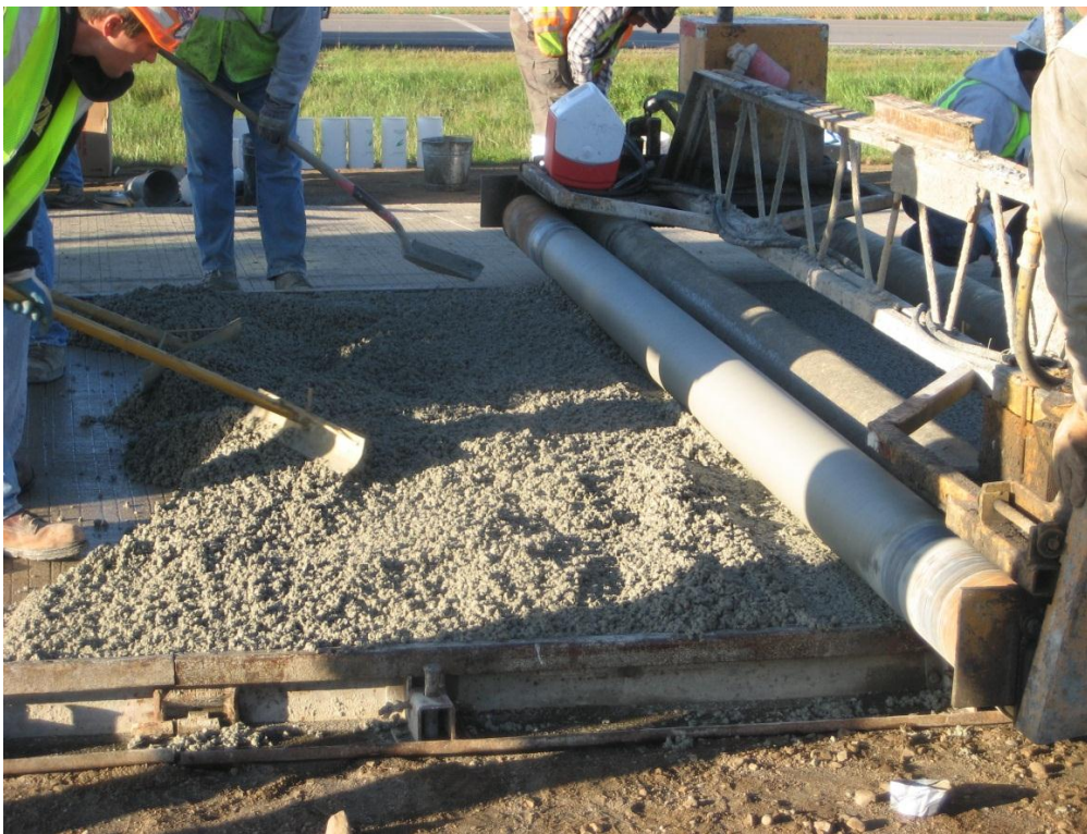
Figure 59. Placement of pervious concrete overlay using roller-screed
