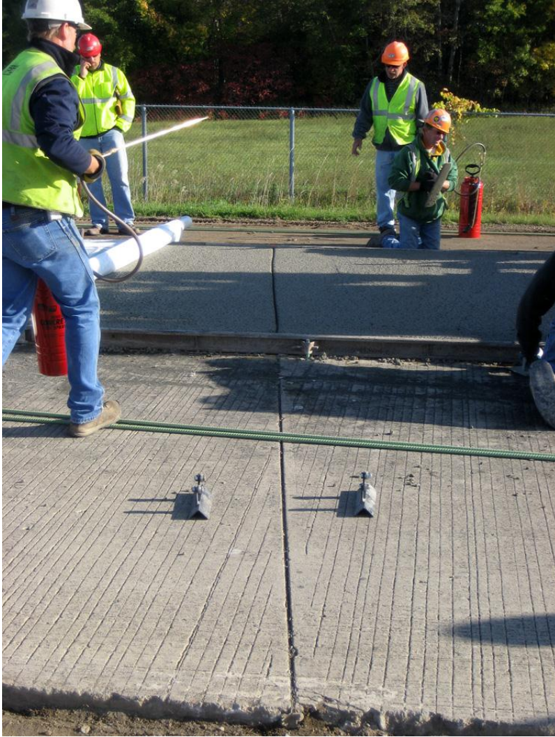
Figure 72. Jointing on fresh pavement
