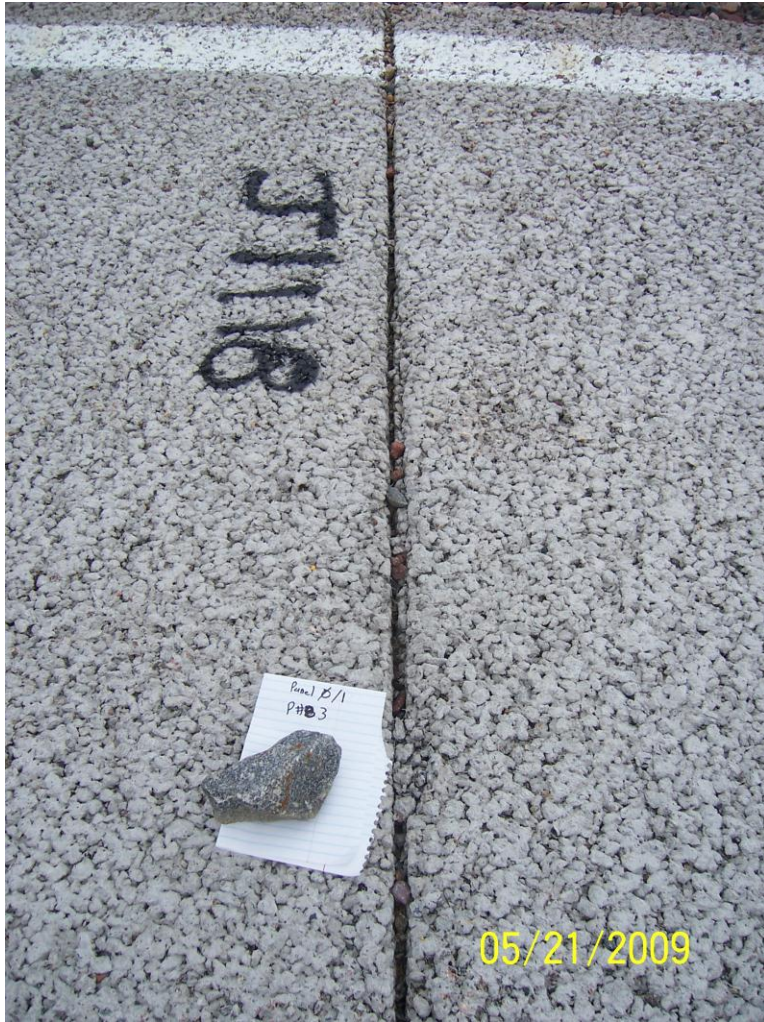
Figure 70. Example of double-jointing
