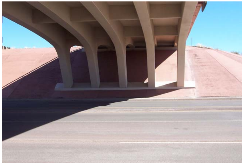
FIGURE 2 K-Frames of Bridge 7937.
