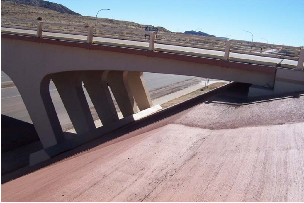
FIGURE 2 K-Frames of Bridge 7937.
