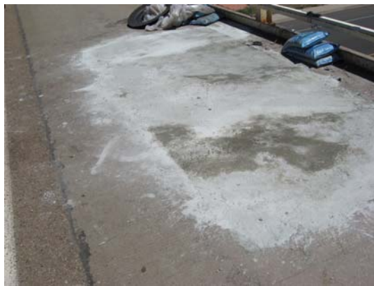
FIGURE 16 Top of Bridge Deck after Concrete Casting Showing the Connection of the Sensors to the Monitoring Box Under the Bridge
