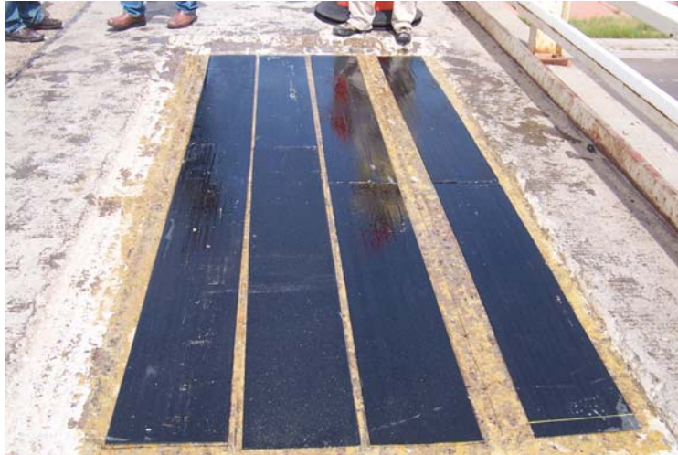
FIGURE 3 FRP Sheets Installed on Bridge 7937.
