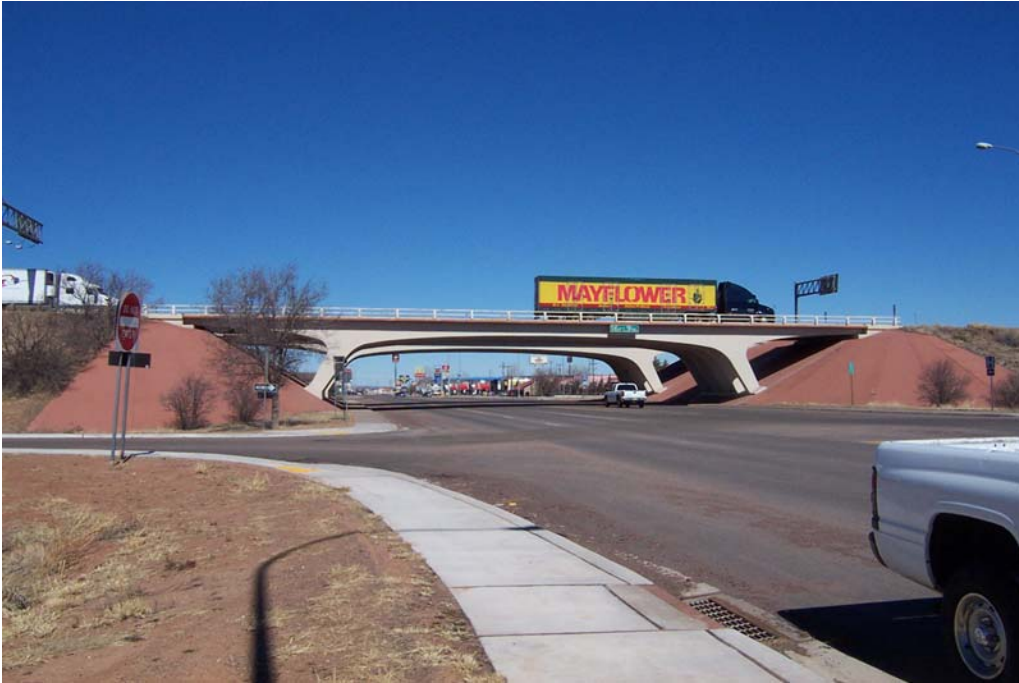
FIGURE 1 Bridge 7937 at Tucumcari.
