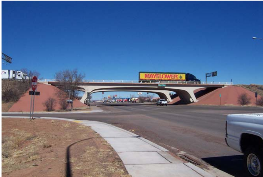
FIGURE 1 Bridge 7937 at Tucumcari.
