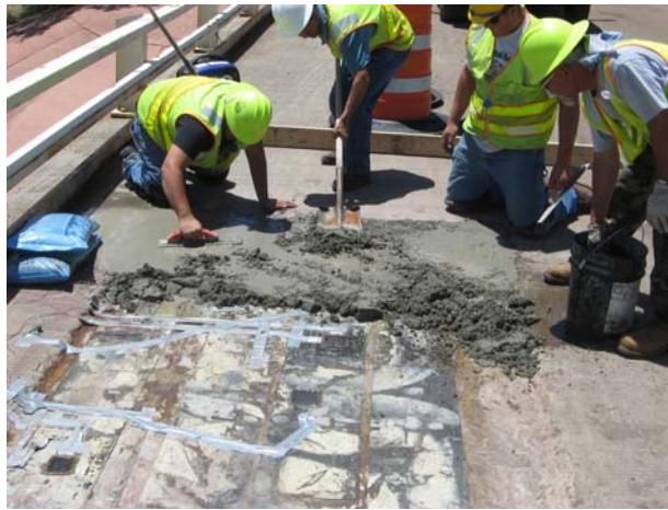
FIGURE 15 Concrete Casting Over Area of Bridge Deck Strengthened with FRP
