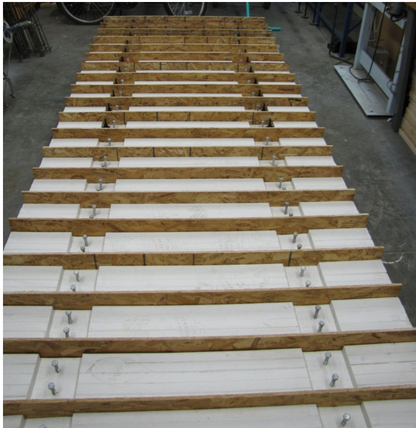
Figure 2.3 Specimens under construction with exposed notch detail
