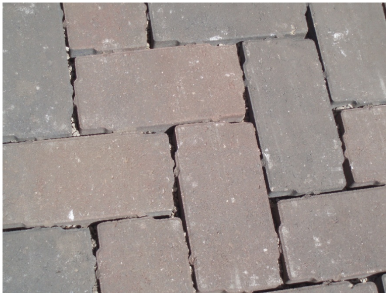
Figure 11: Successful vacuuming of A-3 soil when surface was saturated with water
