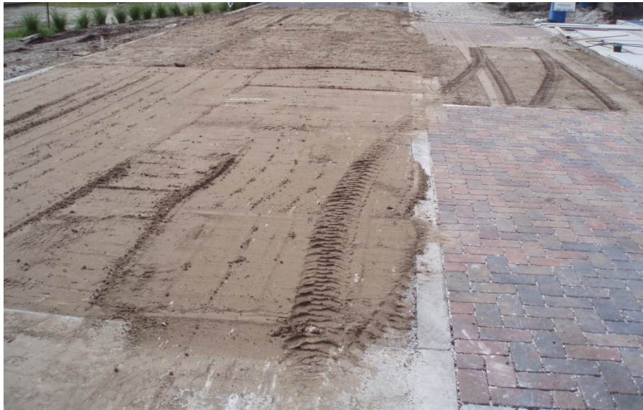
Figure 8: Spreading of A-3 sediments evenly over entire Rejuvenation section
