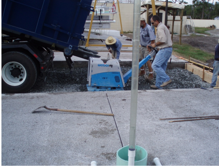
Figure 6: Aggregates placed, leveled, then compacted
