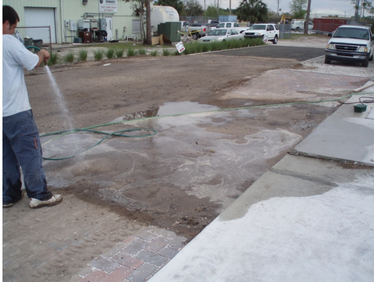
Figure 9: Washing in A-2-4 soils with garden hose
