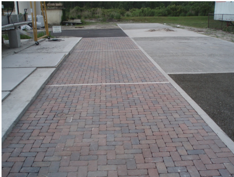
Figure 7: Final Layout of Pervious Pavement Sections with ERIKS
