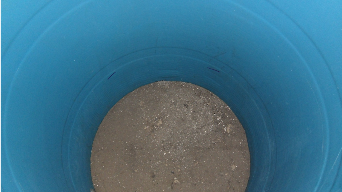
Figure 20: 4 Inches of Compacted AASHTO Type A-3 Soil Installed
