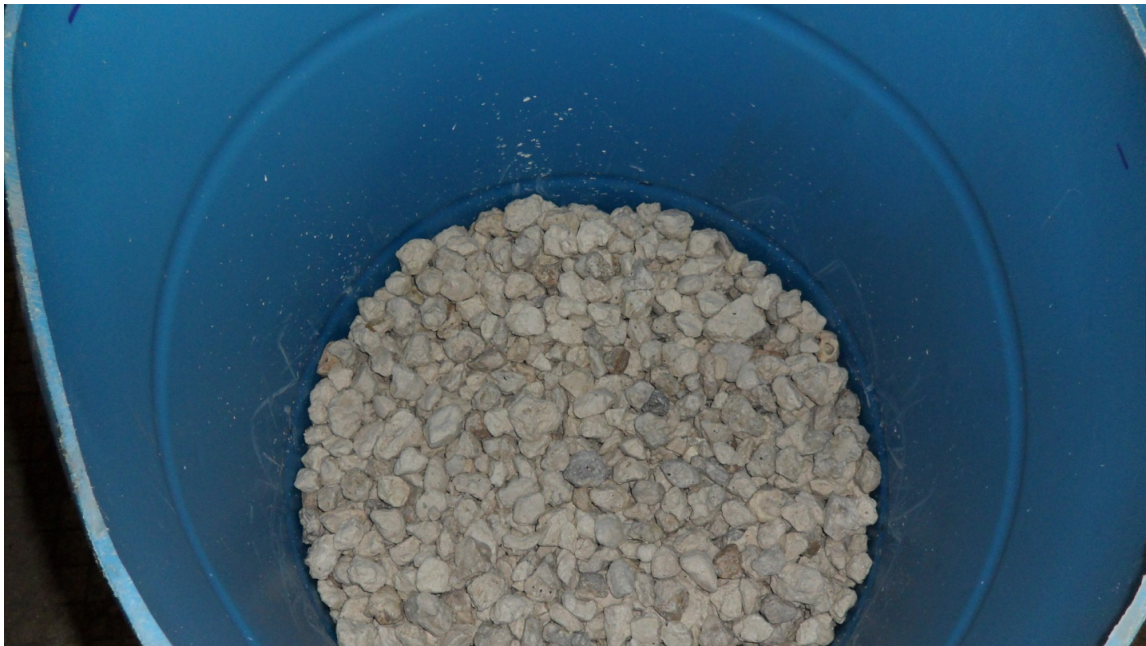
Figure 24: 4 Inches of #57 Stone Compacted
