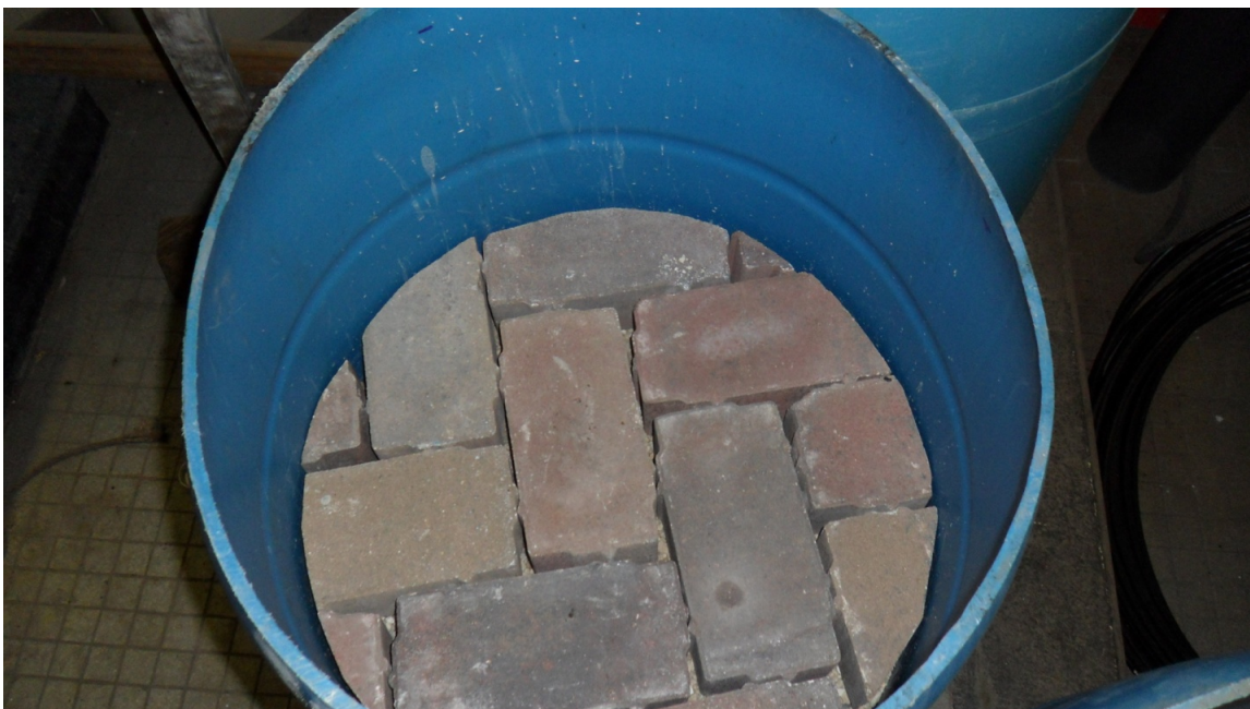
Figure 26: Oldcastle Brick Pavers Installed
