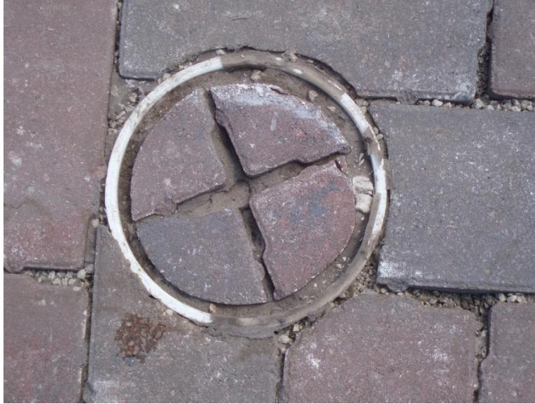
Figure 10: Unsuccessful vacuuming of A-3 soils when dry and hardened
