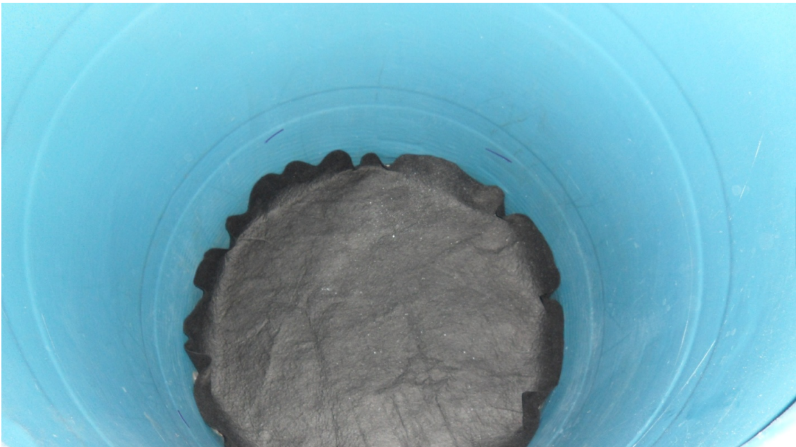
Figure 21: Non-woven Geotextile Separation Fabric Installed
