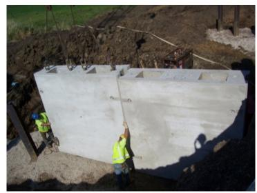
Precast abutments like these being placed at a bridge site near Baldwin, Wis., can reduce bridge construction time from two weeks to under two days.
