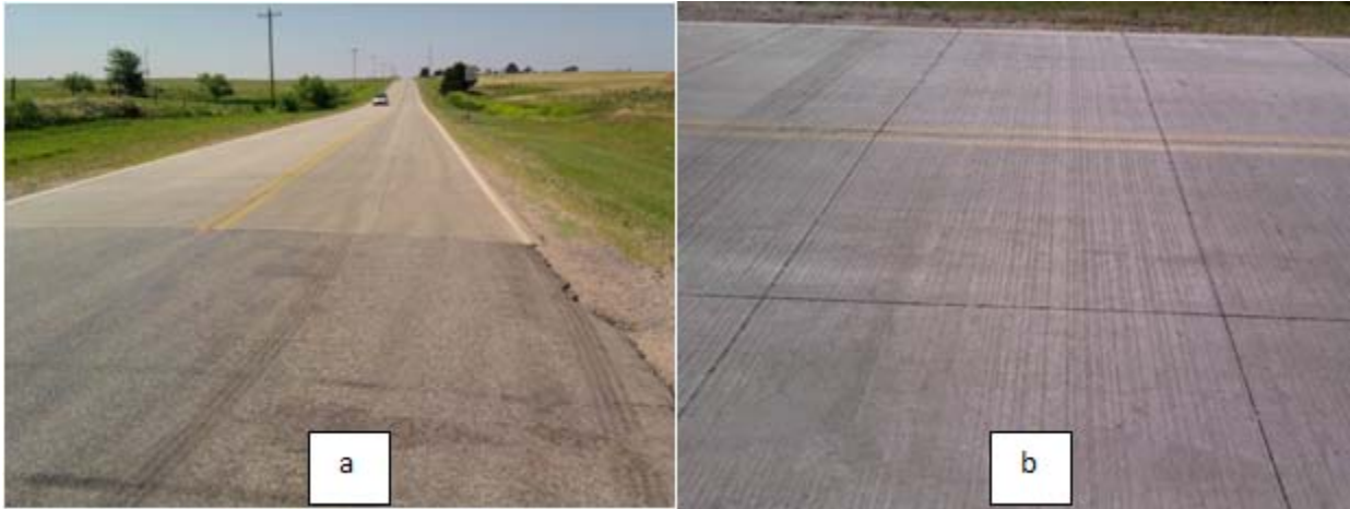
Figure 2.52 - North end of overlay. Photo a is taken looking towards south direction. Photo b is seven panel series from the end of the overlay.
