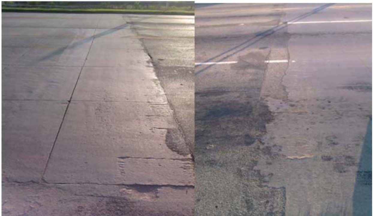
Figure 2.34 - Photo of intersection seen on US 177 towards south-west showing excellent condition of overlay.
