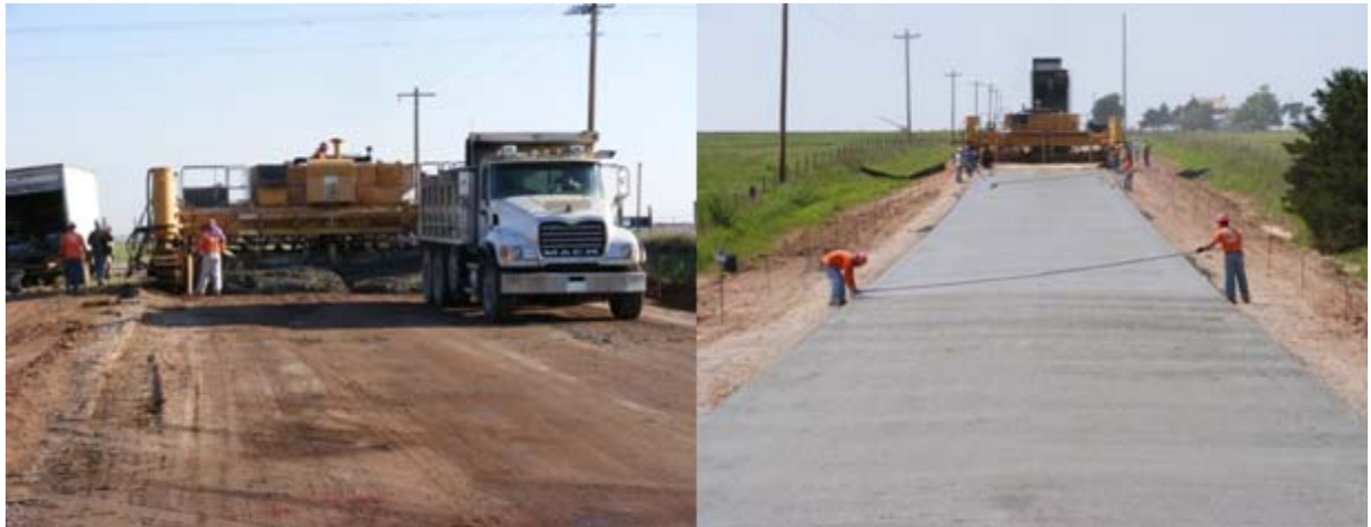
Figure 2.48 - Photos show the construction of the overlay.
