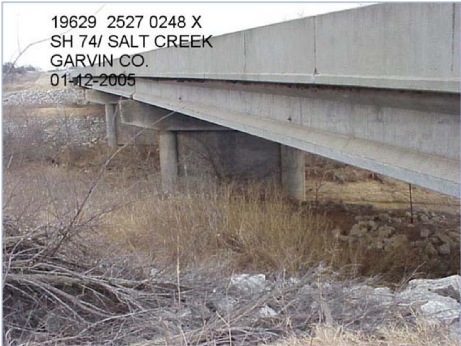
Figure 33. Picture demonstrating extent of damage to piers at bridge 19629 on SH 74 over Salt Creek.
