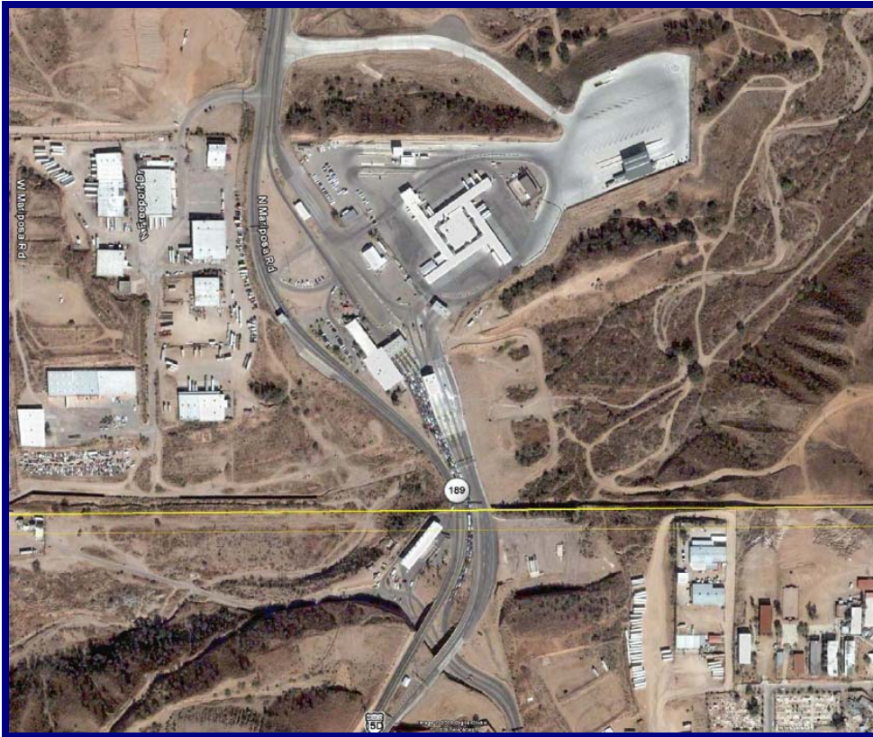
Mariposa Port of Entry
