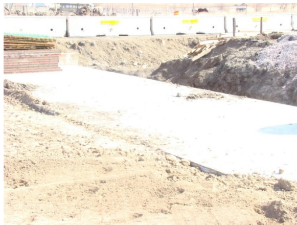
(b) Backfill around the Structure
