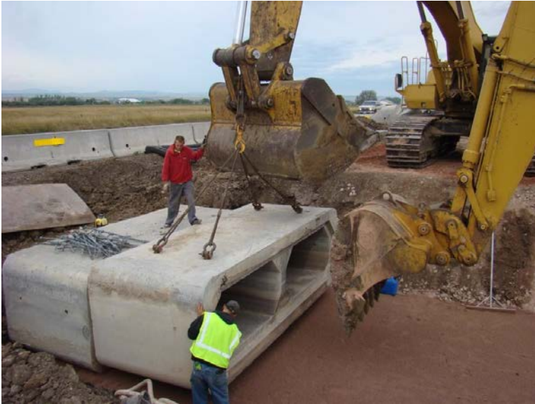
Figure 5.5 Assembly of the Precast Units of Structure #52-485-337
