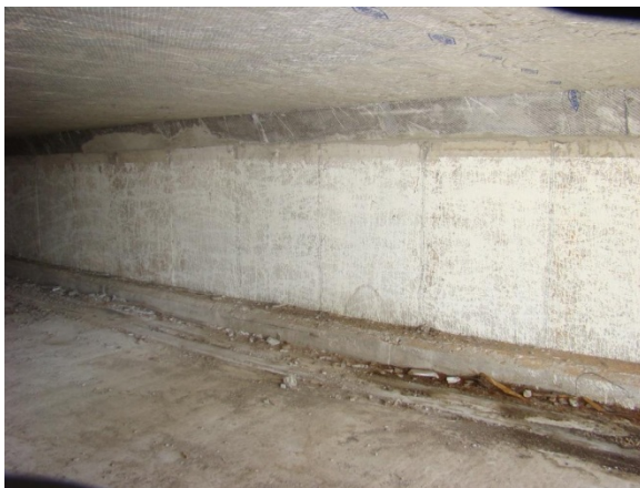
(a) Finished Wall Interior Surface
