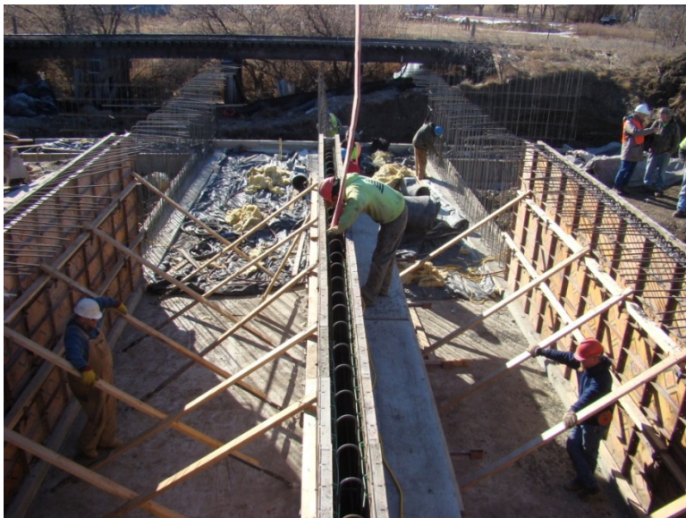
Figure 5.8 Casting of the SCC Mix in Structure #52-489-339
