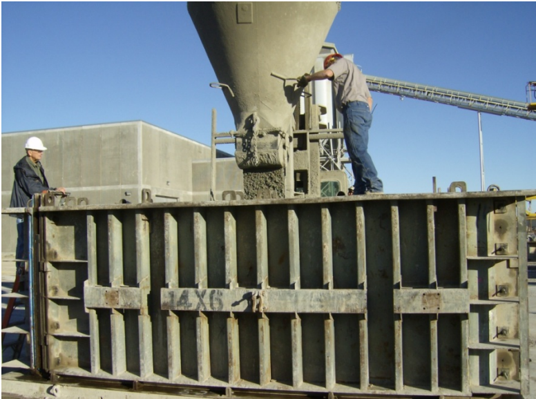
Figure 5.2 Casting of an SCC Box Culvert Unit
