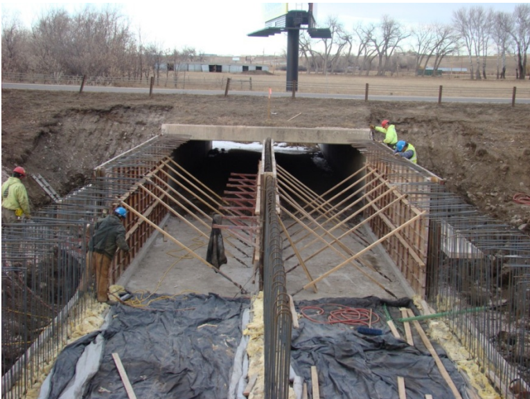
Figure 5.6 The Extension of Structure #52-489-339 under Construction
