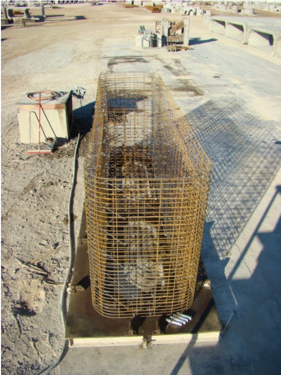
Figure 5.1 Reinforcement Cage of an SCC Box Culvert Unit
