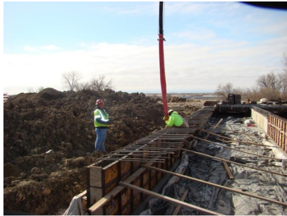
(b) Concrete Placement
