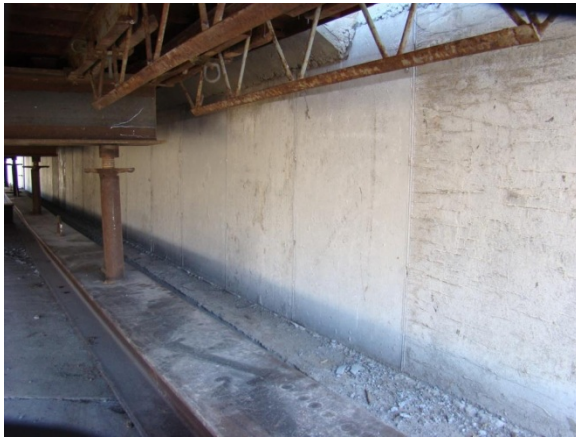
(a) Finished Wall Interior Surface
