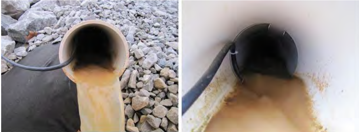
Figure 3.6: ISCO 750 Flow Module connected to the outflow pipe of the basin 4.
