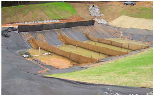
(a) Basin 4 after construction
