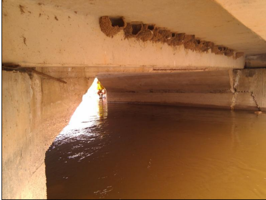
FigureE.52 Bridge 15 Widened with Double T-Girder
