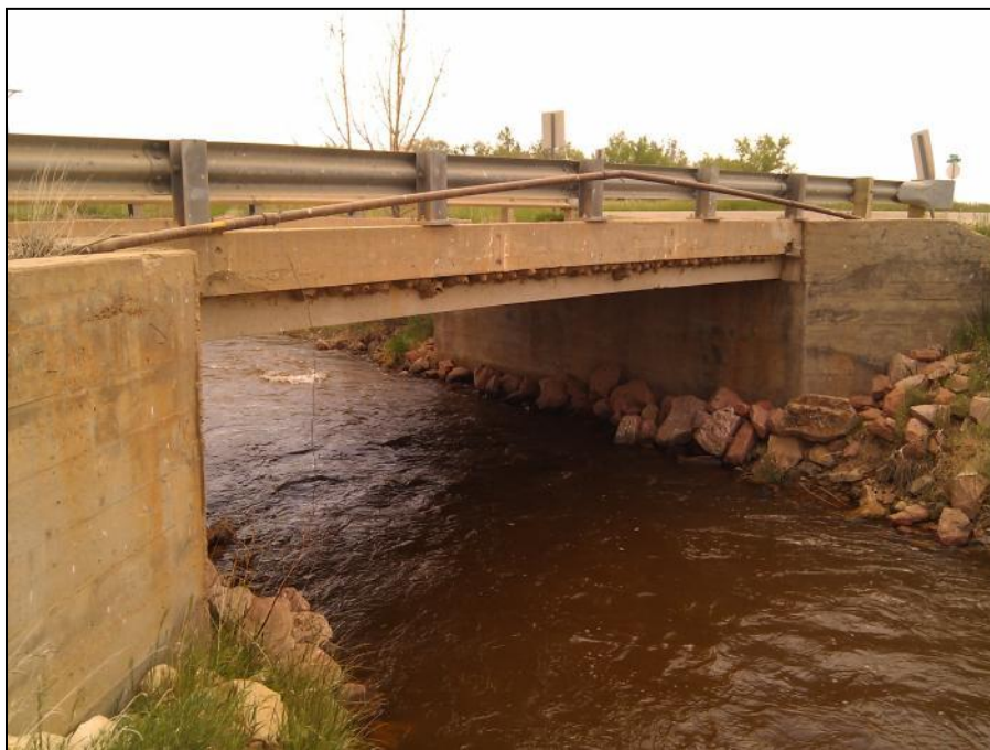
Figure E.6 Bridge 2
