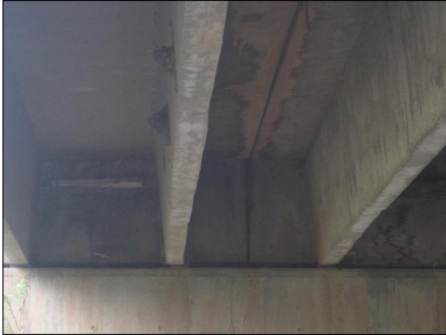
Figure E.54 Bridge 16 Supports
