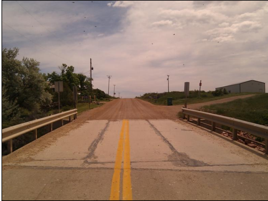
Figure E.46 Bridge 14 Deck
