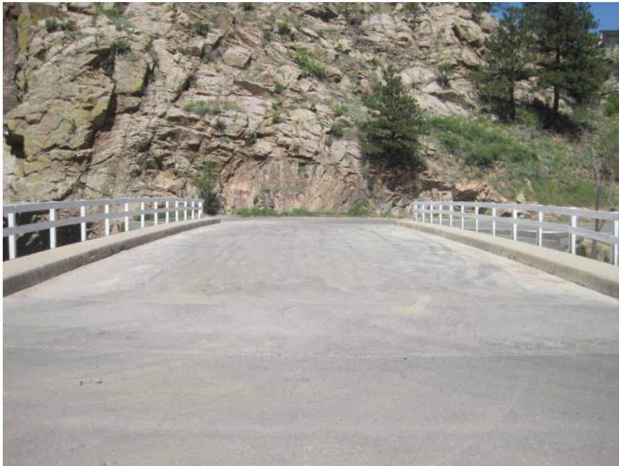
Figure E.20 Deck of Bridge 8
