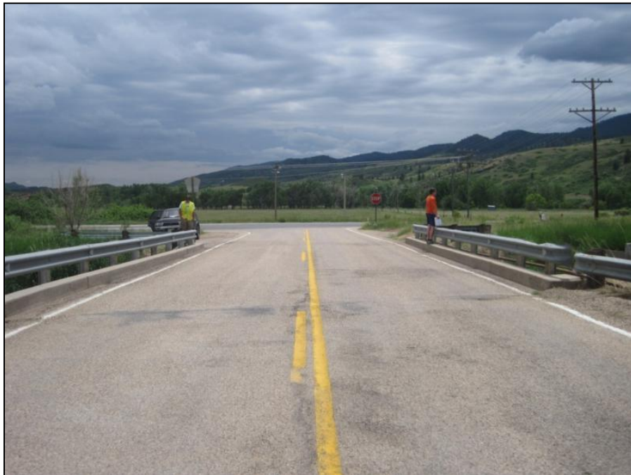
Figure E.26 Deck of Bridge 9
