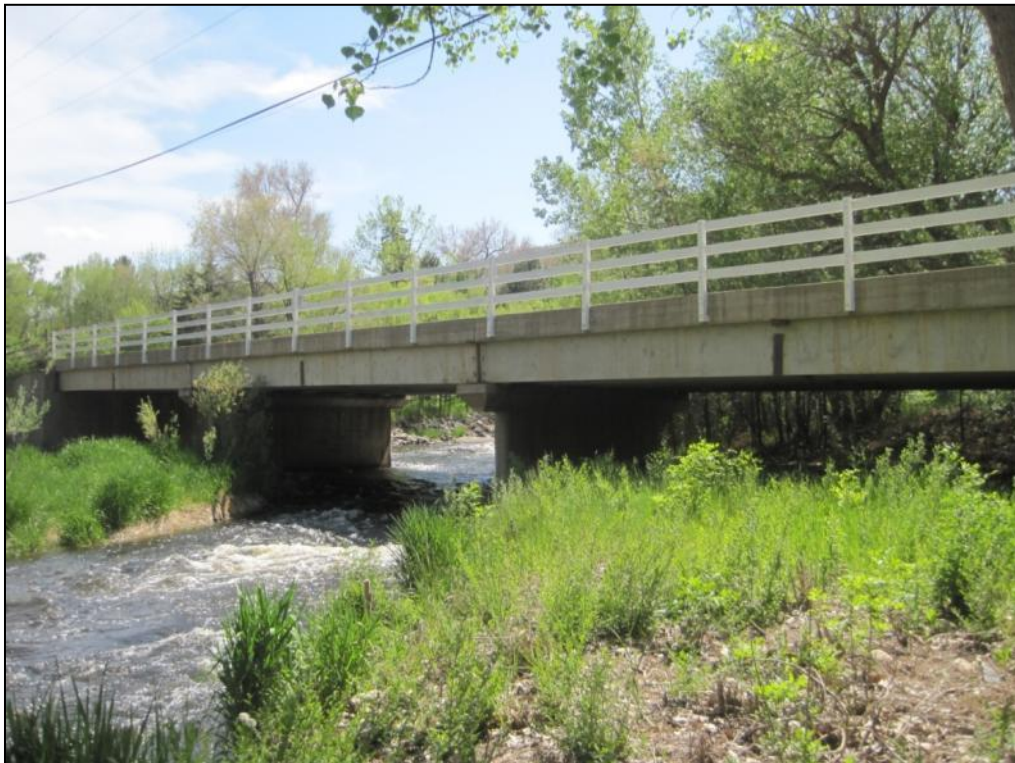
Figure E.33 Bridge 10 - Three spans
