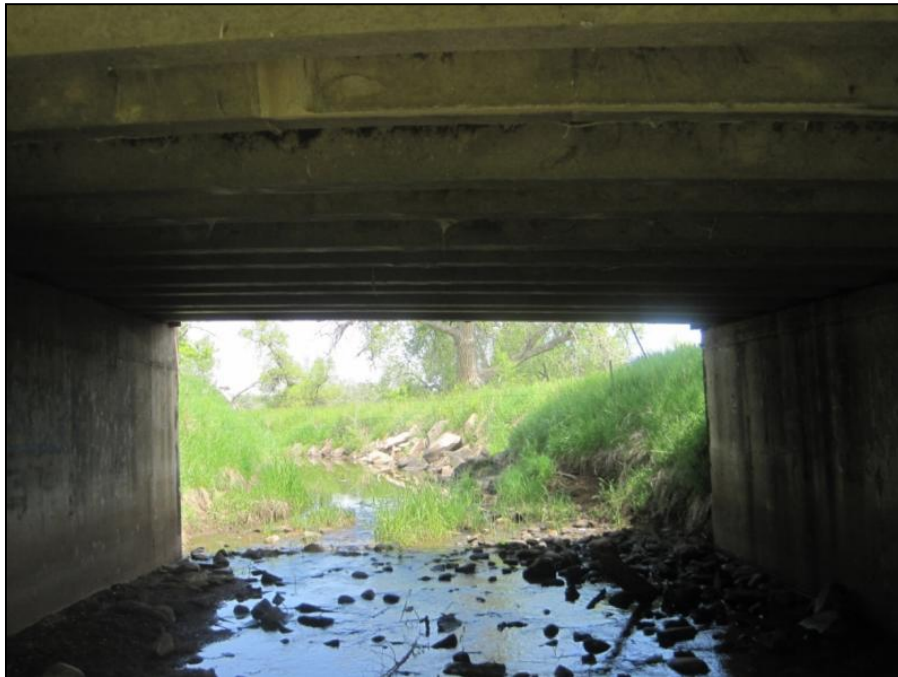
Figure E.41 Bridge 12 Streambed
