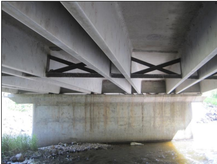
Figure E.35 Bridge 10 Pier
