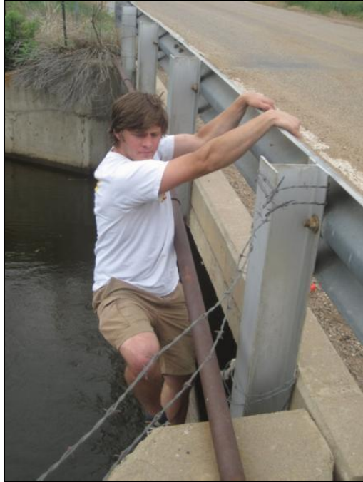
Figure E.13 Difficult access to underside of Bridge 5
