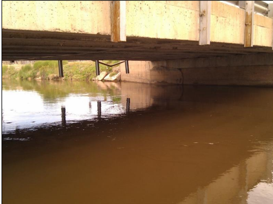
Figure E.37 Bridge 11 Span
