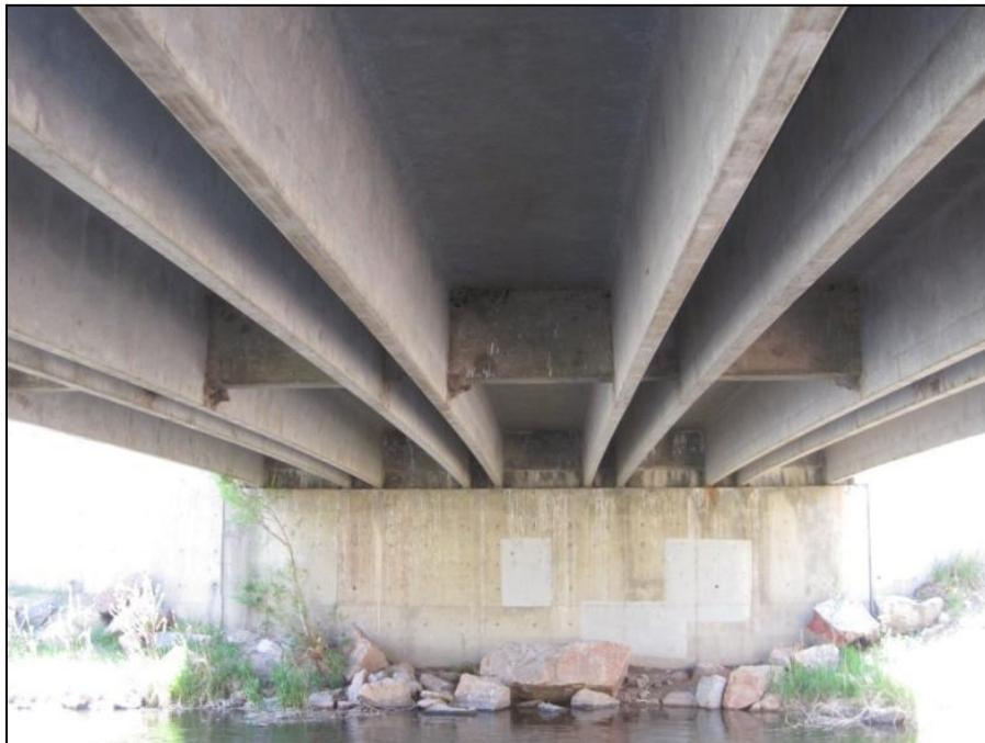
Figure E.24 Bridge 8 - Double T- girders and diaphragms
