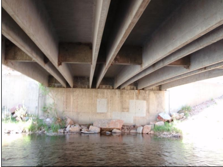
Figure E.23 Bridge 8 - Double T- girders and diaphragms
