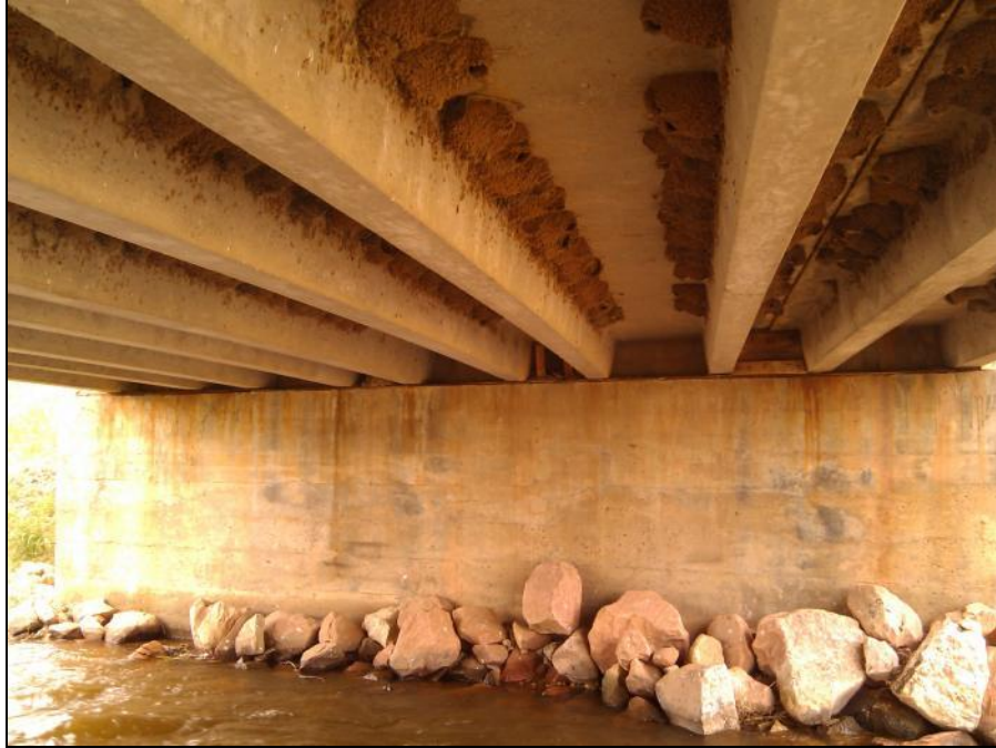
Figure E.5 Bridge 2 - Double T-beams
