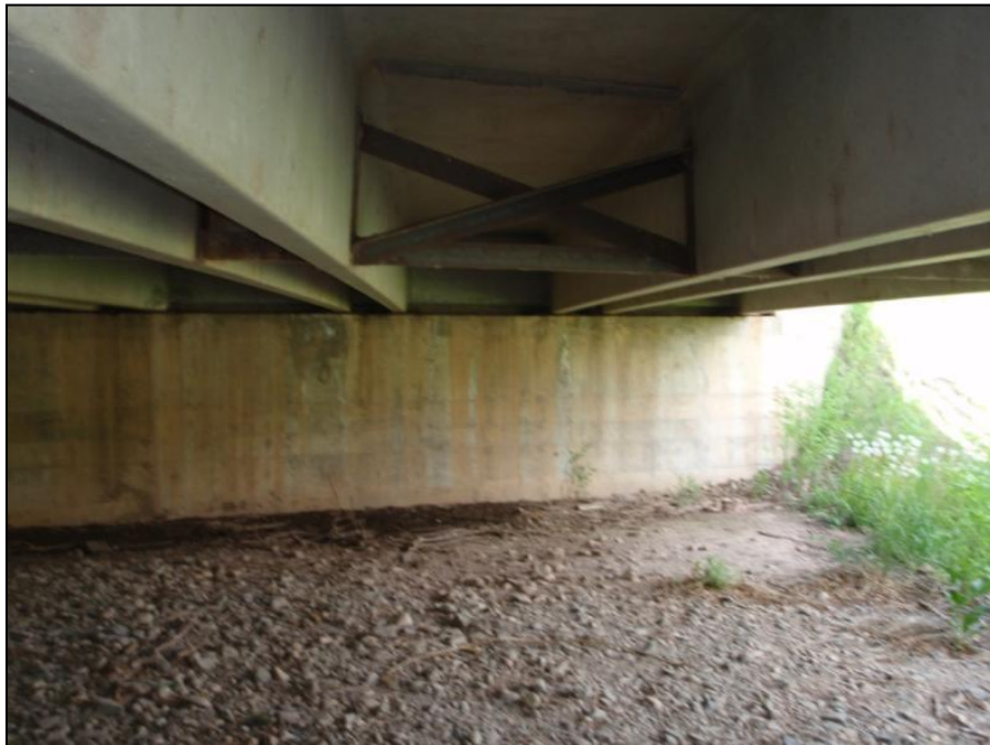
Figure E.31 Diaphragm and double T-girder of Bridge 10
