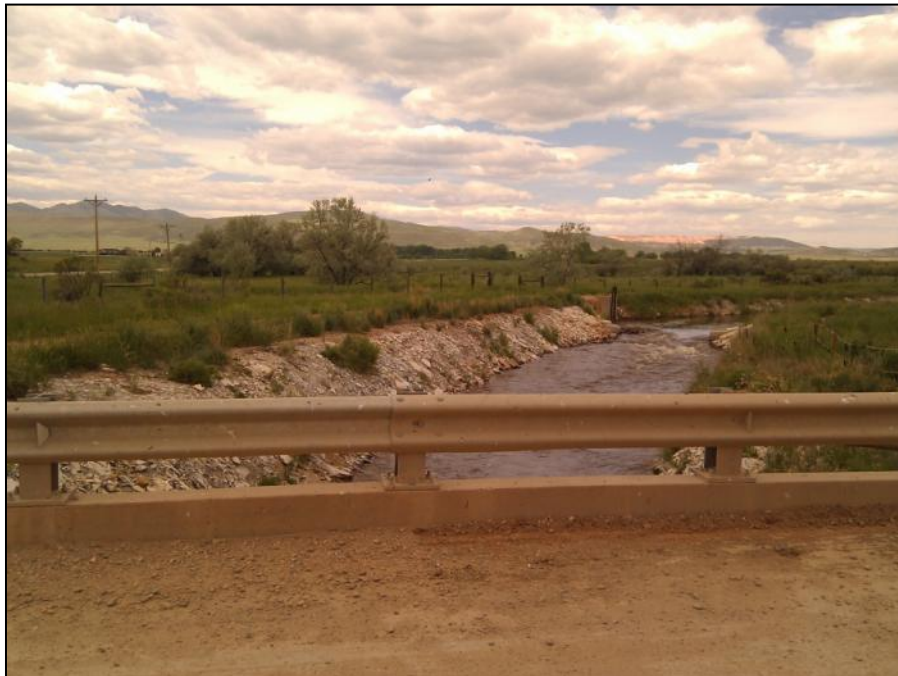
Figure E.4 Bridge 2 - Railing and streambed
