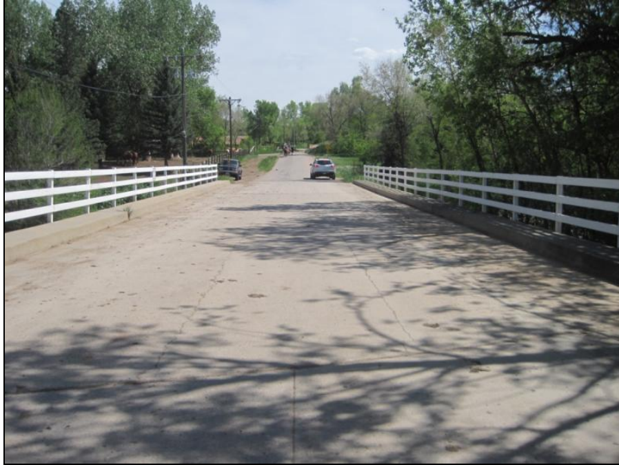
Figure E.32 Deck of Bridge 10
