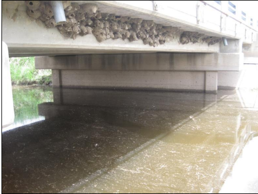
Figure E.27 Bridge 9
