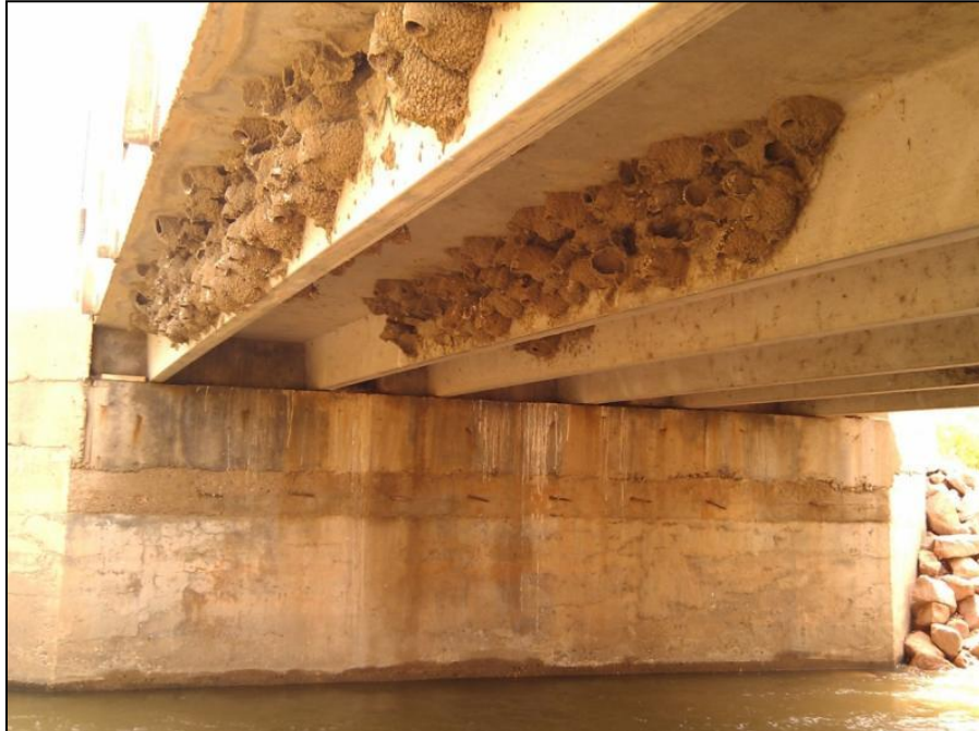
Figure E.45 Bridge 14 Double T-girders
