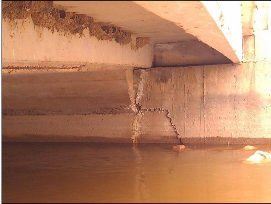
Figure E.50 Bridge 15 - Double T- girder and slab
