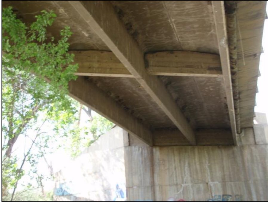
Figure E.3 Bridge 1 T-girders and diaphragm
