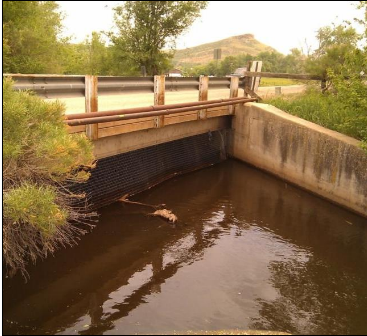
Figure E.44 Bridge 13 Downstream Screen
