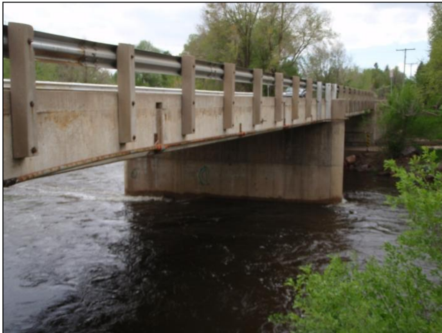
Figure E.8 Bridge 3 - span
