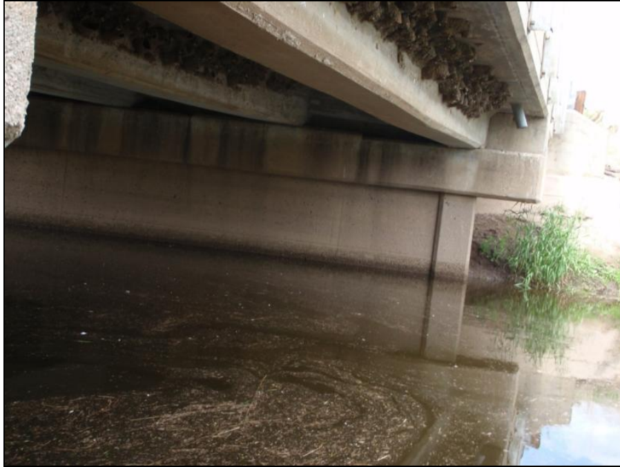
Figure E.30 Underside of Bridge 9
