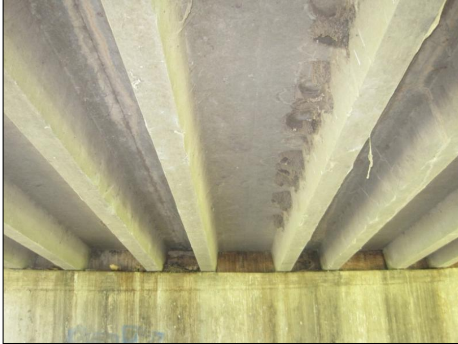
Figure E.42 Bridge 12 Double T-girders
