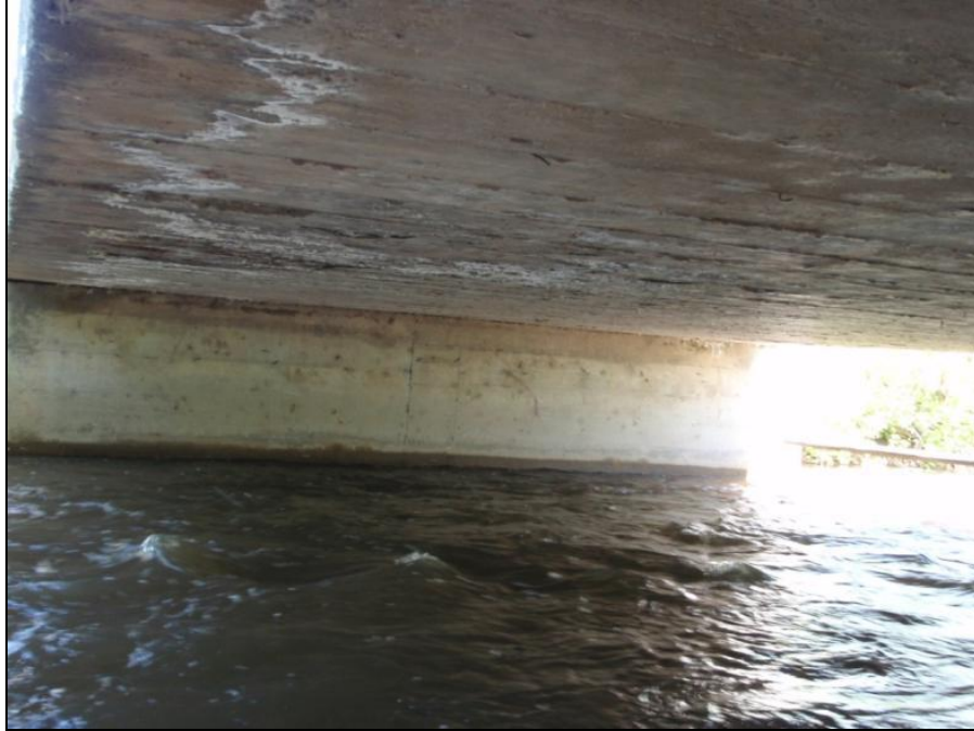
Figure E.19 Bridge 7 - Underside of concrete slab
