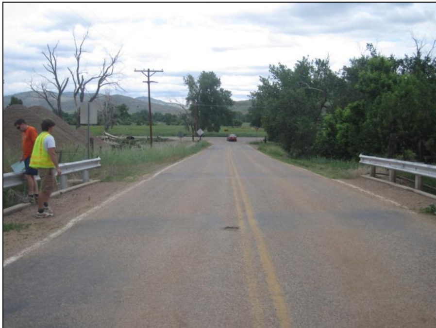
Figure E.12 Deck of Bridge 5
