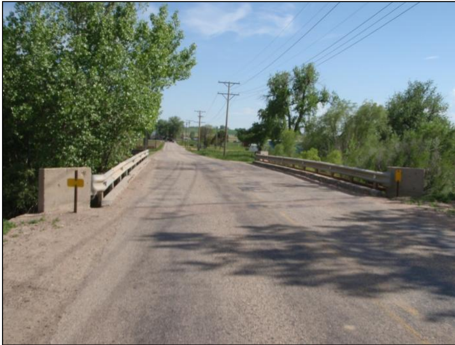
Figure E.1 Bridge 1 Looking South
