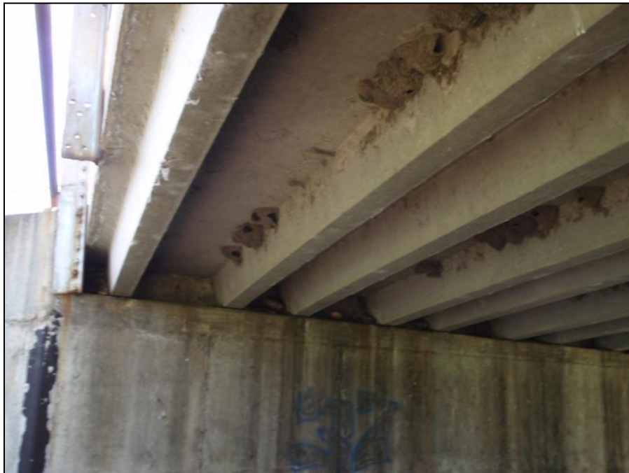
Figure E.39 Bridge 12 Double T-girders
