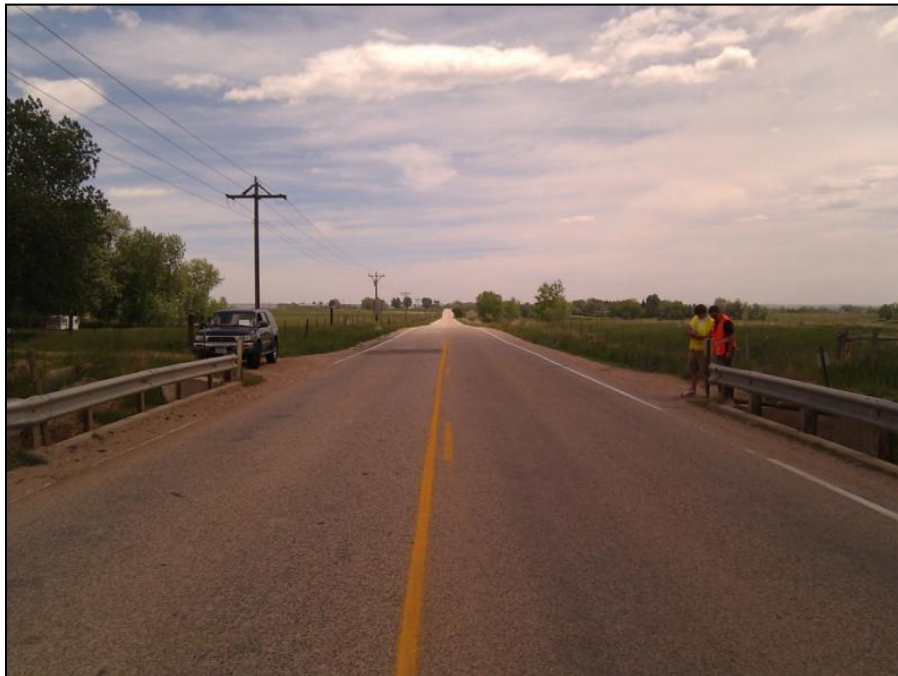
Figure E.49 Bridge 15 Deck
