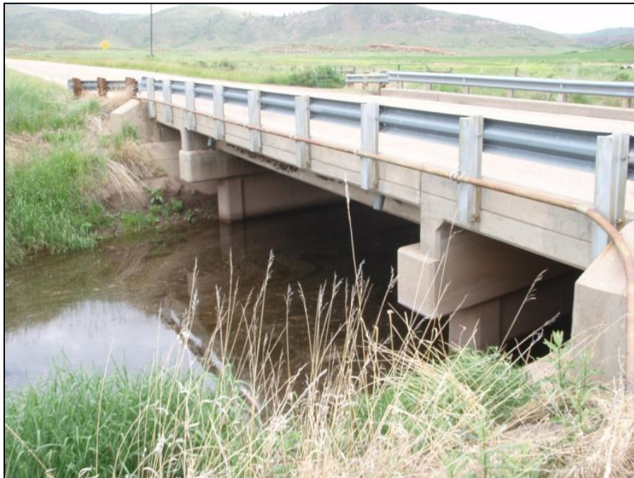
Figure E.28 Bridge 9 - span
