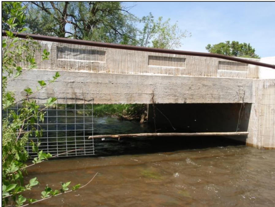
Figure E.18 Bridge 7 - Concrete slab
