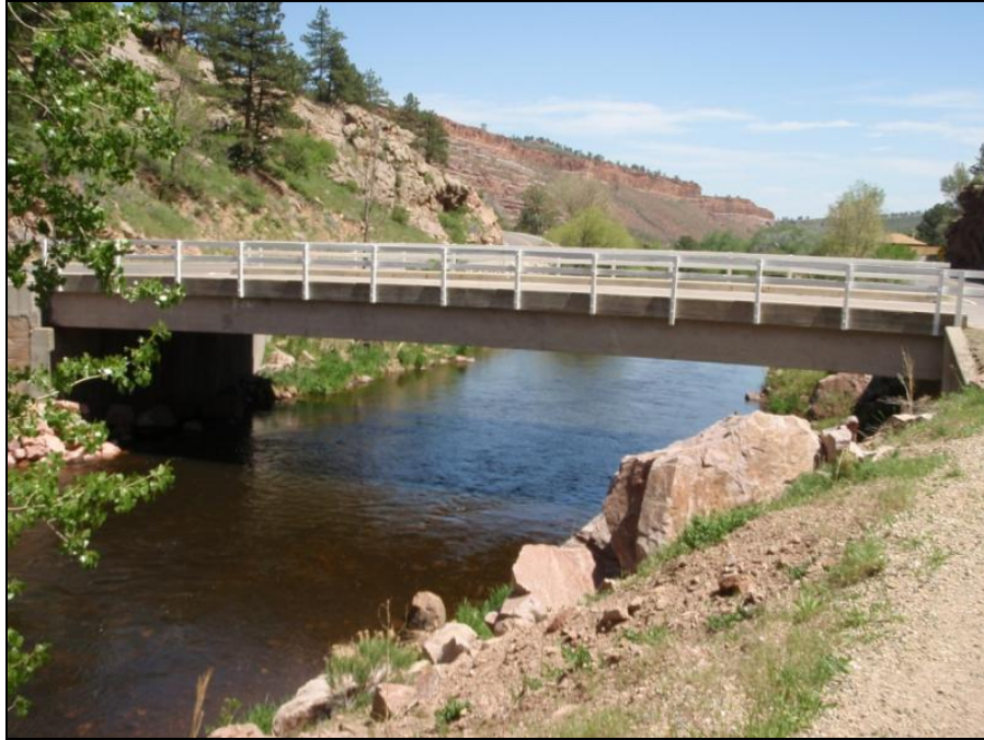
Figure E.21 Bridge 8 - Span
