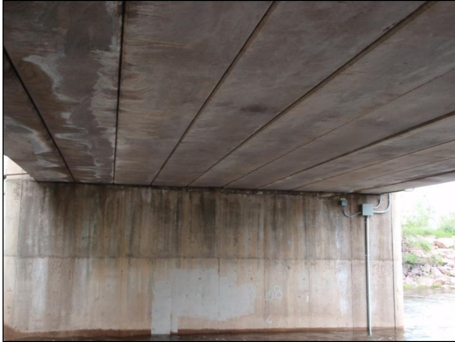
Figure E.9 Bridge 3 - Underside of prestressed box girders
