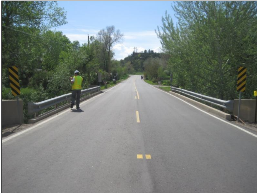
Figure E.10 Deck of Bridge 4
