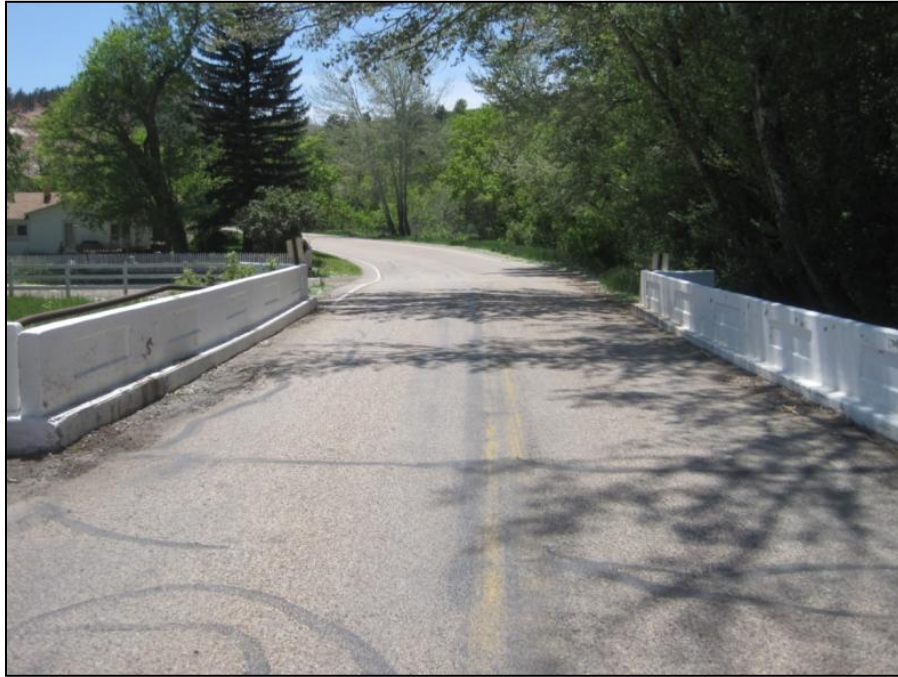
Figure E.17 Deck of Bridge 7
