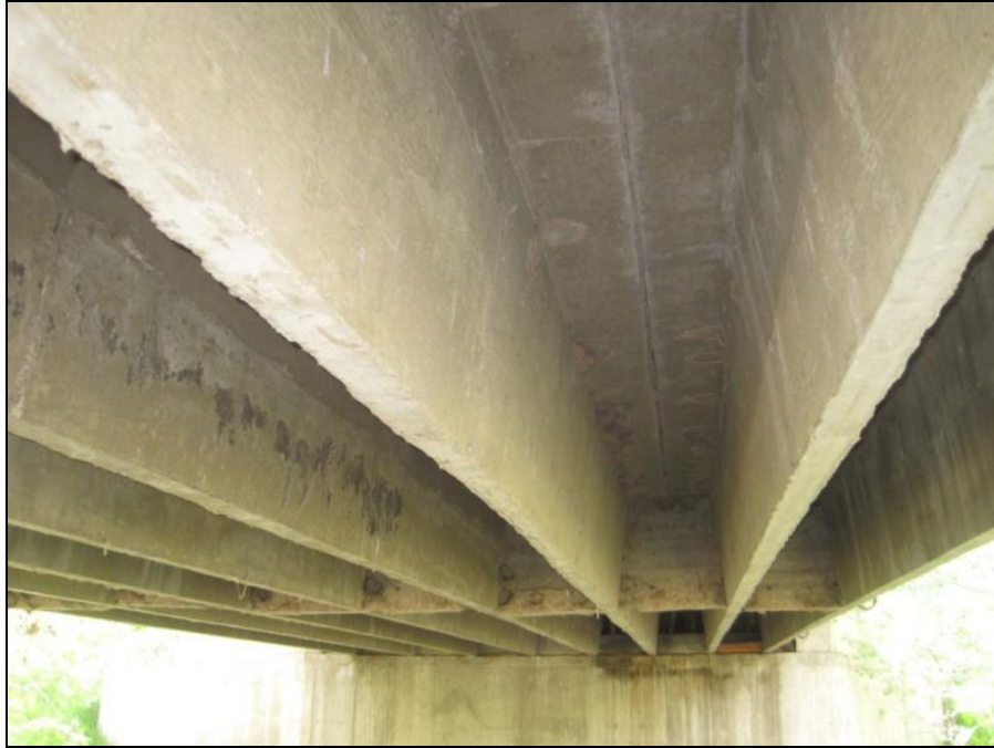
Figure E.11 Bridge 4 - Double T-beams
