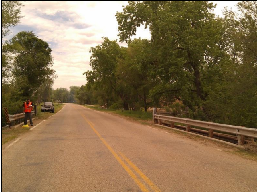
Figure E.43 Bridge 13 Deck
