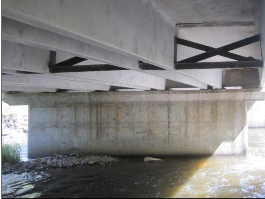
Figure E.34 Bridge 10 Double T- Girders
