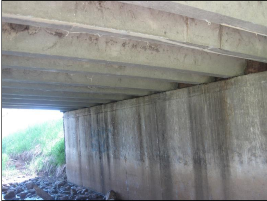
Figure E.15 Bridge 6 - Double T- Beams
