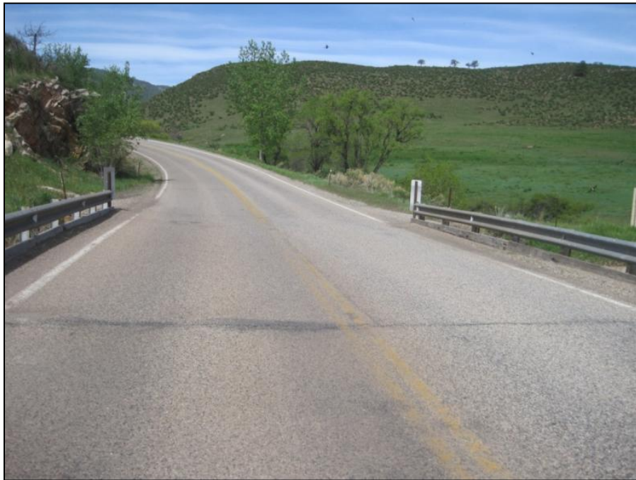
Figure E.14 Deck of Bridge 6
