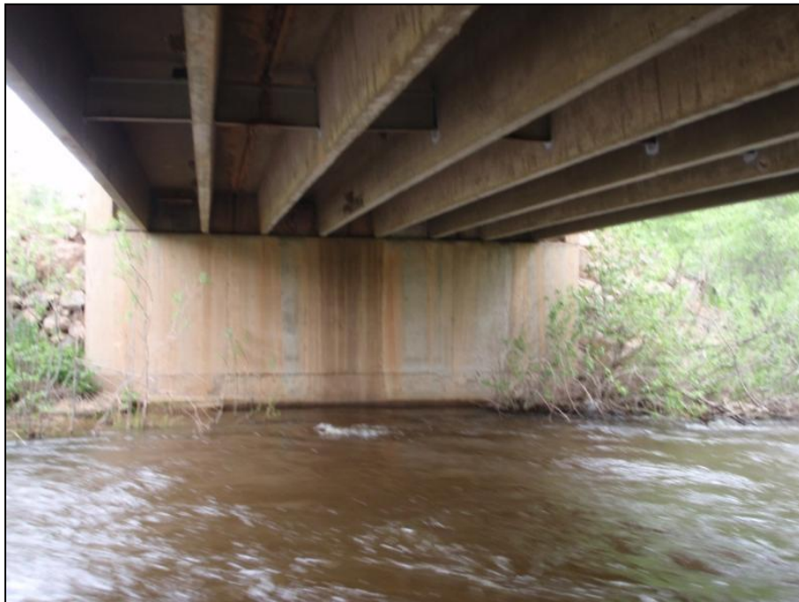
Figure E.57 Bridge 16 - Wing wall and Girders
