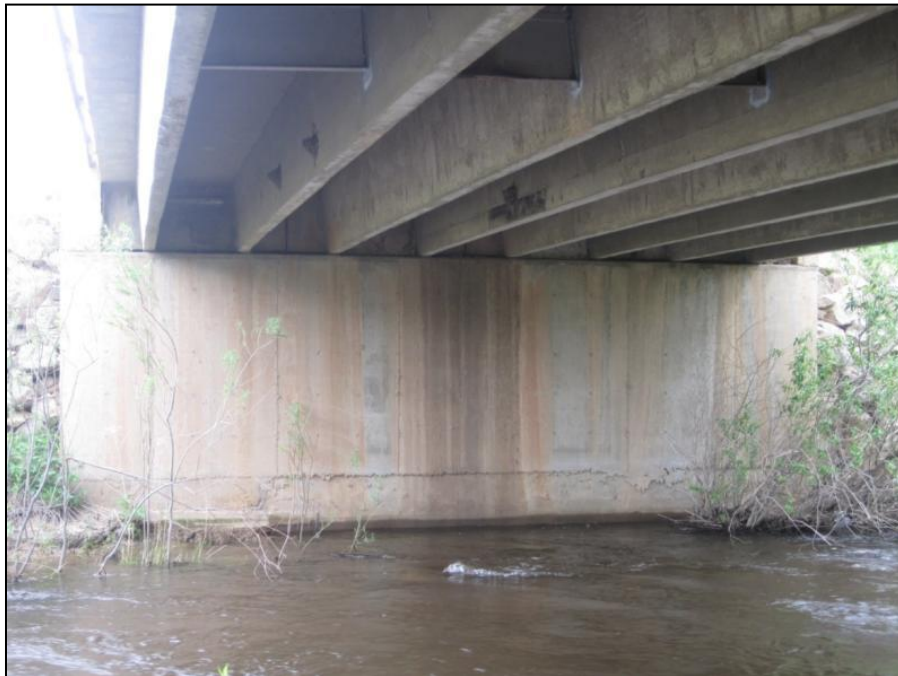
Figure E.53 Bridge 16 Double T- girders and diaphragm
