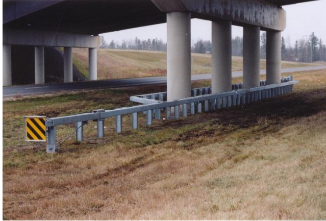
Figure 1.1 Box beak longitudinal barrier (AASHTO 2004)
