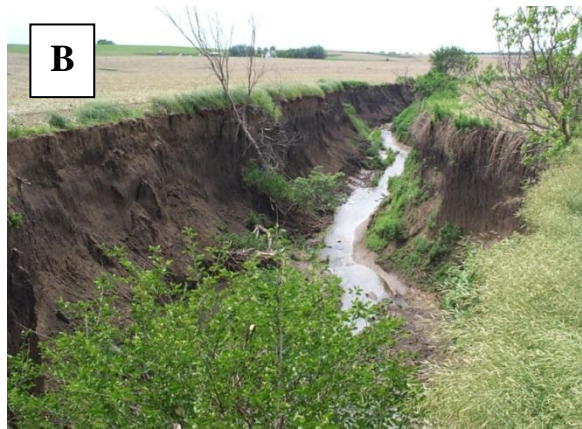
Figure 1.1 (b) Channel incision at Mud Creek
