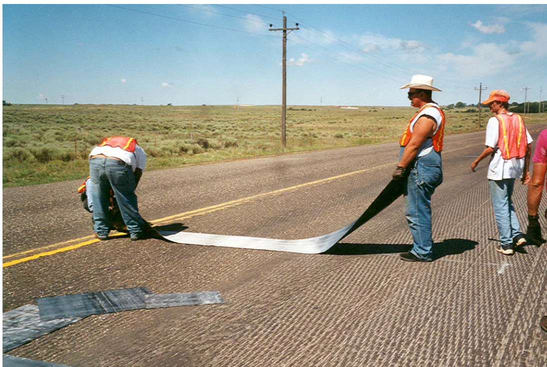
FIGURE 16 Installation of precoated fabric membrane strip.
