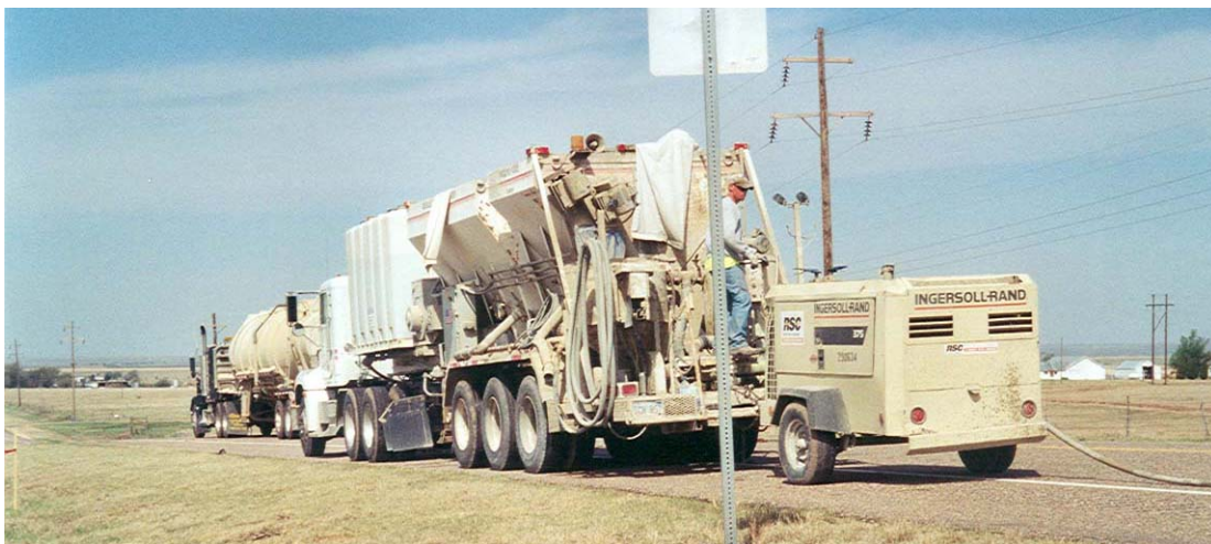
FIGURE 8 Slurry injection equipment.
