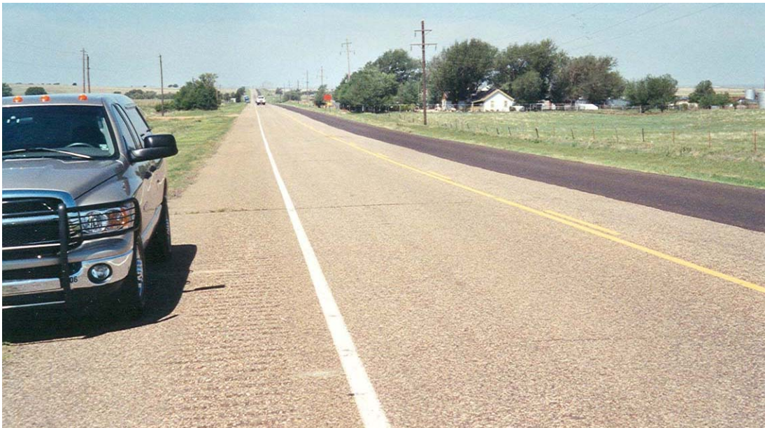
FIGURE 6 US 412 prior to CIR rehabilitation.
