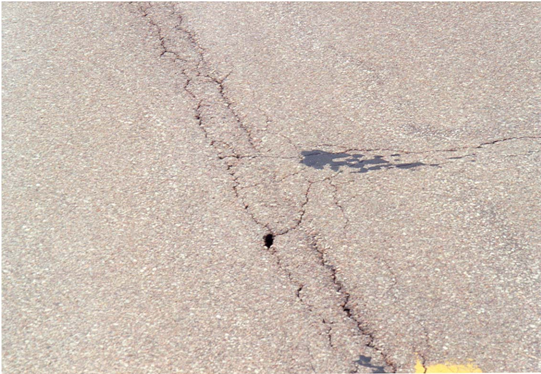
FIGURE 14 Typical distress on US-412 Harper, County.
