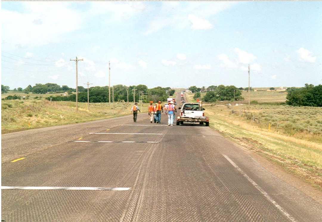
Figure 19 Installation of precoated fabric membrane strips.
