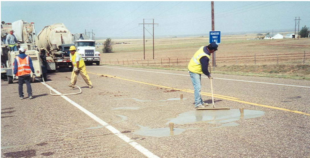
FIGURE 7 Fly ash slurry crack injection on US 412.
