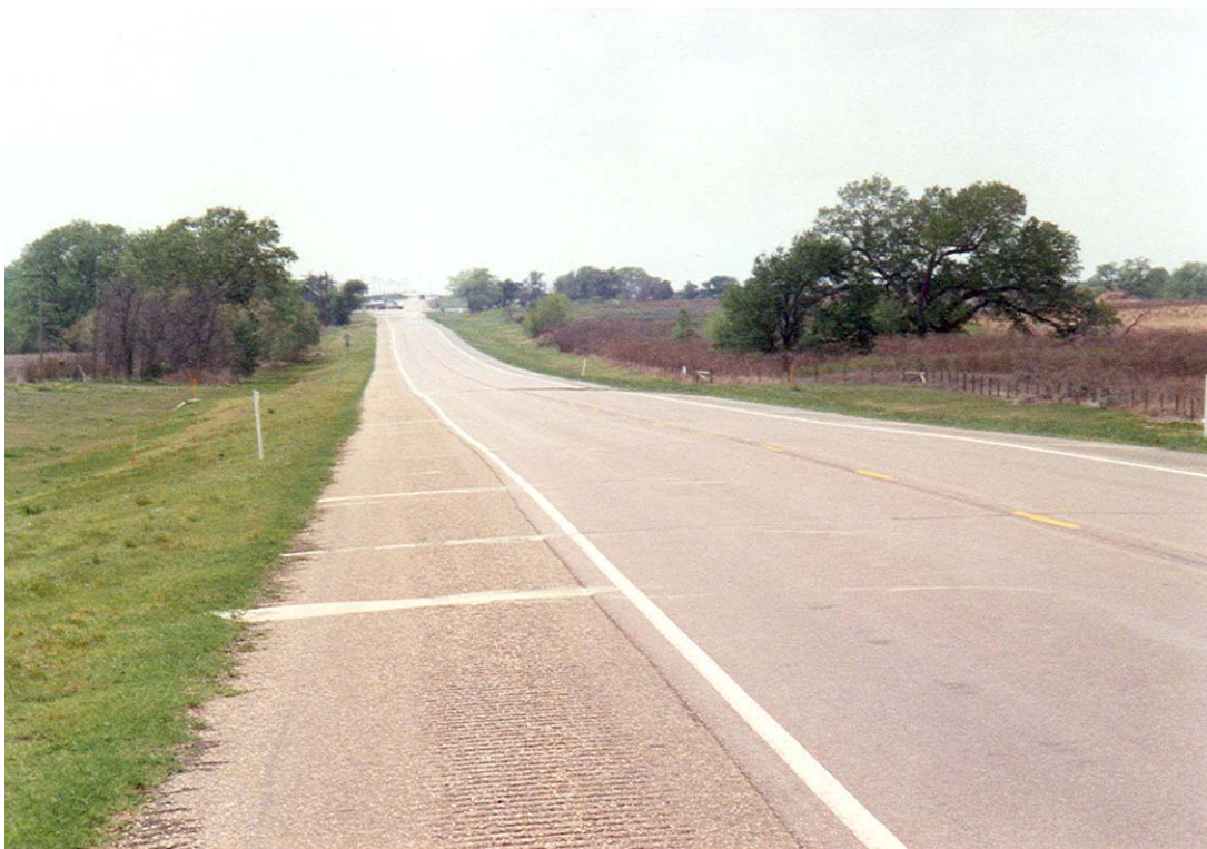
FIGURE 15 US 412 Harper, County after slurry crack injection.
