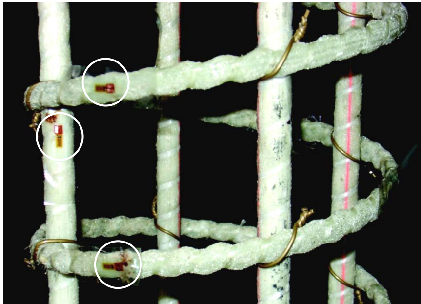
Figure 2.12: Internal strain gauge placement
