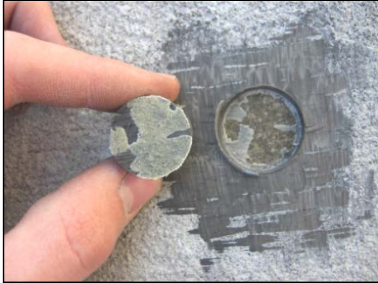
Figure 4.22: Original concrete region bond test
