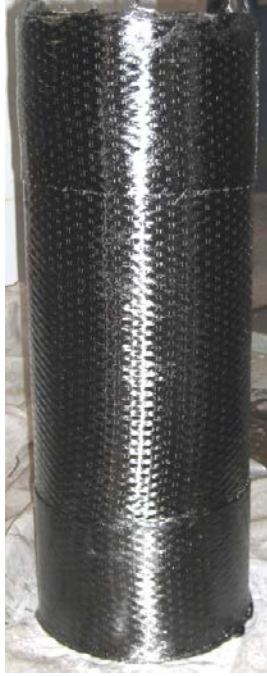
Figure 2.10: CFRP wrapped column
