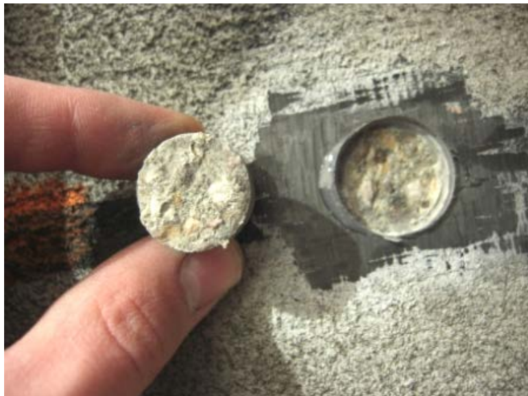
Figure 4.21: Grout region bond test
